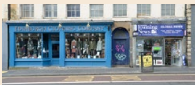
South Bridge shop front restored by EWH grant funding (© EWH)
