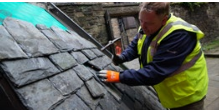
Roofing demonstration at the launch of the ‘Guide to Building Maintenance in a Changing Climate’ at Acheson House
