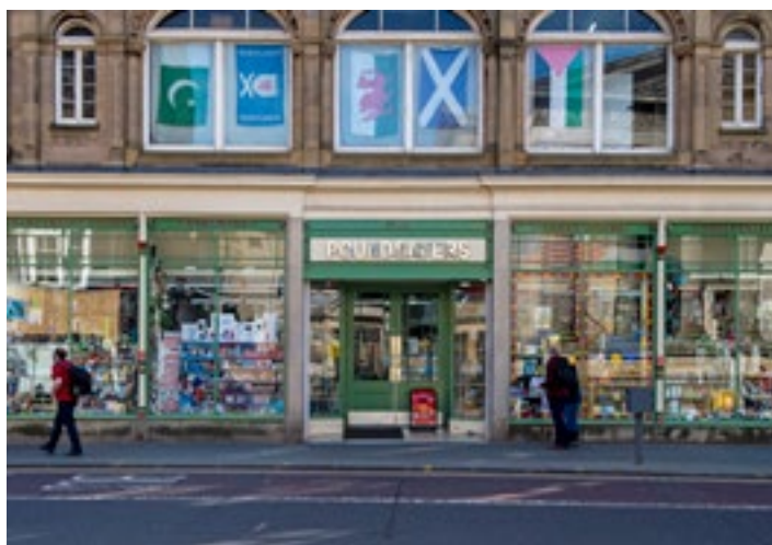
A successful shop front restoration on Nicolson Street (© Neil Hanna)
