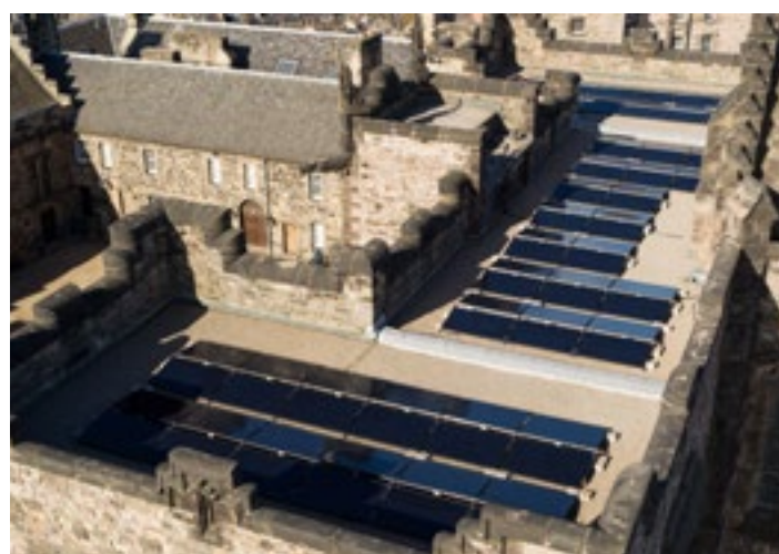
Solar panels concealed behind raised parapets
