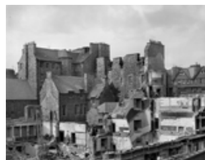
Jamaica Street, Edinburgh just prior to demolition
