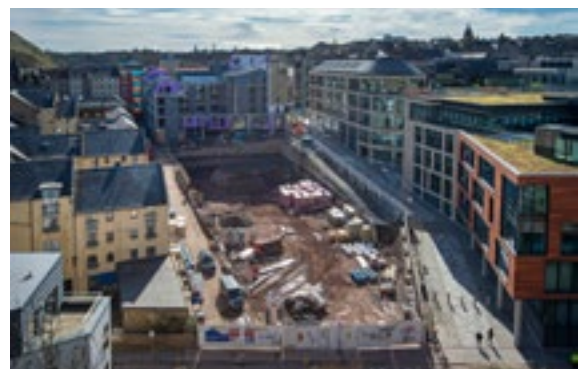
Development under construction at New Street (© Neil Hanna)
