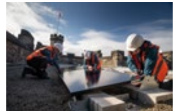
Solar panel installation
