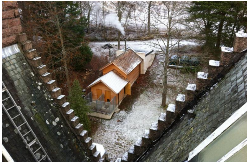
Fig: 2 Double dog kennel and new boiler house. Photo taken from roof of castle.
