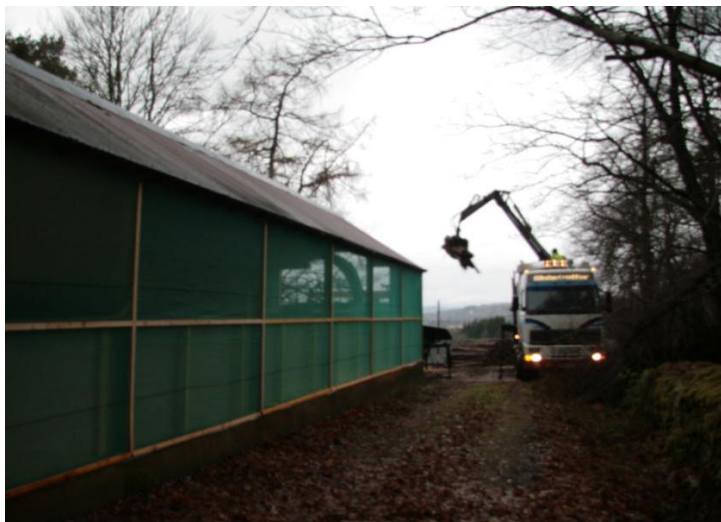
Fig 7: Wood chip store in a renovated silage pit, note the mesh walls for ventilation
