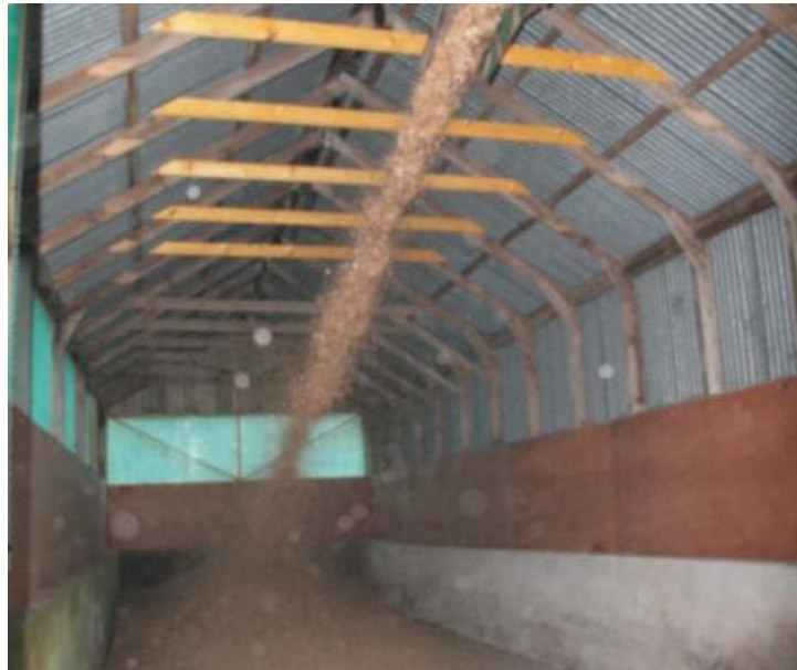
Fig 6: Wood chip propelled to the rear of the wood chip store
