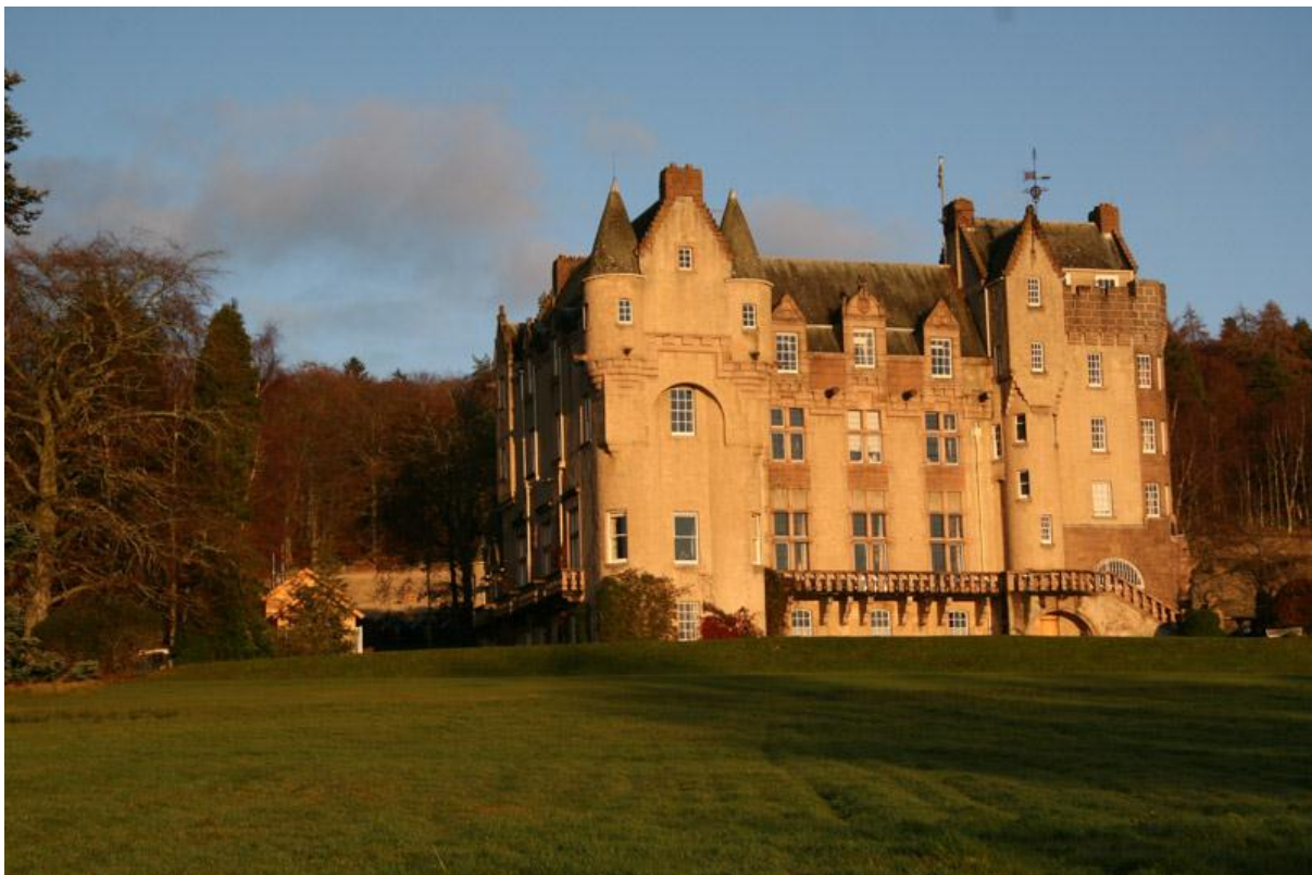
Fig 11: Kincardine Castle. The Boiler House can be seen discretely located behind the holly tree to the left.
