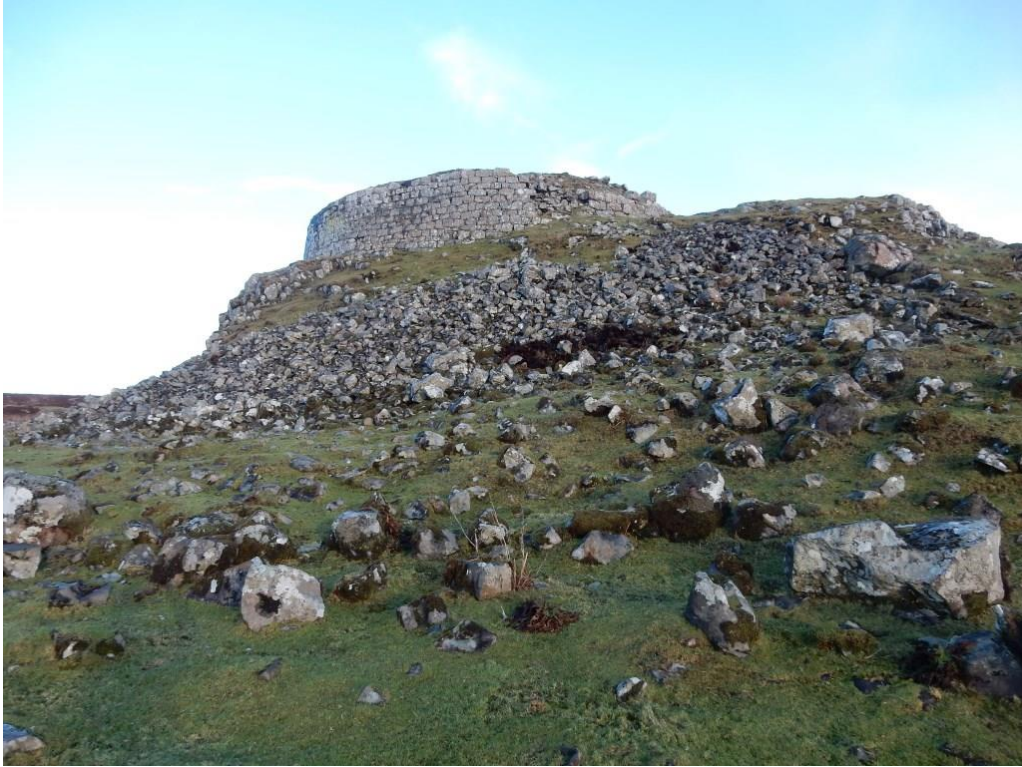
Dun Beag, south-west sector, showing collapsed masonry
