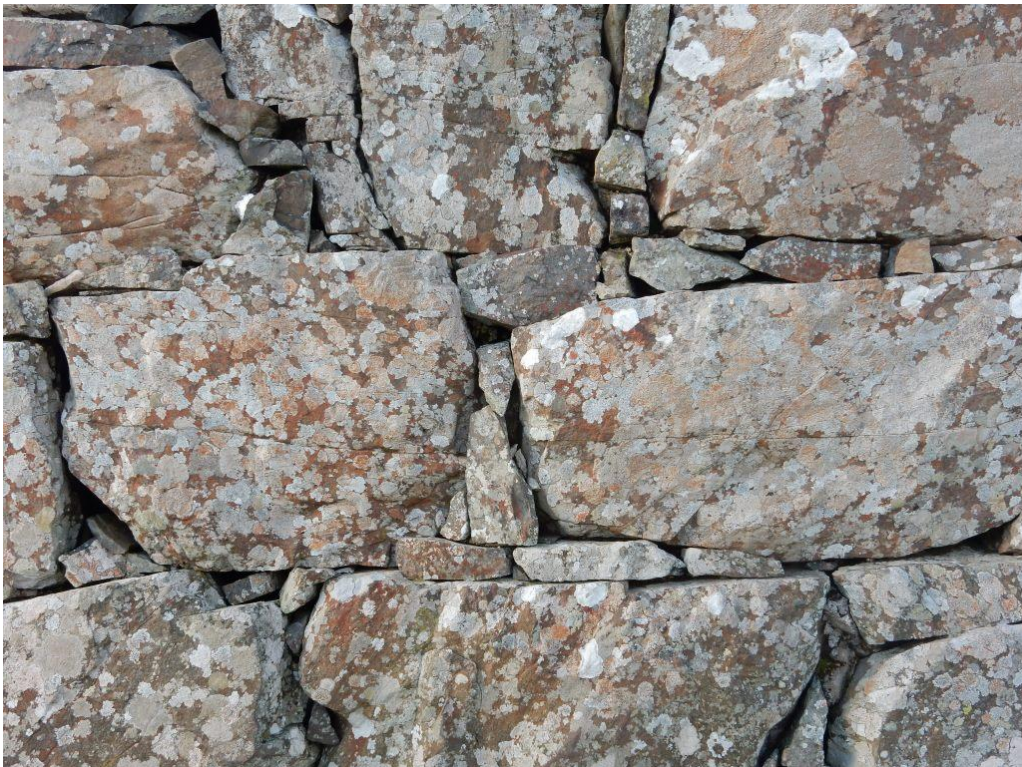
Dun Beag, detail of wall showing pinnings
