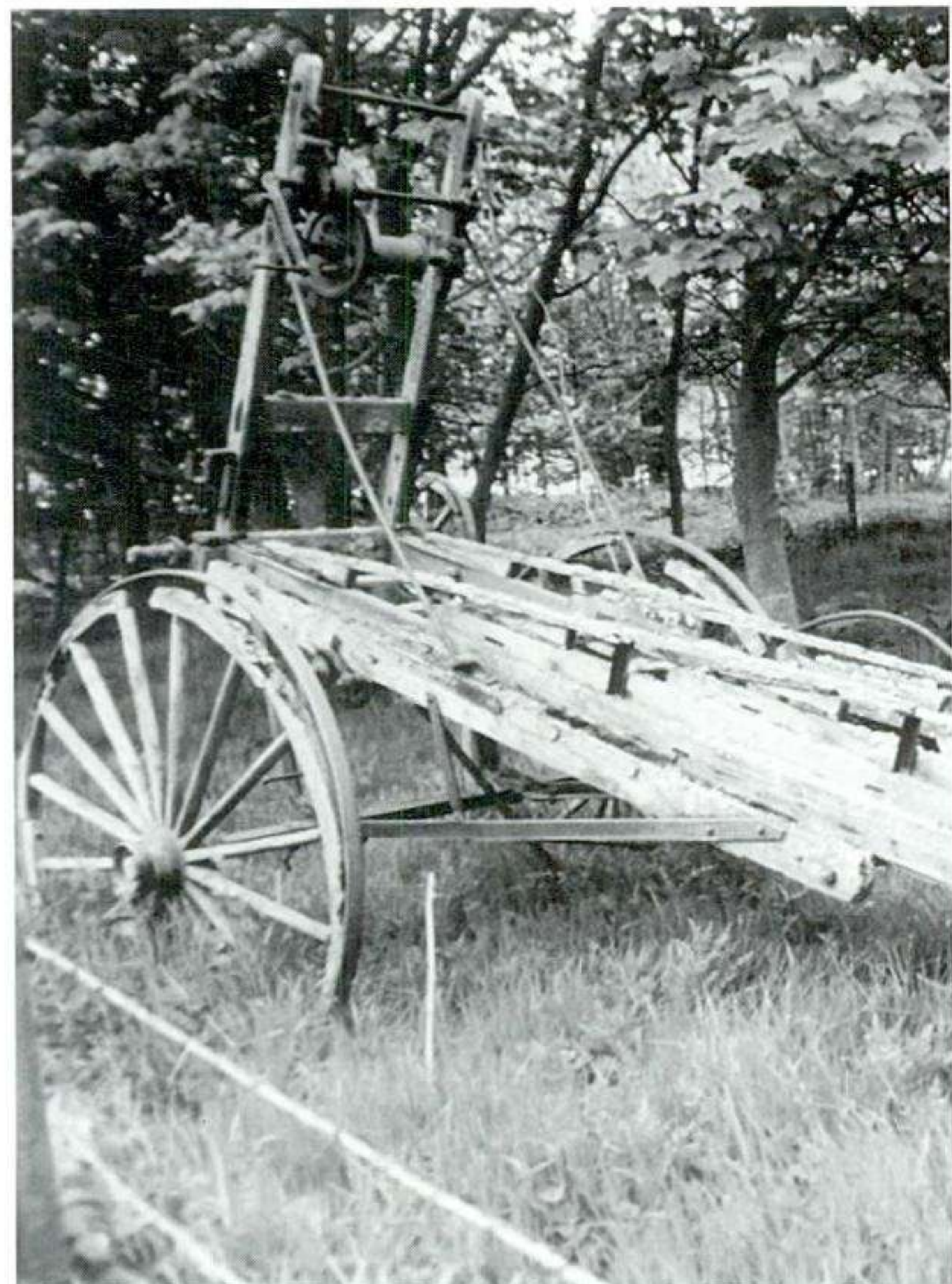
Fig. 5 Escape ladders. Displaying the skills of estate craftsmen in metal and wood, this extending escape ladder was easily transported around on its two cart wheels. A ratchet device on the winding drum prevented the ladder from accidentally retracting whilst in use.
