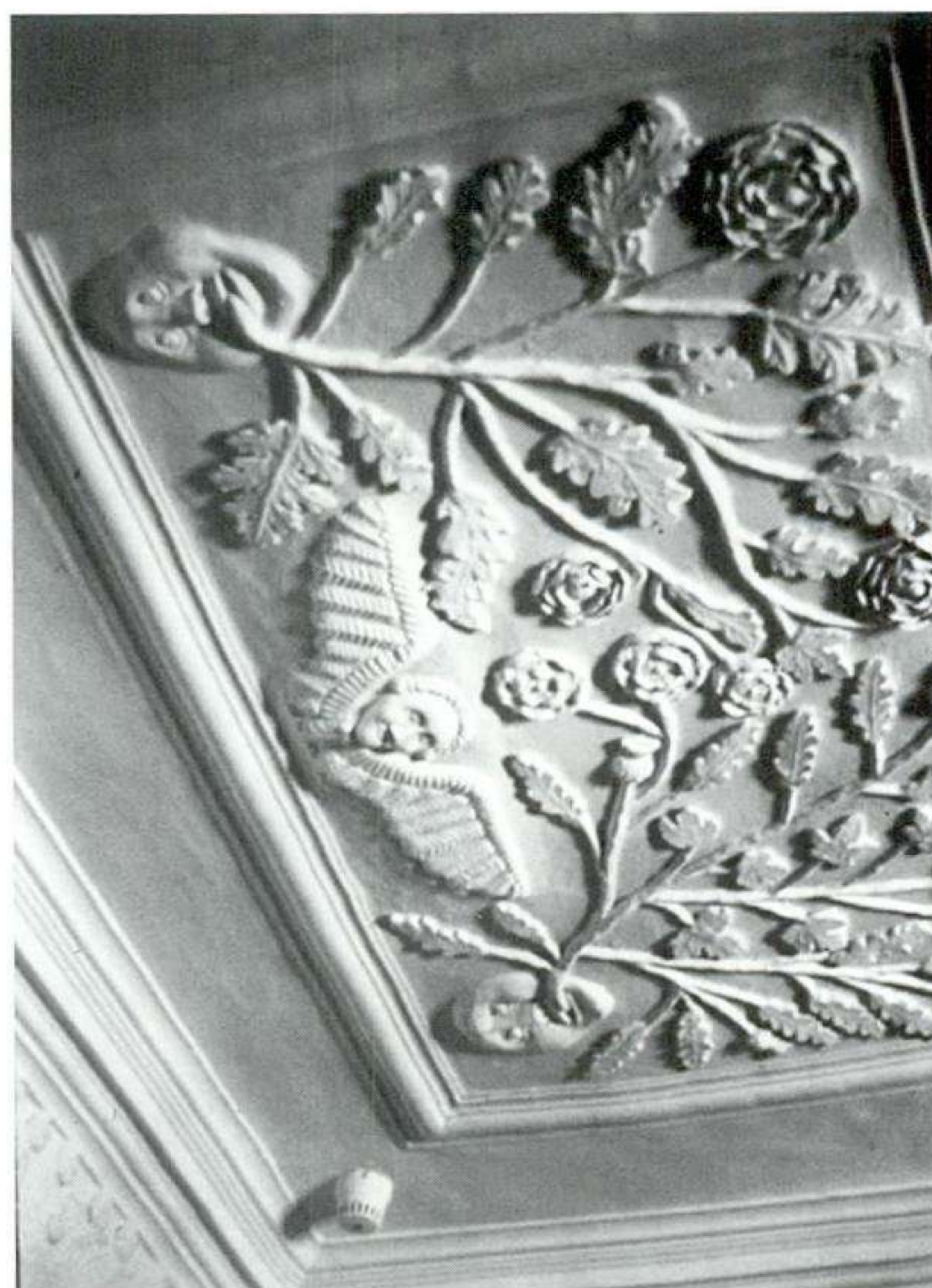
Fig. 12 Detection equipment. With a limited choice of sympathetically designed equipment being available to the specifier, it can be difficult to be sensitive in the appropriate positioning of smoke detector heads. Due to their size and required operating parameters, in certain situations it may be more relevant to install an air sampling system.
