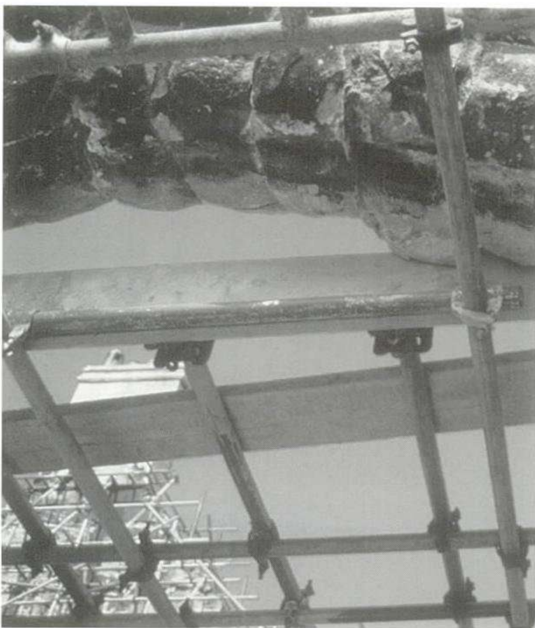
Fig. 2 Temporary support in place at Mar Lodge after the fire
