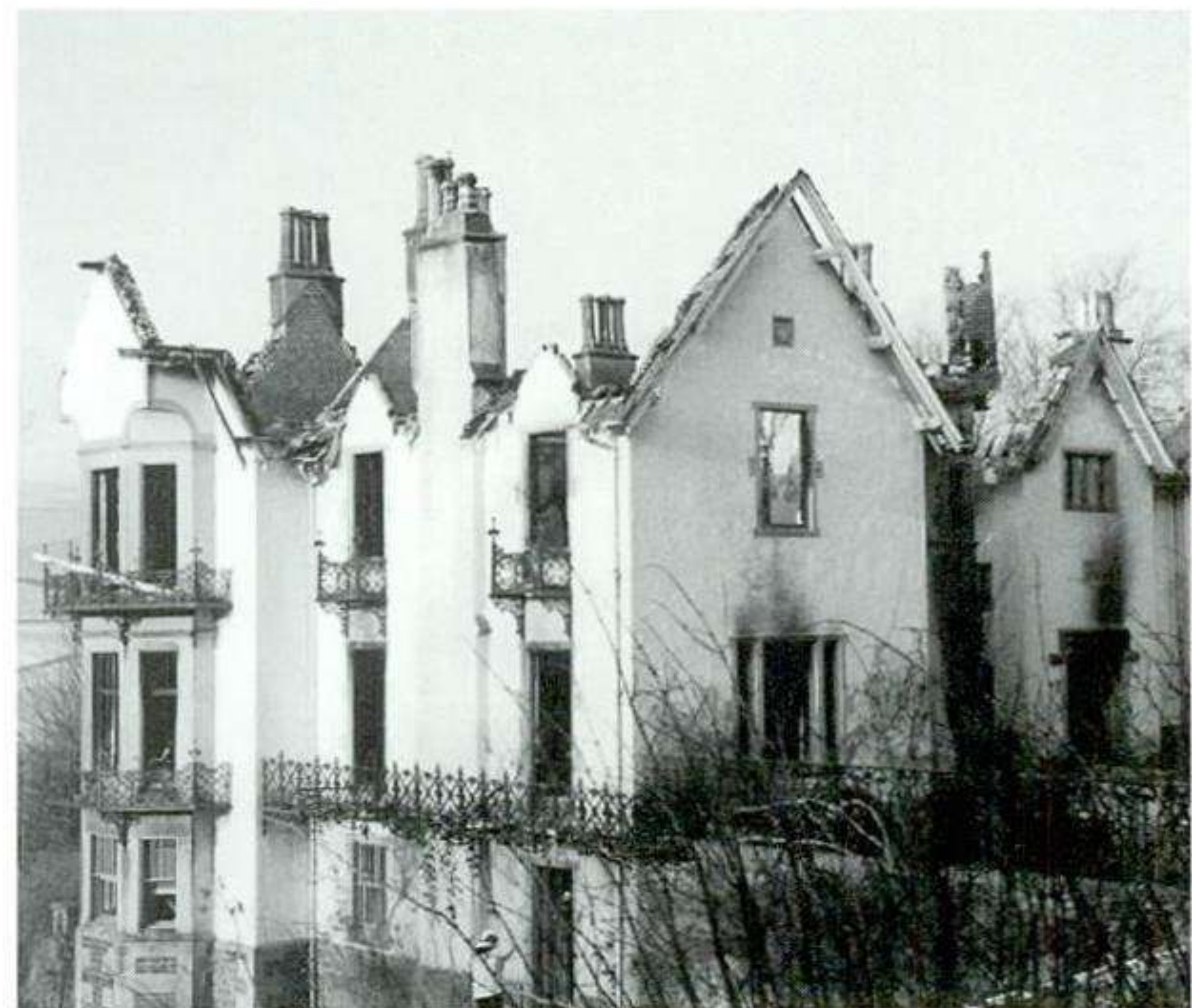
Fig. 10 Torsonce House, Stow, Roxburghshire
