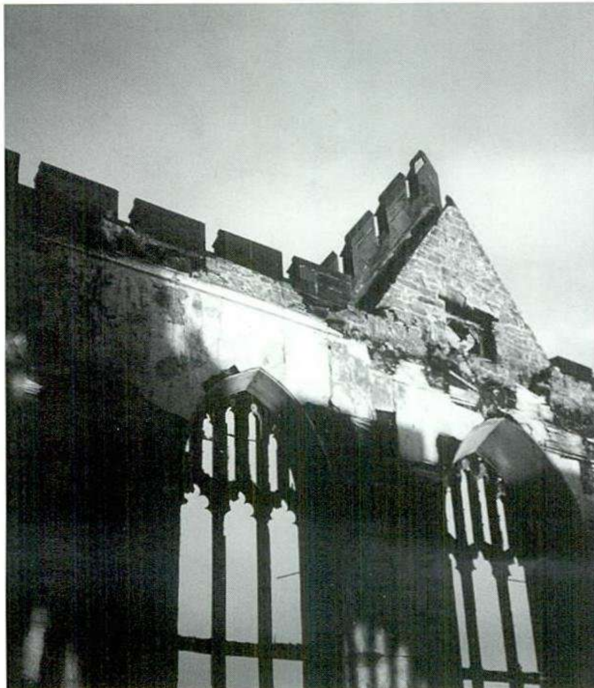
Fig. 1 Dunbar Parish Church after a fire in 1987 which destroyed the interior and roof.
