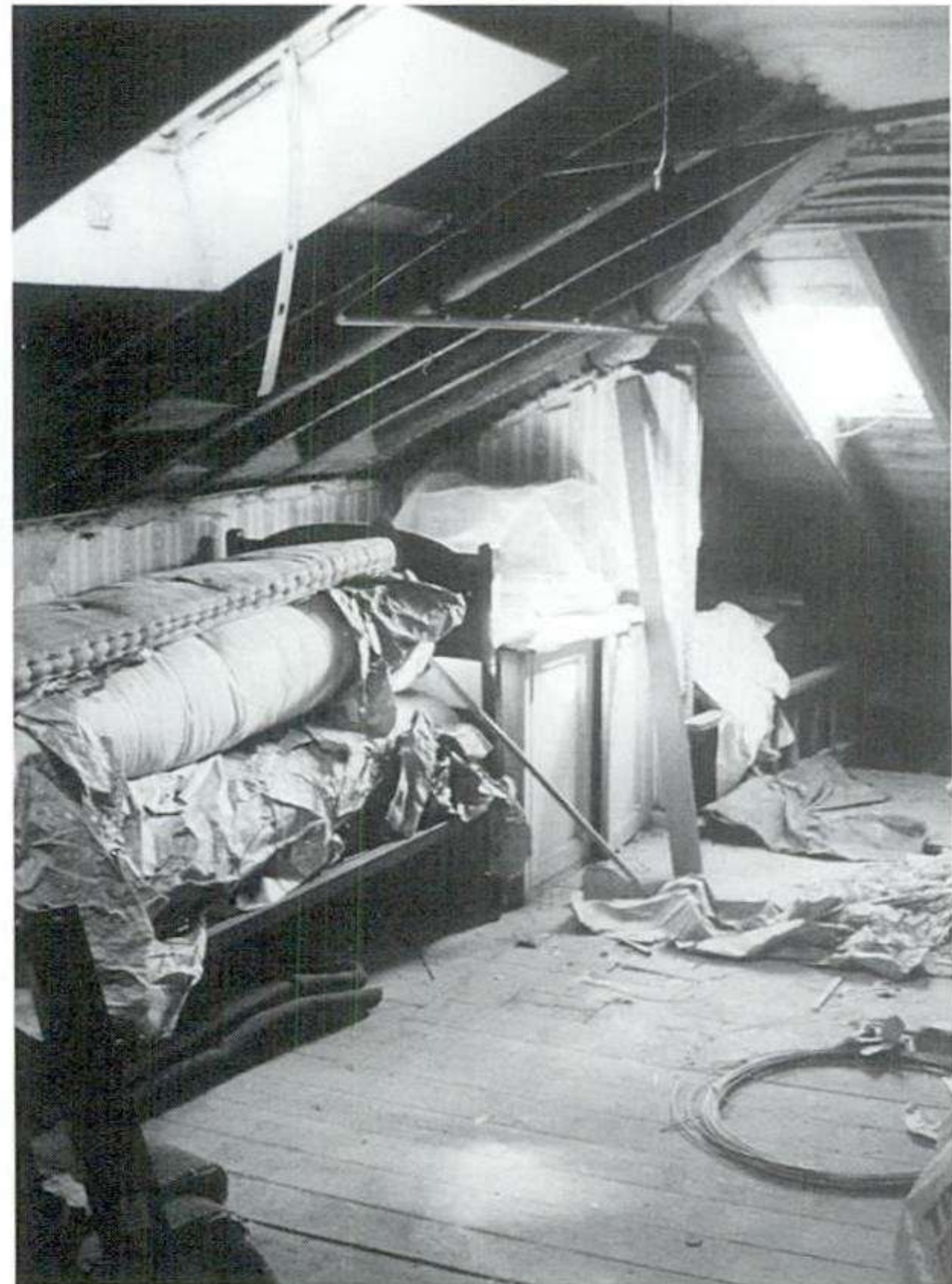
Fig. 17 Additional fire risks. Fires need ignition, oxygen and fuel to gain hold. Through effective management and training much can be done, without additional cost, to reduce the risks involved. Human nature tends to hoard material things, and if storage space is available, it will be filled with items - valuable or not. Attic spaces are particularly vulnerable to this phenomenon. They should be regularly inspected and any unwanted or high risk items removed, especially if they contribute to an increased fire load.
