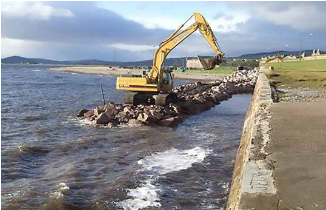
Figure 21: An area of protective 'rock armour' has been built in front of the walls to reduce the destructive force of the waves.
