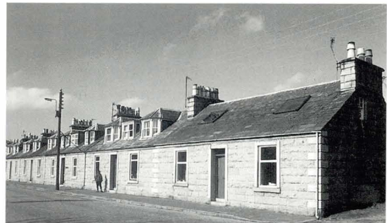
Plate 4 Cleaned granite in Dalbeattie. Buildings cleaned circa 1970.
