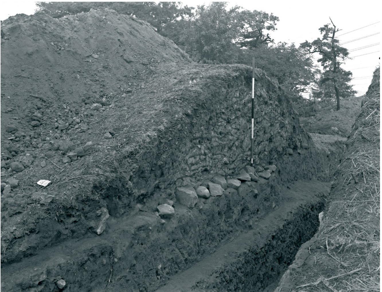
Figure 3.1 Professor Anne Robertson's section through the Antonine Wall at Tentfield Plantation, east of Rough Castle, in 1959, reveals many layers of turf work erected on a stone base. This provides valuable information on the nature of the vegetation at the time the Romans started to build the Wall
