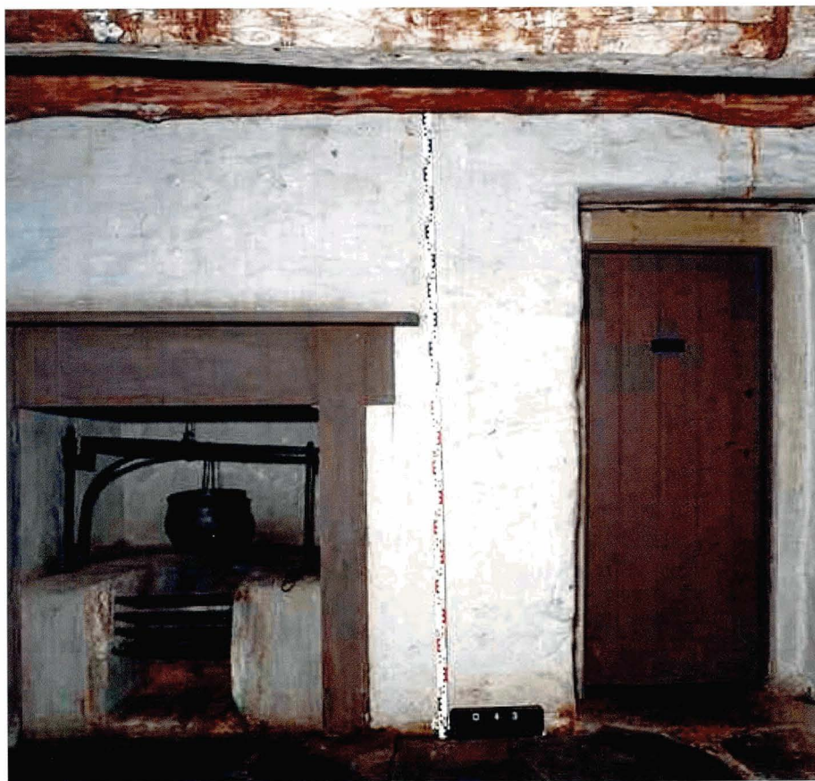
Illus 136 Internal elevation, represented as rectified photography. This image is part of a systematic photographic record prepared of the whole Township, comprising over 500 images. (Photo: C Hutchison, Historic Scotland)
