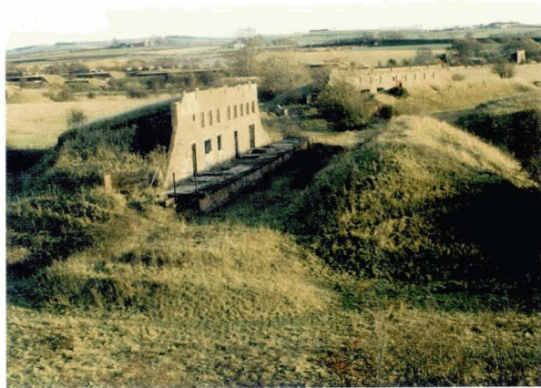
Illus 151 A general view of part of the site of Bowhouse Munitions factory, showing the spacious layout and bunds. (Photo: GUARD)
