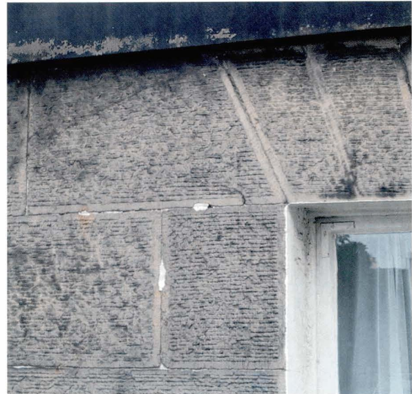
Illus 86 The form of surface tooling can be a guide to date, here horizontal droving in a detail from Edinburgh's New Town indicates a late C18 to mid C19 date. (Photo: Ross Dallas)
