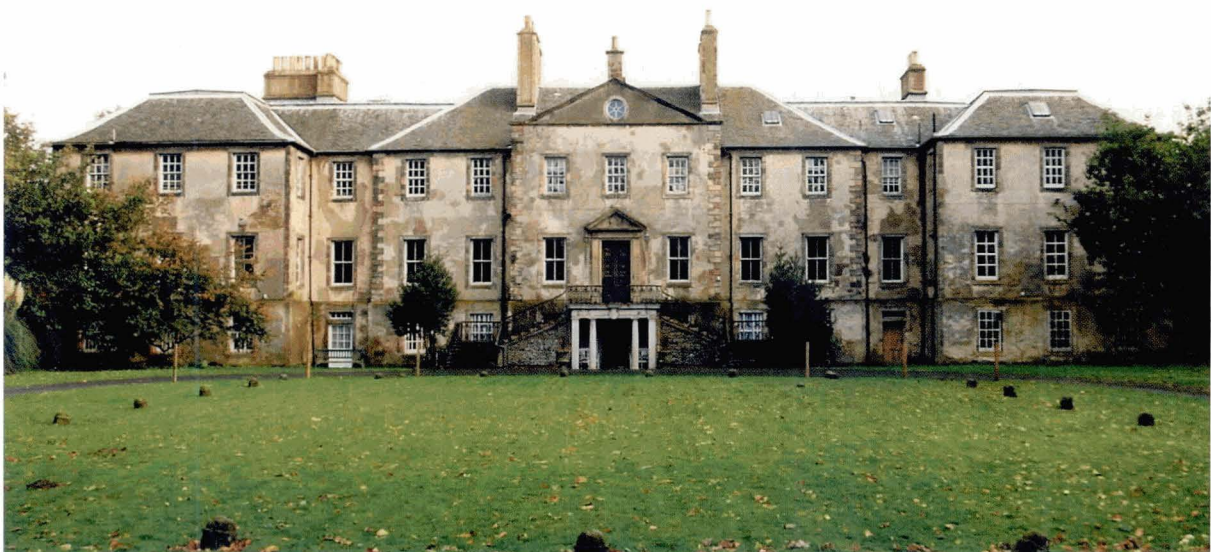
Illus 143 A general view of Newhailes House, south west front in 1998, before conservation works commenced. (Photo: JRA)
