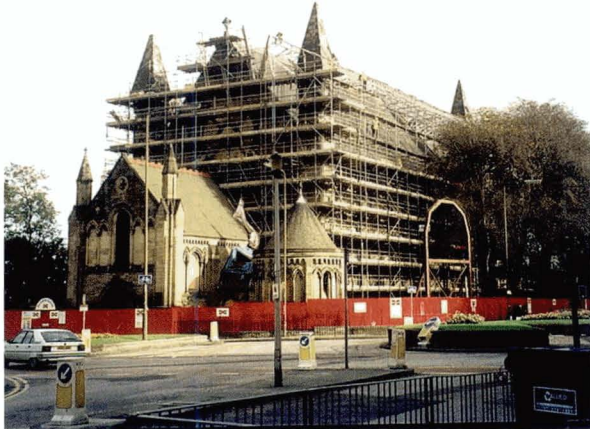
Illus 20 Mansfield Place Church from the west. (Photo: Simpson & Brown)
