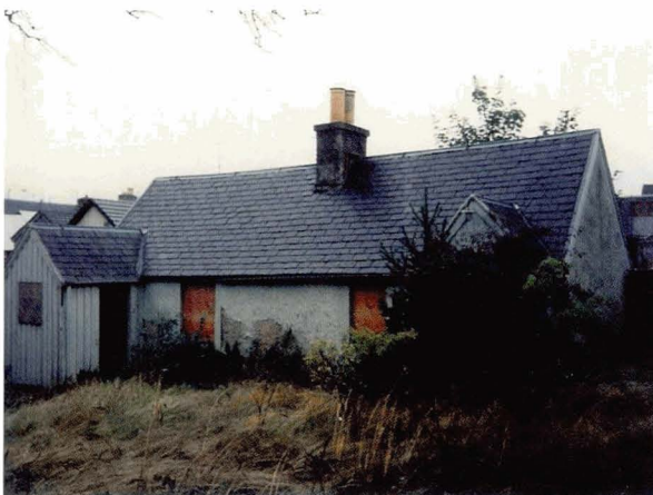
Illus 108 This apparently plain cottage in Grantown-on-Spey proved on investigation to have a post and beam structure dating to the C17. (Photo: GUARD)
