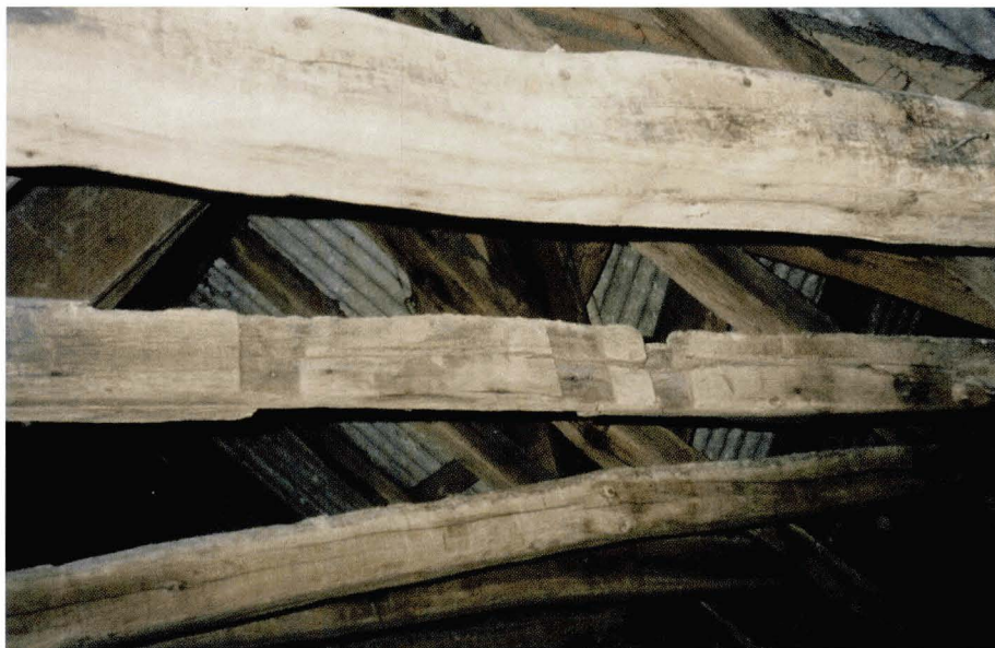
Illus 92 68 - 74 High St, Brechin. A group of oak timbers all felled in 1470 were found within the roof of this supposedly C17 house. They all bore redundant joints and duplicate carpenter's marks, indicating reuse. (Photo: AOC)
