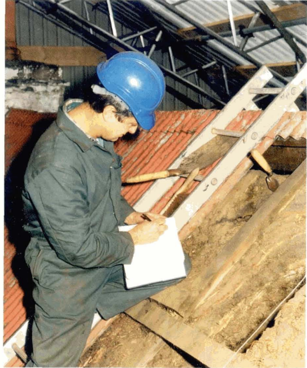
Illus 83 Sampling of a thatched roof, preserved under corrugated iron at Sunnybrae Cottage, Pitlochry. (Headland Archaeology Ltd, photo, Historic Scotland)
