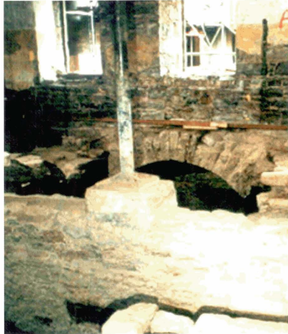
Illus 106 Wheelpit at Stanley Mills, Perthshire. This historical feature had been lost to view. The watching brief ensured that its significance was recognised and noted, ensuring that a proposed modern feature was moved to avoid damage to the pit. (Photo: Historic Scotland)
