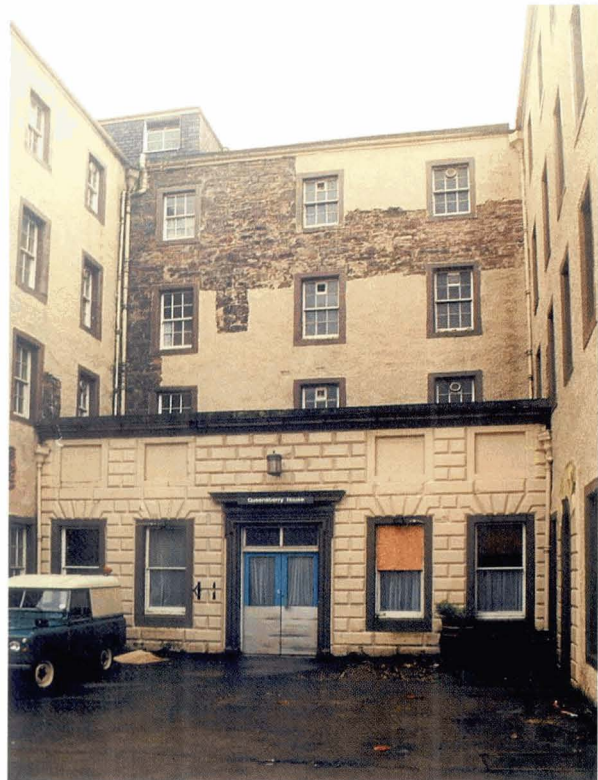
Illus 118 Queensberry House, Edinburgh, in 1999, looking south. Note the test areas of harling which had been stripped. (Photo: Ross Dallas)
