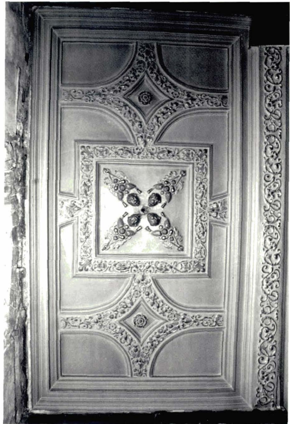
Illus 54 View of part of late C17 plastered ceiling, found on the first floor. (Photo: Andrew Hollinrake/Kirkdale)
