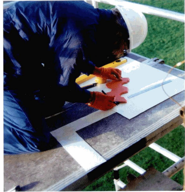
Illus 27 Transferring the profile to paper. The profile must be drawn off at 1:1, but this can then be digitised for transfer to a CAD program, when it can easily be rescaled. (Photo: Historic Scotland)
