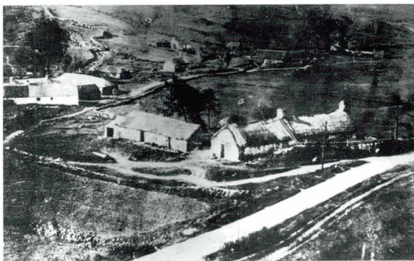
Illus 135 The Township in 1904. The buildings now described as houses A and B are in the foreground. Such early photography can provide invaluable information. For example, House A, then thatched, now has a corrugated iron roof. (Photo: Trustees of Auchindrain Township)
