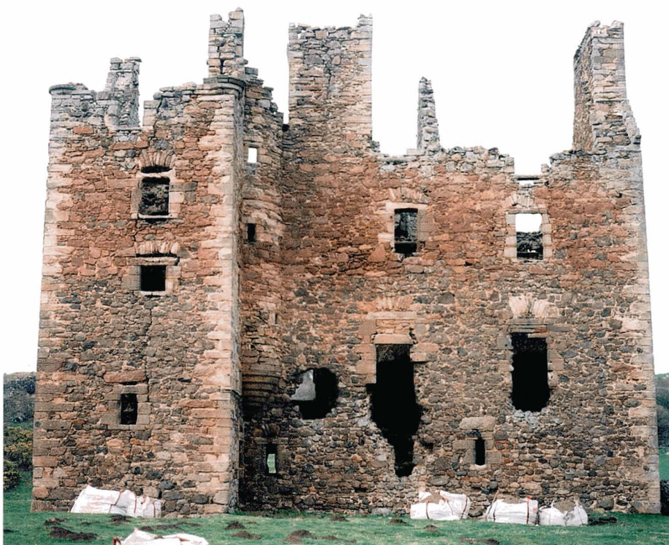
Illus 163 The Tower exterior, south face, with the stair turret projecting forward. The largely complete nature of the structure can be seen, allowing for reconstruction of the Tower without significant conjecture. (Photo: CFA Ltd)
