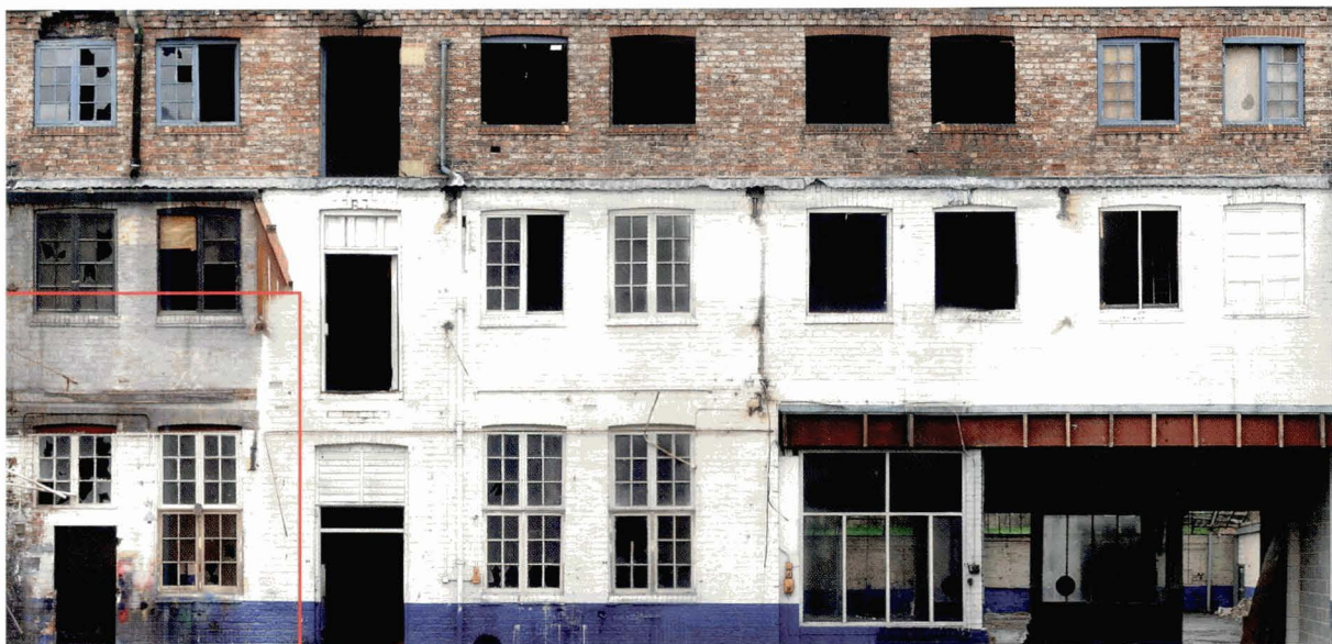
Illus 115 Photographic record of an exterior, presented as rectified photography, made up of a composite of several images. With digital input and modern computer programs, this type of product can easily be prepared. (Photo: Colin Briden)
