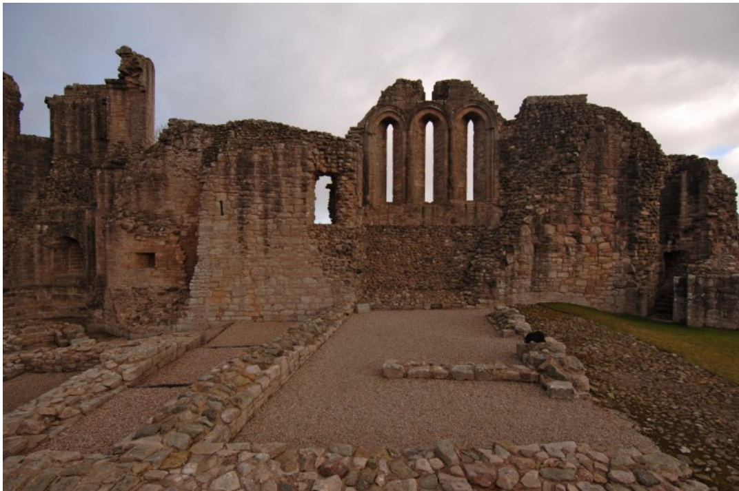
Figure 3: Interior view of chapel, looking north-east
