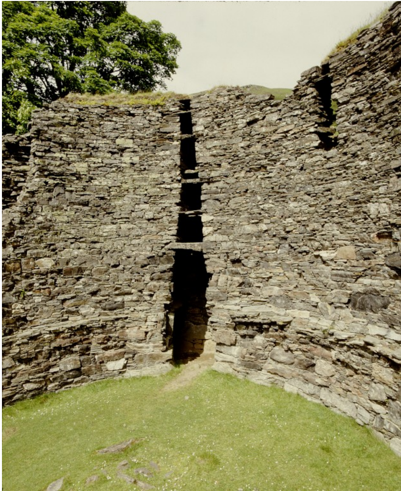
Interior, showing scarcement
