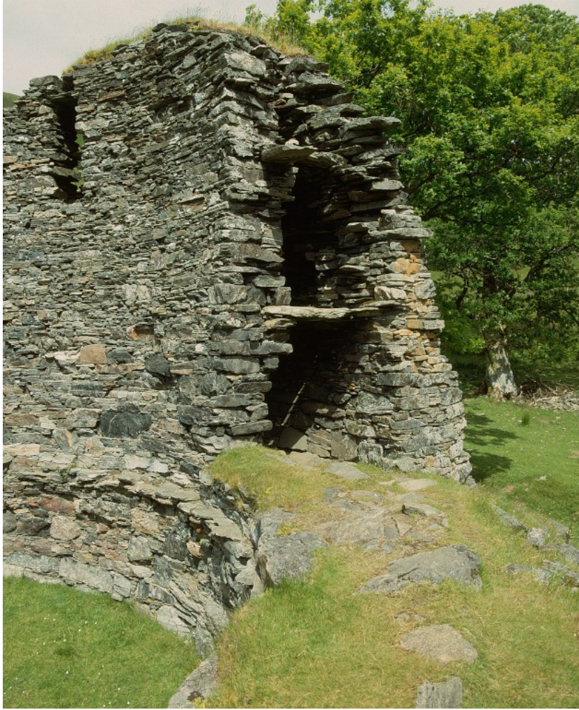
Eastern end of high-surviving wall, showing gallery levels: the smooth stonework on the inner wall may represent the last traces of a vertical void in the masonry.
