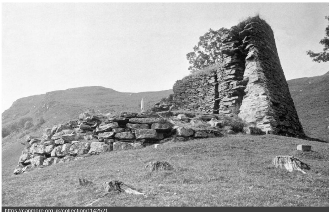
1897 photograph by Erskine Beveridge - with early cement repairs clearly visible on right
