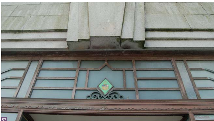
Fig. 57 Bronze window frames in an Art Deco style for a 1930s Co-operative building in Stonehaven
