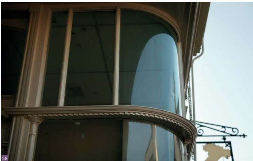
Fig. 58 Curved glazing is an important aesthetic element of some shopfronts
