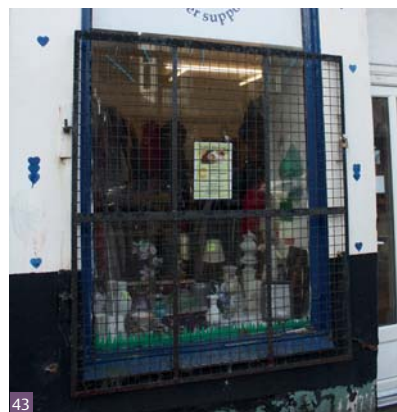
Fig. 42 Bespoke and lightweight modern shutters which protect the shopfront were installed in Bo'ness as part of the Townscape Heritage Initiative © L. Lennie
