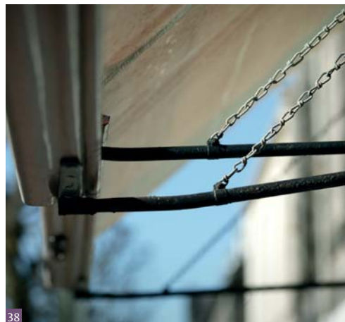
Fig. 37 Zig-zag arm mechanism in retracted position
