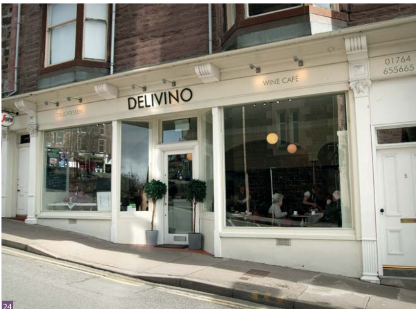
Fig. 24 Late Victorian shopfront with decorative cast iron columns by MacFarlane's Saracen Foundry (Crieff)
