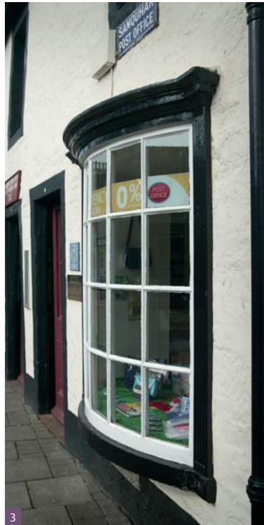
Fig. 2 Early shops typically had a fixed display window created from multiple small panes (Dunkeld)
