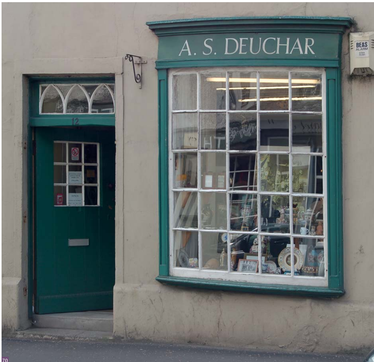
Fig. 70 Shop before conservation and repair
