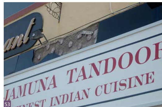
Fig. 53 Damage can occur to Vitrolite if care is not taken with fixings such as signage
