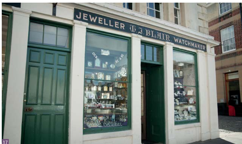
Fig. 17 Pilasters frame the shopfront. Early examples tend to be of a plain design, such as this one in Kelso
