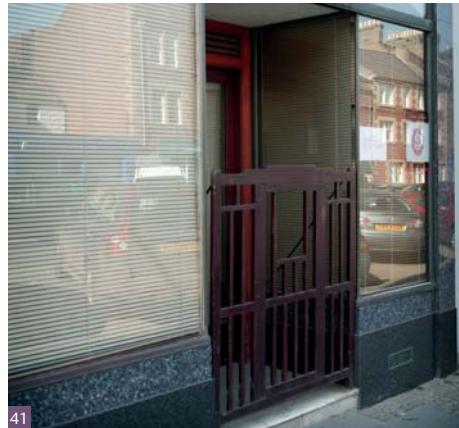
Fig. 40 Double storm doors protect the shop lobby when closed © L. Lennie
