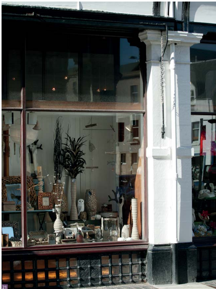
Fig. 21 Late Victorian shopfront with prismatic glass stallriser and pavement lights which direct light into the basement area (St Andrews)
