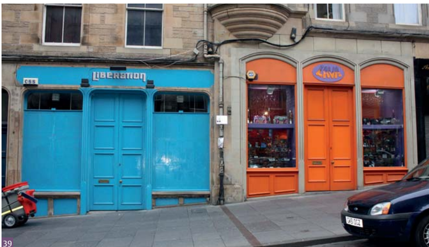
Fig. 39 Shops in Cockburn Street, Edinburgh are fitted with rising shutters. The blue shop on the left has the shutters in the closed position © L. Lennie
