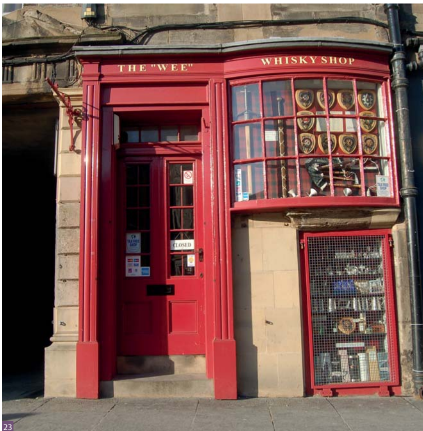
Fig. 23 Georgian shopfronts used multiple paned windows, sometimes set in a bowed frame with a narrow fascia (Edinburgh)
