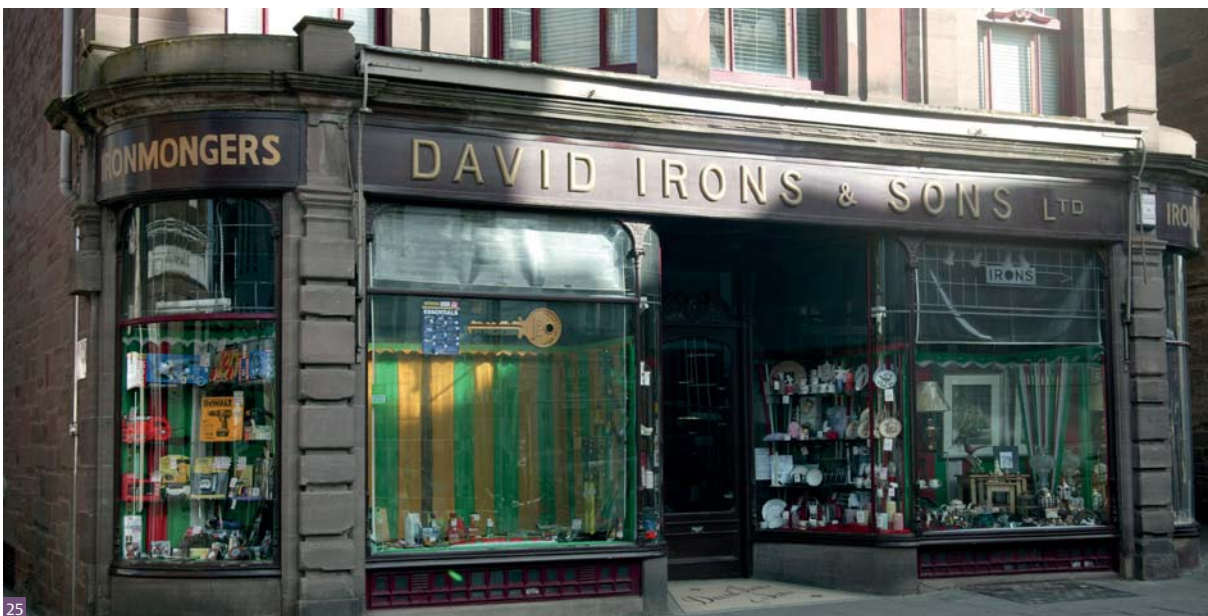
Fig. 25 Edwardian shopfront with curved glazing, mosaic entrance and decorative clerestory (Forfar)
