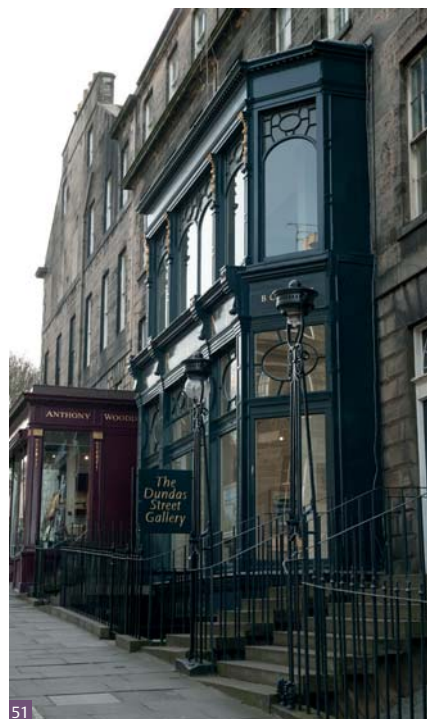
Fig. 50 Use of contrasting colours can help to highlight architectural detail
