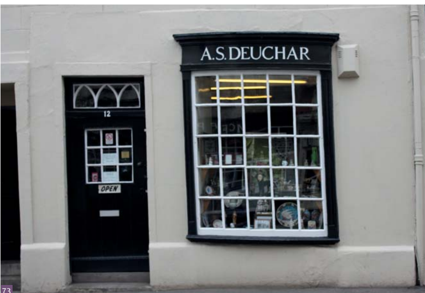
Fig. 73 The shopfront after repairs and repainting
