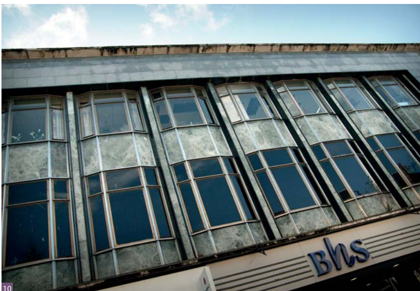
Fig. 10 Polished stone cladding and metals like bronze were widely used in the design of inter-war and post-war shopfronts, including this former department store in Perth dating from 1960
