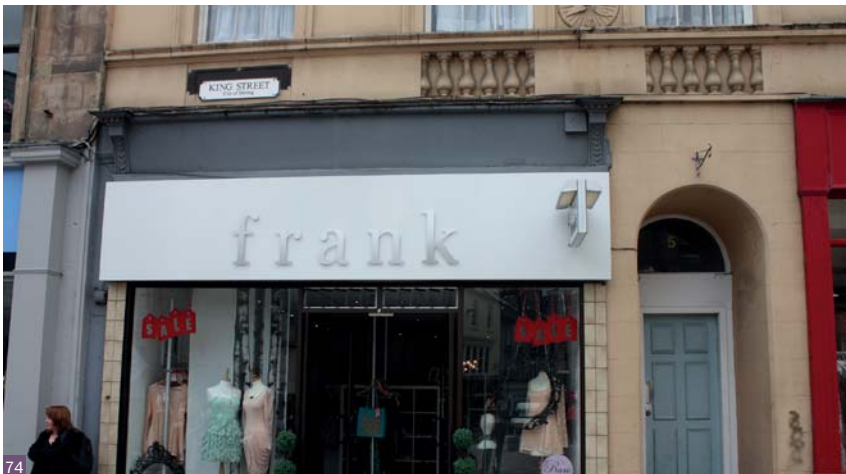
Fig. 74 Modernised shopfront in Stirling with aluminium windows, modern tiled stallriser and poorly proportioned signage, but the Victorian fascia above survives © L. Lennie
