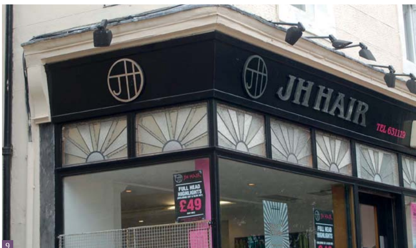
Fig. 9 Sunrise motif incorporated into the glazing of a 1930s shopfront (Falkirk)
