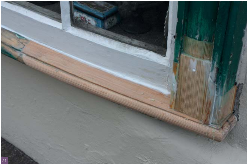
Fig. 71 Part of sill replaced in matching timber
