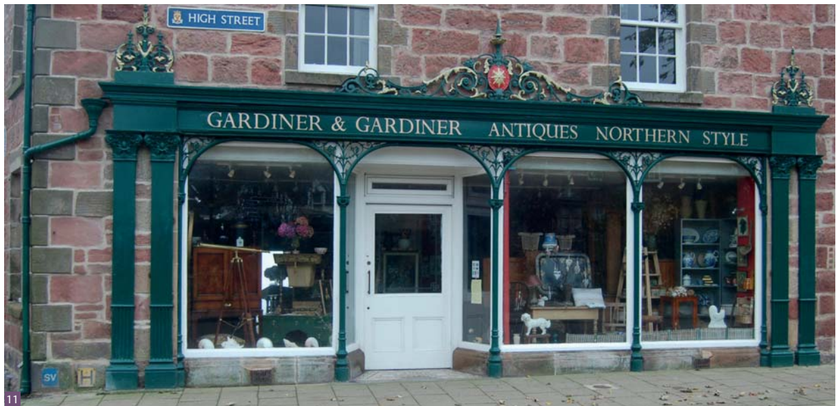
Fig. 11 Cast iron shopfront, Cromarty, by Saracen Foundry, Glasgow
