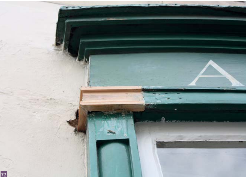
Fig. 72 Small area of fascia replaced
