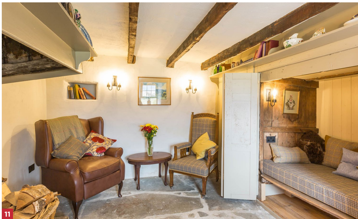
Figure 11. The fire performance of this modest timber ceiling was improved by the addition of a lime plaster between the joists. © Calum Innes.
