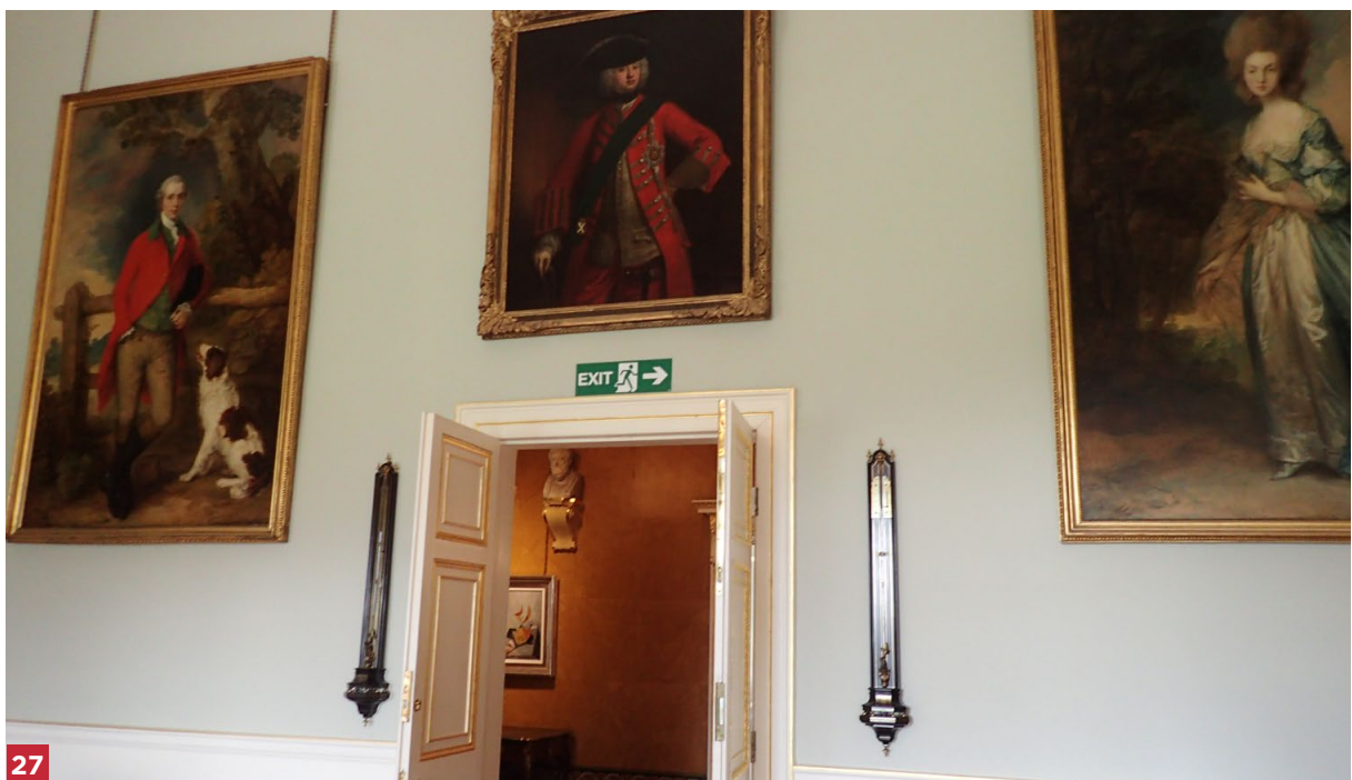
Figure 27. Standard escape signage can look out of place in a historic setting.
