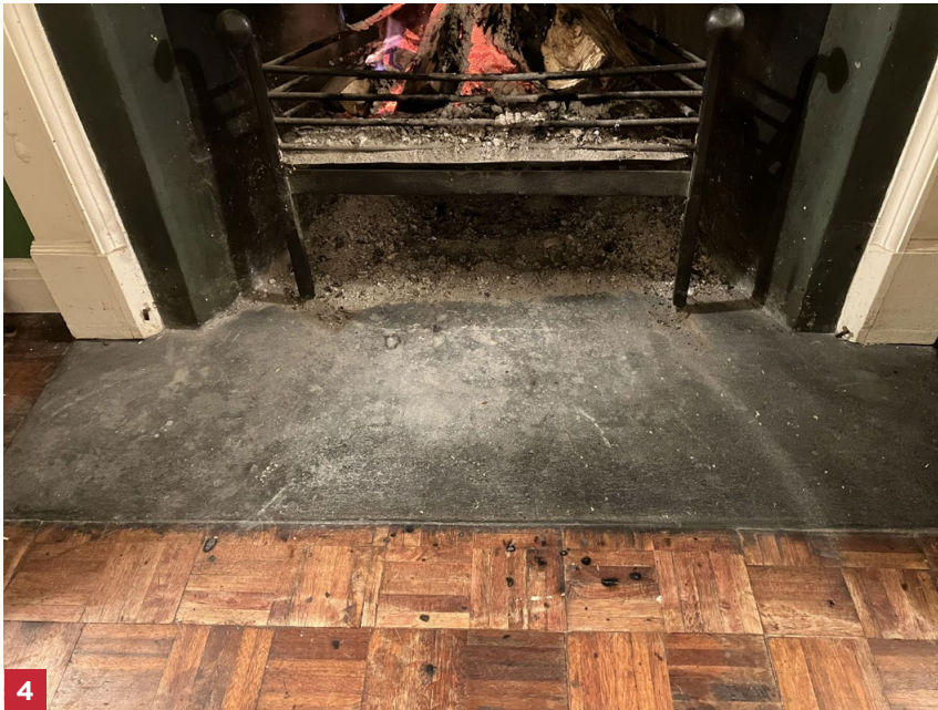
Figure 4. This previously damaged hearthstone has been repaired with a repair mortar. Note the wrought-iron basket designed to fit the opening and to burn logs.
