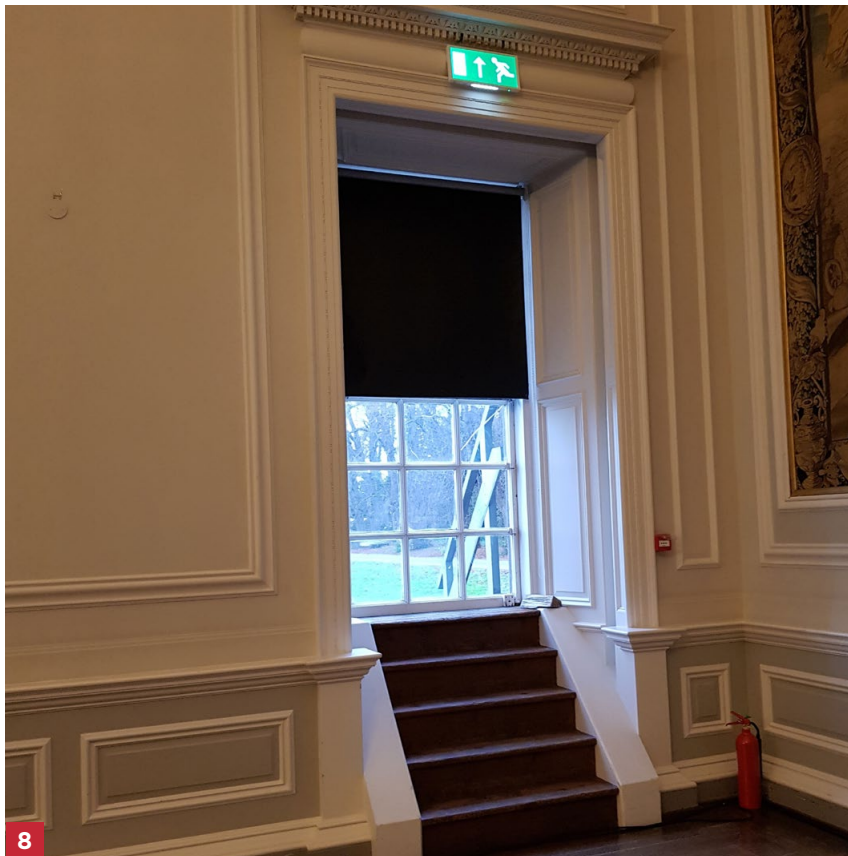
Figure 8. A category A-listed building where a window has been sympathetically converted into an additional fire escape route.
