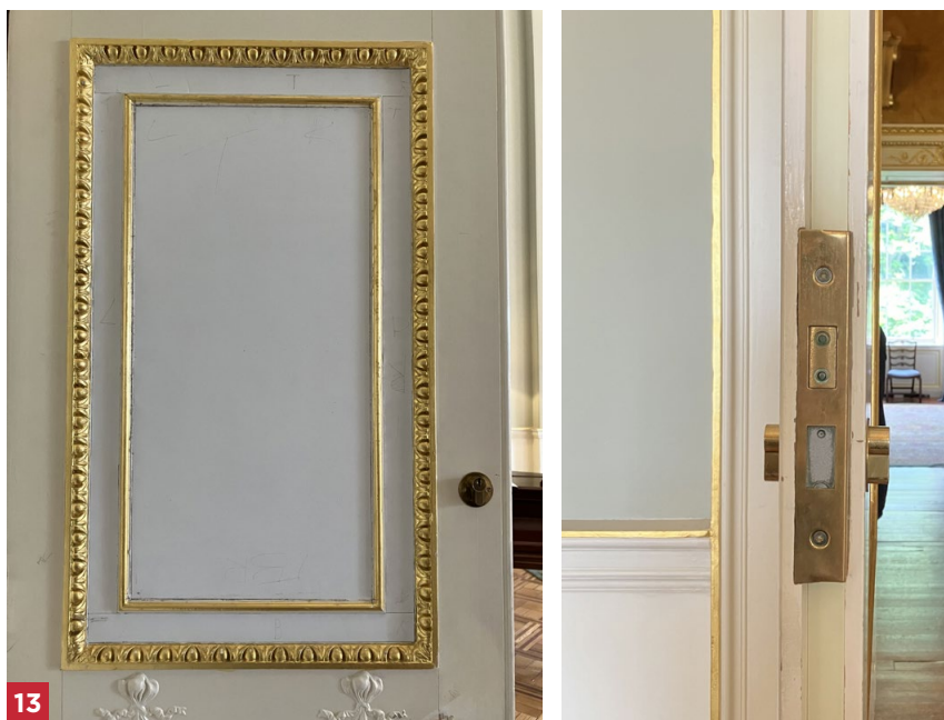
Figure 13. At category A-listed Duff House in Banff, there was a need to improve the fire resistance of doors. This was achieved by the insertion of intumescent paper on the panels of the doors and intumescent strips around the door edges.
