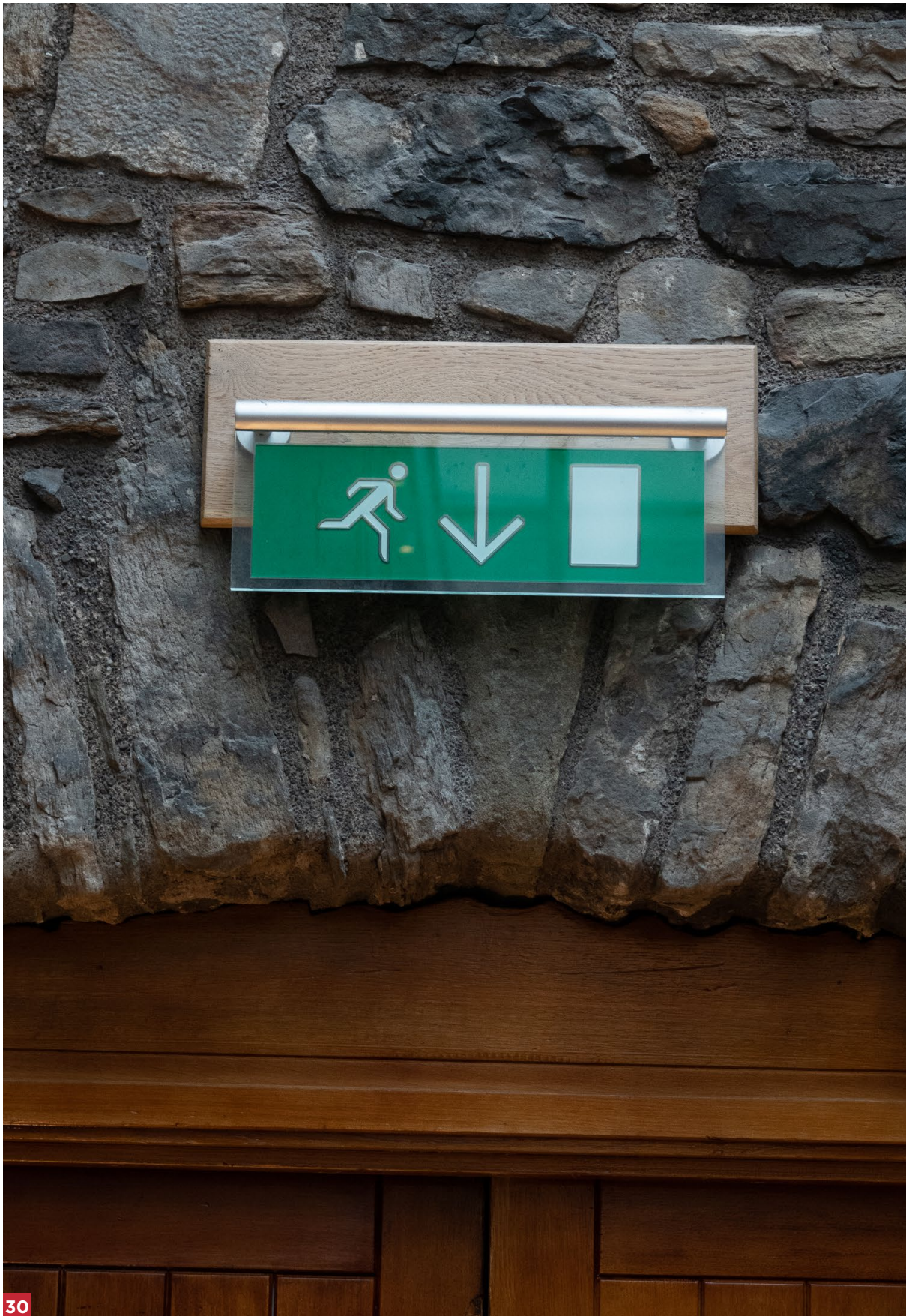
Figure 30. Lighting and signage combined with a chrome fitting.
