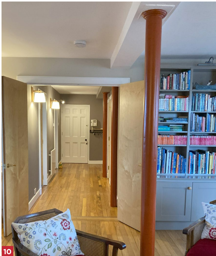
Figure 10. These columns were retained as a fire risk assessment identified that the fire suppression system would control the spread of fire and the damage to the columns.
