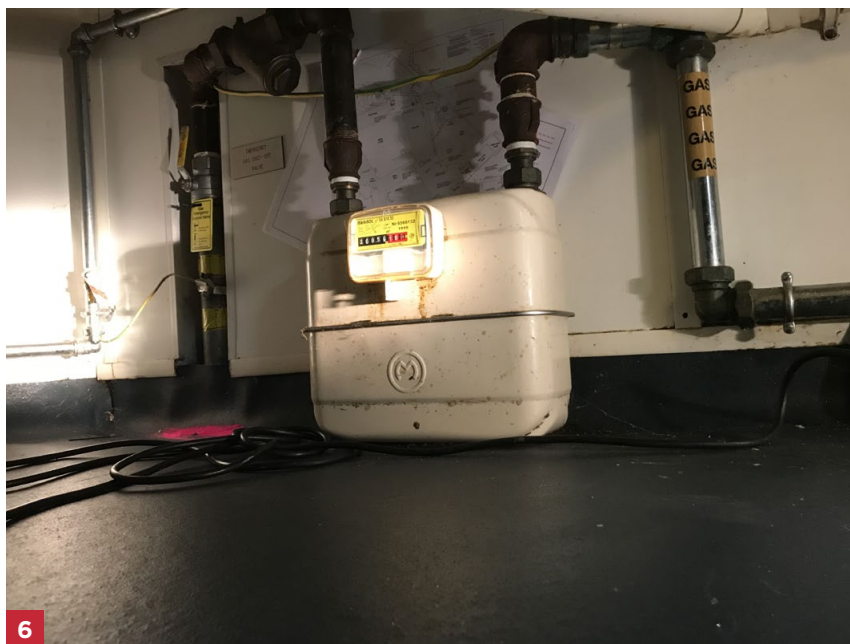
Figure 6. Gas meter in the Great Hall kitchen at Stirling Castle with a compression fitting (the elbow below and above the 'Gas' marker tape on the chrome pipe at the right of the meter). Such fittings can be mandated at tender stage to eliminate hot works on site.
