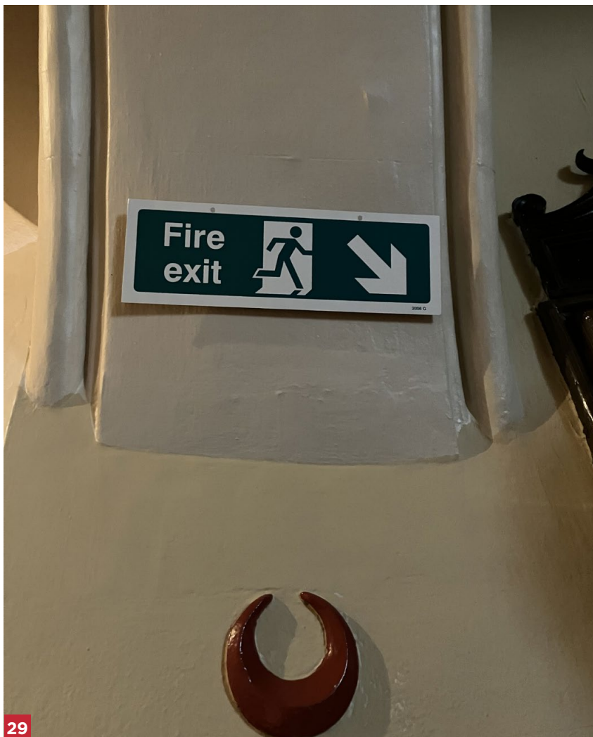
Figure 29. A fire exit sign at Fyvie Castle, which is attached to the wall using velcro rather than being surface mounted.
