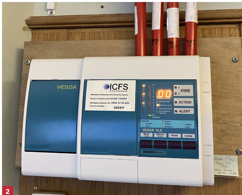
Figure 2. Duff House in Aberdeenshire has an air aspirating fire detection system designed to protect the contents as well as the occupants. The system features a sampling point that is constantly sampling the air for smoke particles, allowing for a fast response to a potential fire.
