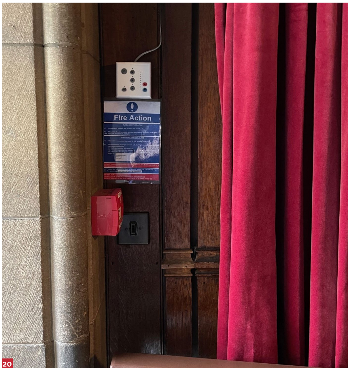
Figure 20. A discreet manual call point.
