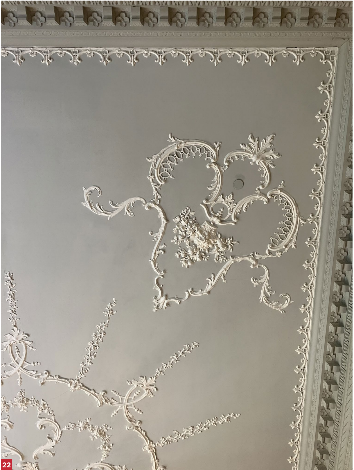
Figure 22. Concealed sprinkler heads in the decorated ceilings at Duff House have coloured caps to blend with interior finishes in the rooms.
