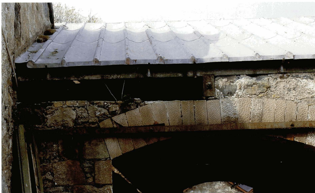
Illus 8 The Steading, Torosay Castle ©Bruce Walker. The use of profiled cladding sheets
