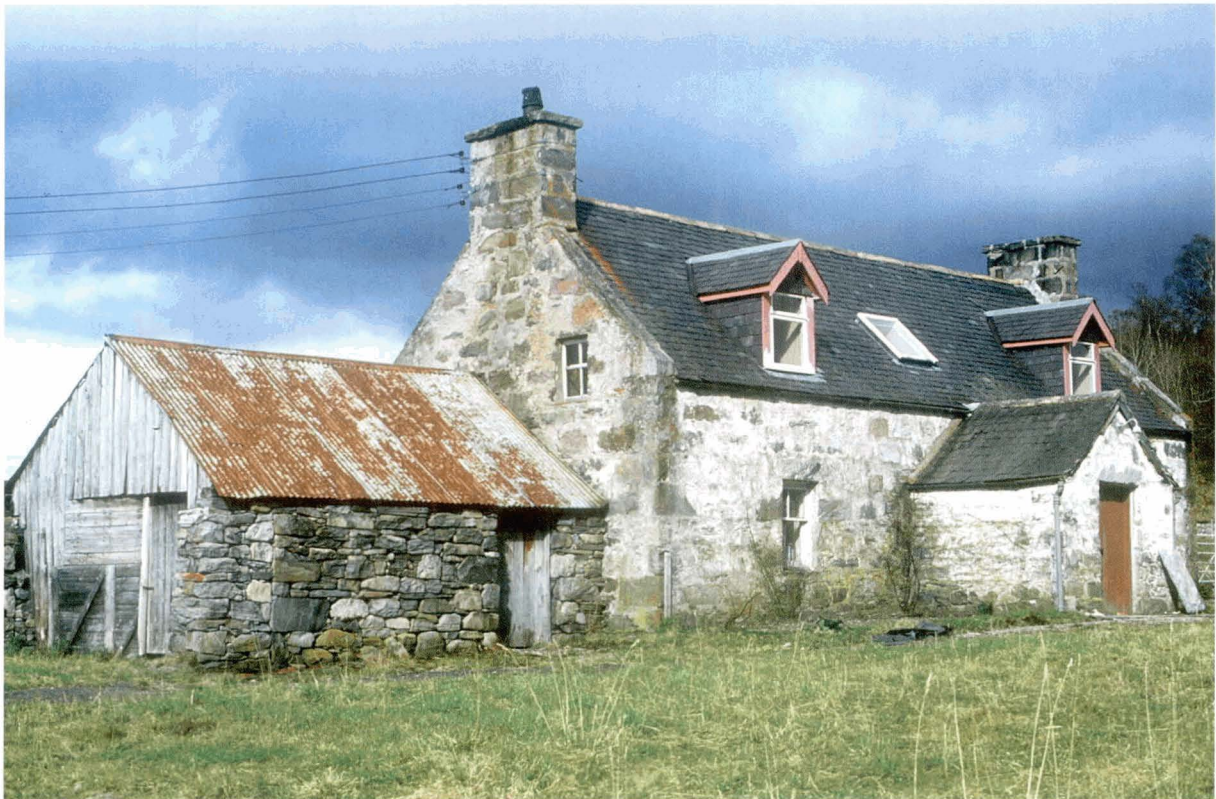
Illus 17 Tromie Mill, Moray. Outbuilding roofed in corrugated iron. © Ingval Maxwell
