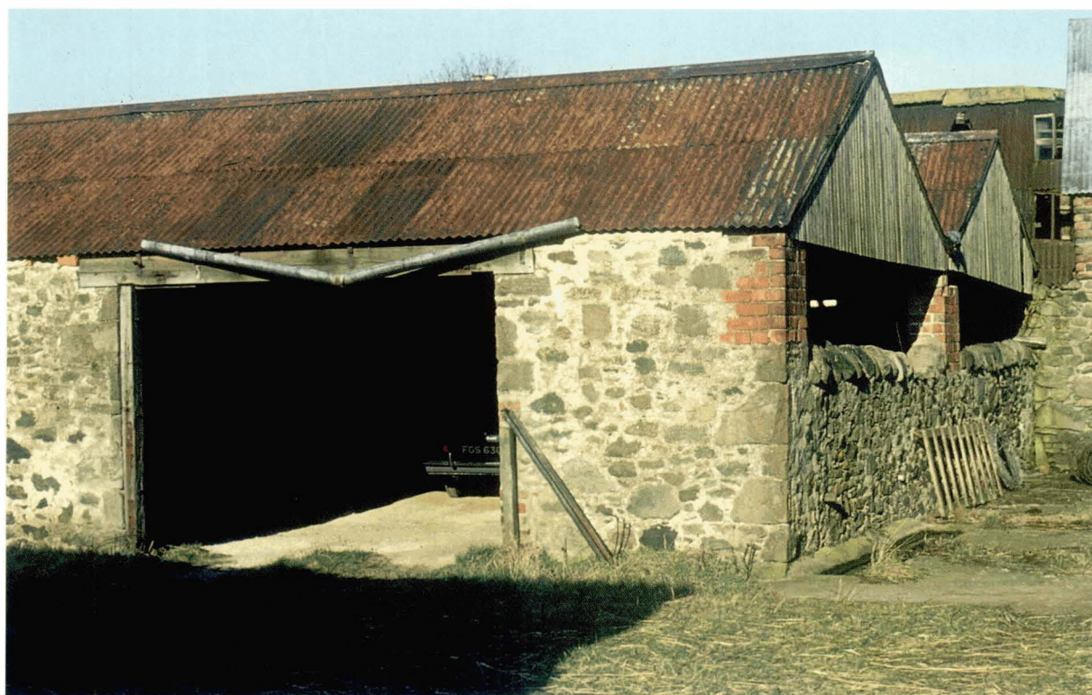
Illus 12 Whiteriggs Farm Cattle Wintering Courts. As previously open Cattle Courts were roofed over toward the end of the 19thC corrugated iron sheeting was a favoured material to use for the roof covering. © Ingval Maxwell
