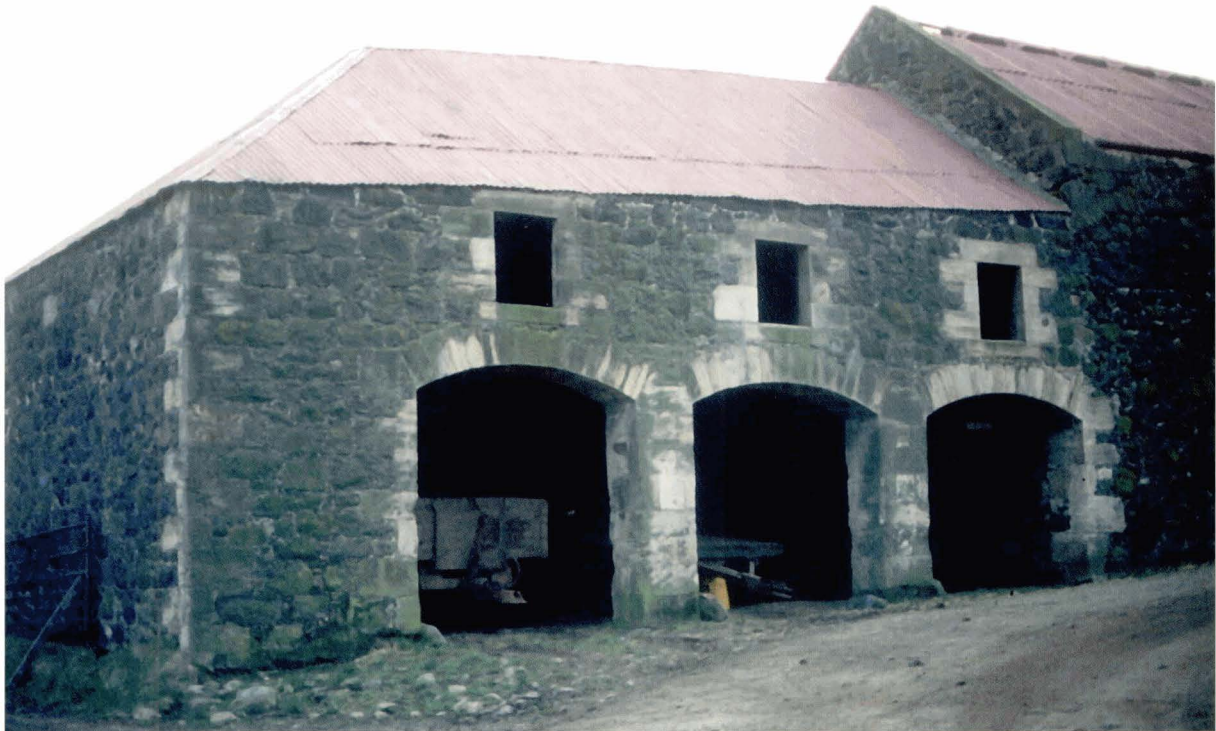
Illus 16 Dogton Farm Cartshed, Fife. Mid 19th C building roofed in corrugated iron. © Ingval Maxwell
