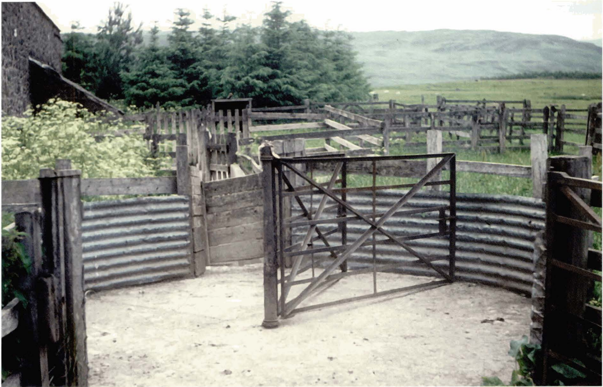
Illus 23 Kilburn, Angus: Sheep dip construction incorporating angle iron gates on a steel post and curve profiled corrugated iron side sheets © Ingal Maxwell
