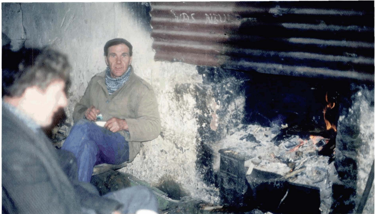
Illus 24 Brothershields, Midlothian: corrugated iron sheet smoke board in farm bothy © Ingval Maxwell
