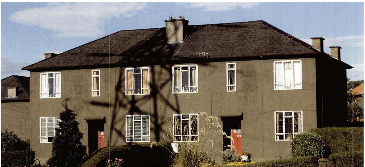
Illus 9 Houses in Dundee, Angus ©Bruce Walker. The use of sheet metal walling panels
