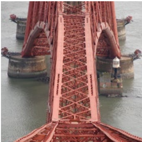
View showing the construction of the Bridge.
