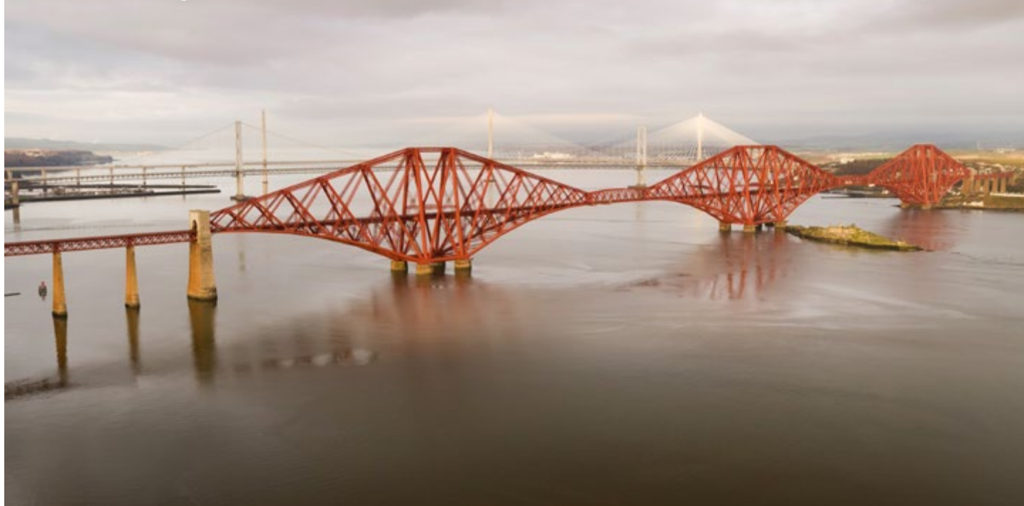
The three Forth Bridges from the air looking west.
