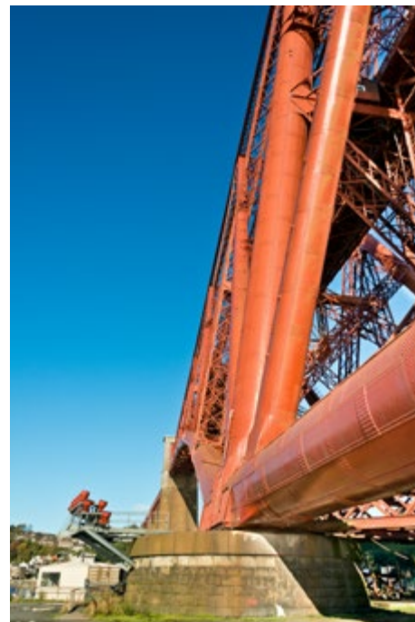
North west caisson, columns and diagonal bracing Fife cantilever.
