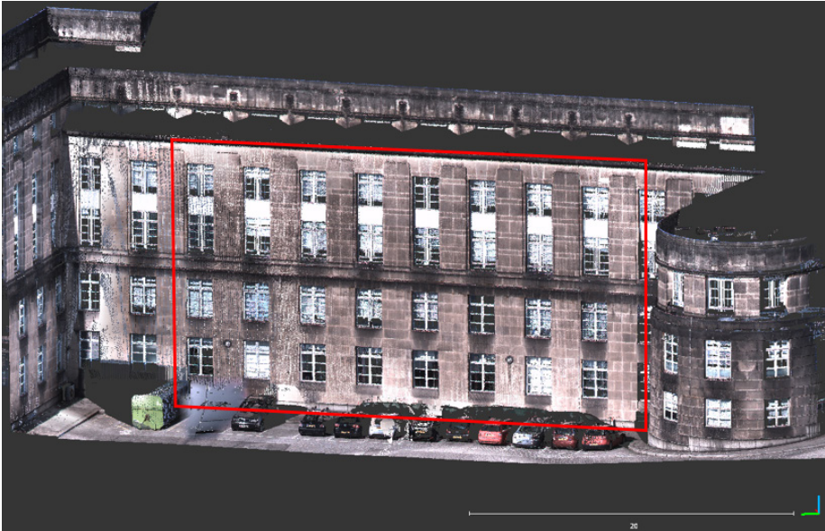
Figure 12: South-eastern façade of St Andrew's house. The region of interest is highlighted in red.
