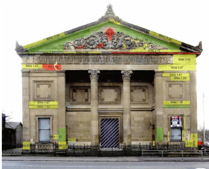
Figure 1: Rectified image of façade with overlays showing stone decay codes and repair needs. Image reproduced from Stonemasonry skills and materials (2007).
