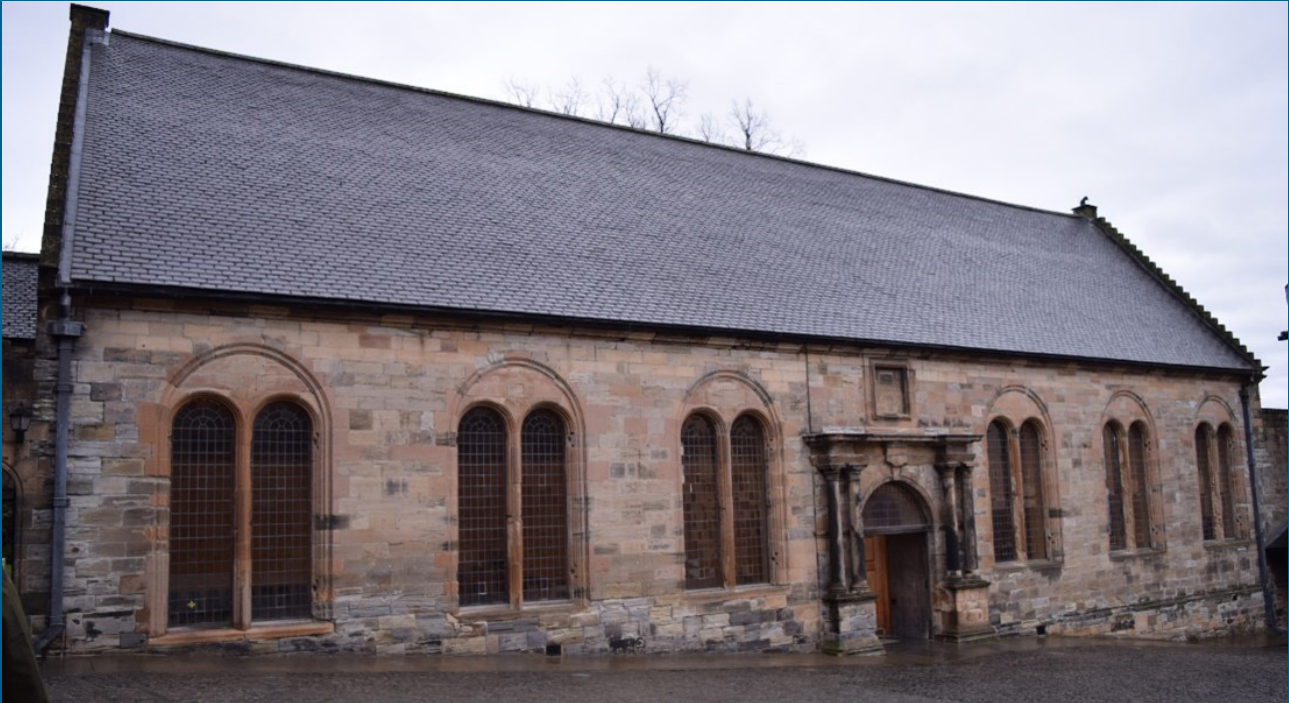
Figure 20: South façade of the Chapel Royal in Stirling Castle.
