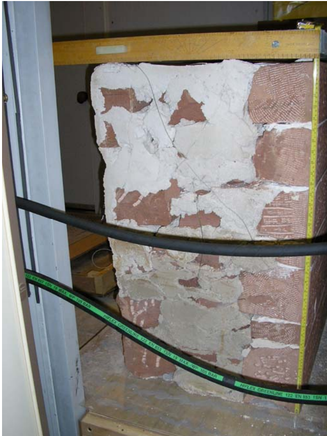
Figure 3: Solid wall construction. The example is of a test wall built by Historic Scotland's masons for GCU from Locharbriggs sandstone (see Laboratory measurement in section 5 ). The outer leaf (right) has an ashlar finish, whilst the inner leaf is a rubble construction. It has been estimated that the proportion of mortar in the wall is about 30% by volume.
