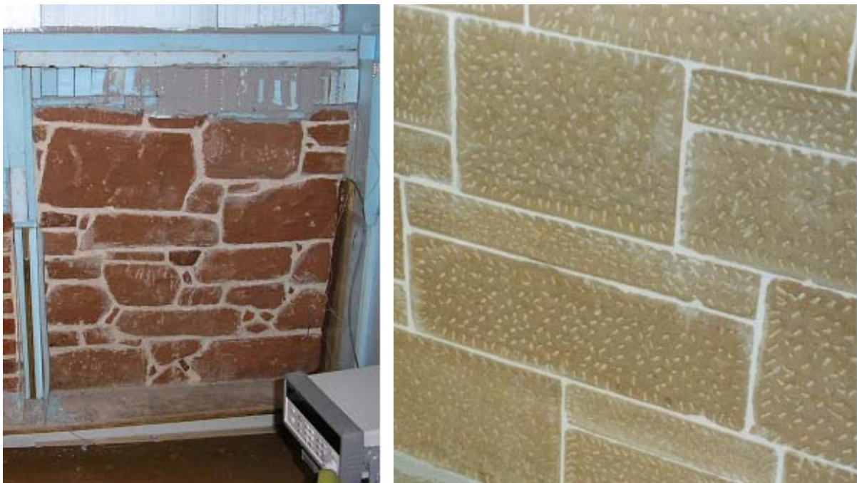
Figure 14. Locharbriggs sandstone wall in test chamber. The left photo shows the internal rubble face; the right photo the external ashlar face.
