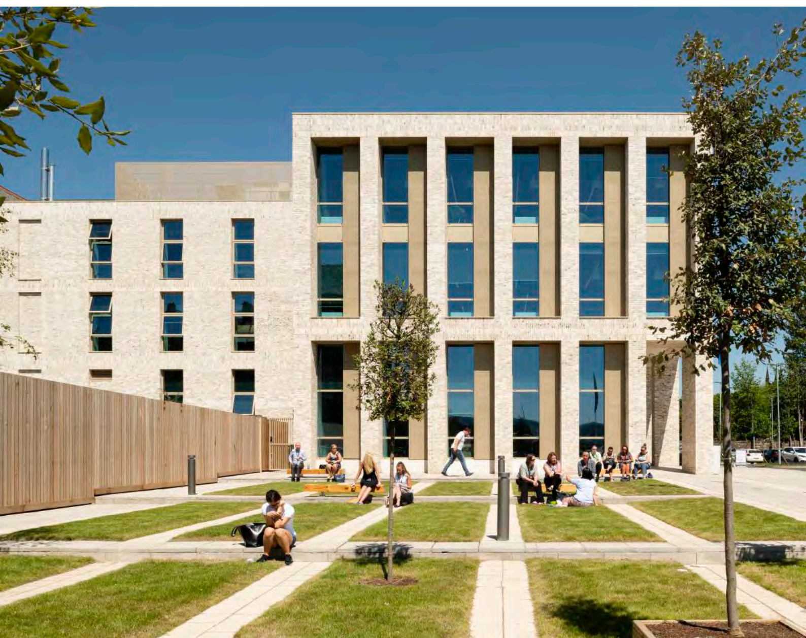
Below: View of the extension added to the rear of the building © Jim Stephenson
