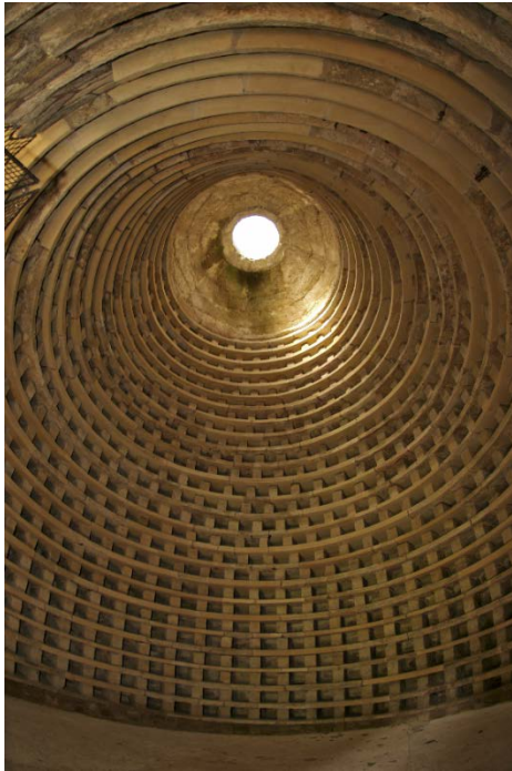
Interior view of Dirleton doocot
