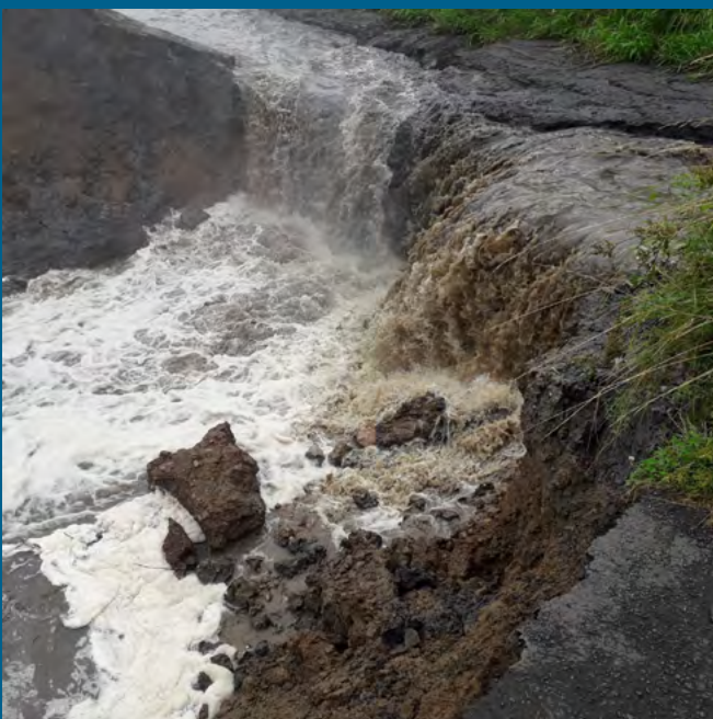
Images of the breach prior to installation of temporary dams to stem the flow of water. Over 11,000 fish were rescued from the flood waters below the breached section. Images © Scottish Canals
