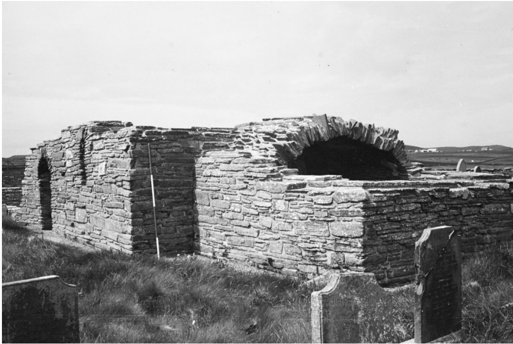
Figure 5: 1981 image looking north-west. Note remains of the barrel vaulted chancel roof. © Dr. Raymond G. Lamb.
