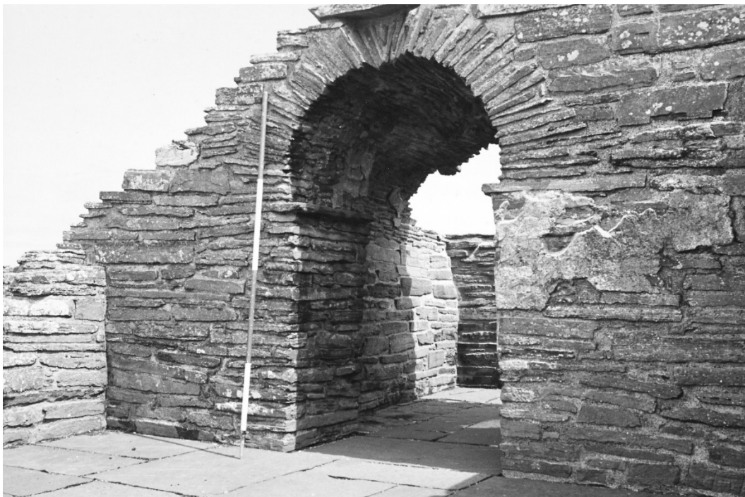
Figure 4: 1981 image of arch leading to barrel-vaulted chancel, looking north-east. Note traces of plaster adhering to walls within nave. © Dr. Raymond G. Lamb.
