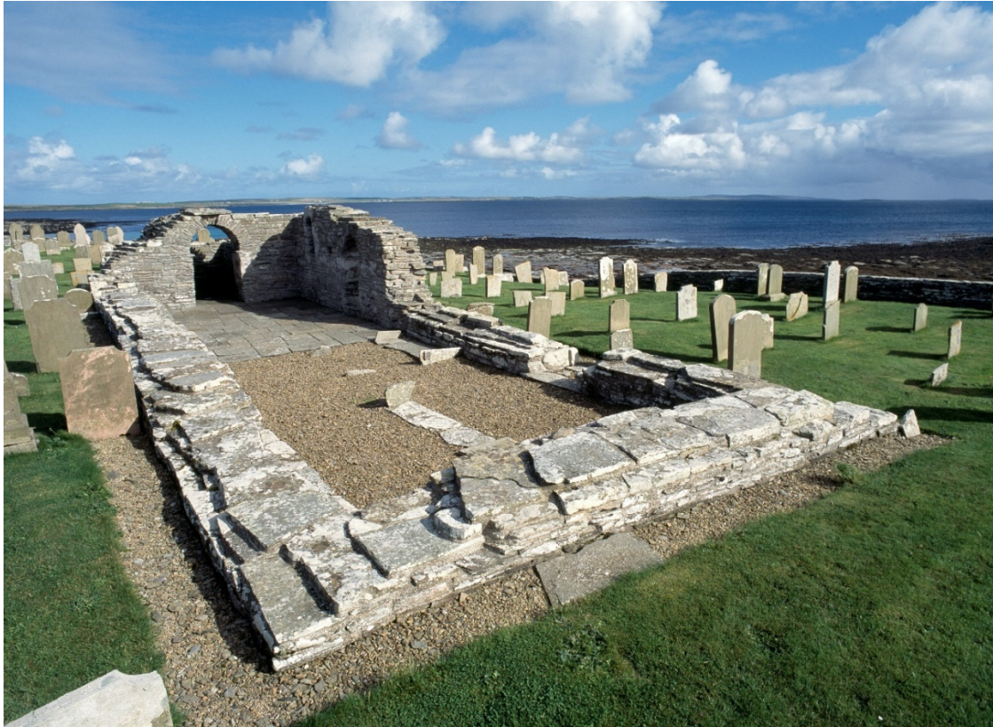
Figure 2: view from north-west, with internal paving demarcating the original footprint of the nave, before its extension to the west. © Crown Copyright: HES.
