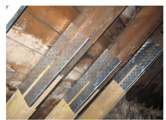
Modern metal pre drilled straps used in rafter splices.
