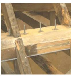
Composite repair using resin, new timber and steel plate
