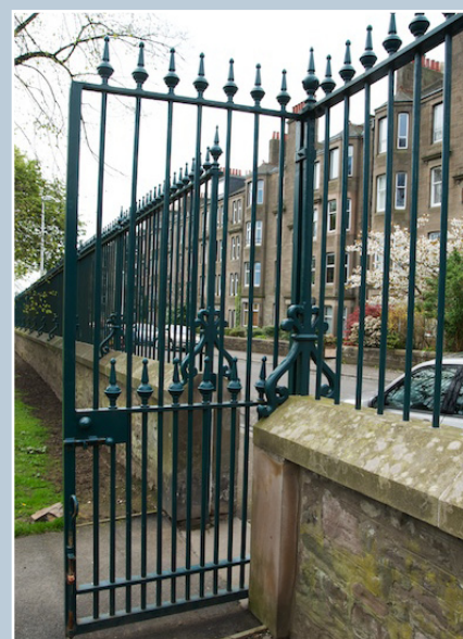
Railings reinstated in 2006 define the edge of Baxter Park, Dundee, and are key to its regeneration and good management. The patterns were deduced from a short surviving section.
