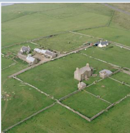
Like many 18th- and 19th-century buildings in Shetland, Belmont House (1777), Unst, stands at the centre of an extended formal arrangement of field boundaries. This aerial view was taken in 2005 before the recent restoration of the house. © Crown copyright: RCAHMS. Licensor www.rcahms.gov.uk .
