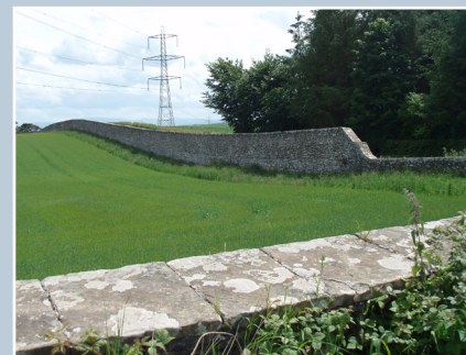
Boundary walls at a country estate in the Scottish Borders.
