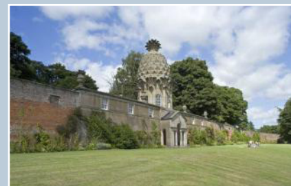
The famous 1761 Pineapple pavilion (now a holiday cottage) forms part of the boundary of the walled garden at Dunmore, Falkirk. Pineries originally flanked the entrance: heating and ventilation shafts for the glass houses are built into the brick walls. © Crown copyright: RCAHMS. Licensor www.rcahms.gov.uk .
