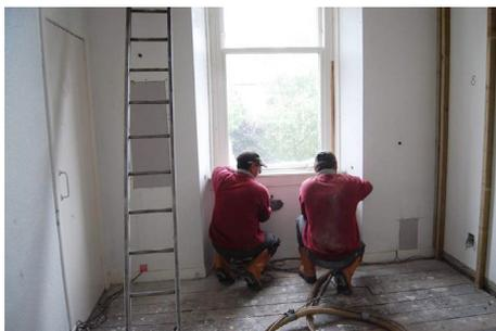
*Fig. 8 Insertion of bonded polystyrene bead insulation behind plasterboard.*
