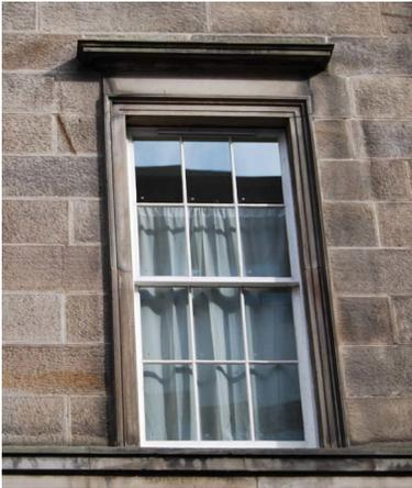
*Fig. 6 Vacuum pane glazing inserted into original window.*
