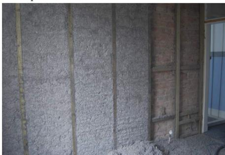
*Fig. 9 Blown cellulose material applied to mass masonry wall between timber strapping.*
