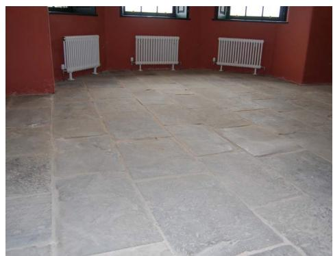
Fig. 3 Stone flags back in place after the laying of an insulated lime concrete floor.
