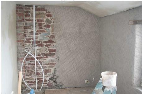
*Fig. 10 Insulated lime plaster on a traditional mass wall.*
