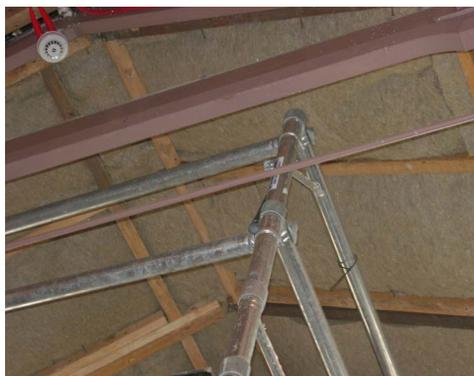
*Fig. 2* Wood fibre board fastened between rafters.
