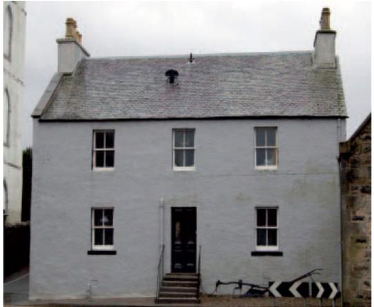
*Fig. 7 Where inappropriate cement render has been applied to a traditional building its replacement with an insulated lime based material may be appropriate.*
