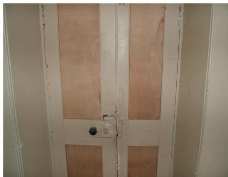
*Fig. 4 A 19th century timber door with insulation installed in the panels.*
