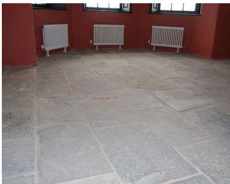
*Fig. 3* Stone flags back in place after the laying of an insulated lime concrete floor.
