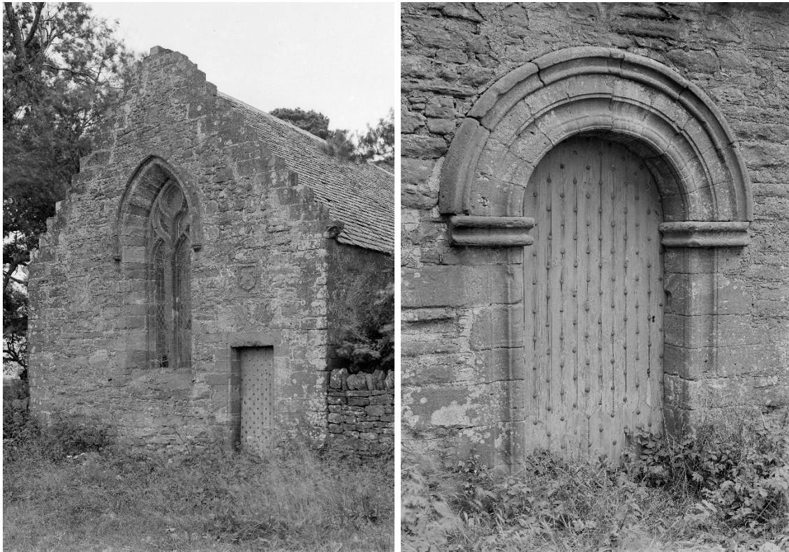
Figures 2a and 2b: Photographs from 1929. a) View of north transept gable, including window with uncusped loop tracery. b) View of round-headed south doorway. Both © Courtesy of HES (B C Clayton Collection).
