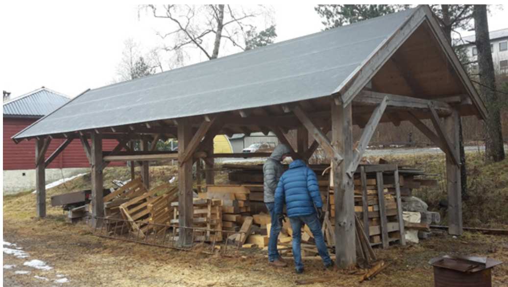
Fig. 6: A traditionally-framed timber structure called a Gapahuk. This structure was a training project built in two weeks by Voss second-year students for a local family. 34
