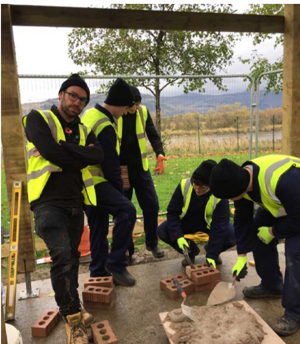
Figures 7 and 8: Students work together with skilled HES crafts people to construct a timber-framed bicycle shed with masonry foundations.
