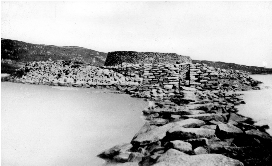
SC 1151590 © Courtesy of HES. - Unattributed photo apparently taken between 1861 and 1874 (on evidence of the loch level): note the modern blocking wall across the causeway.
