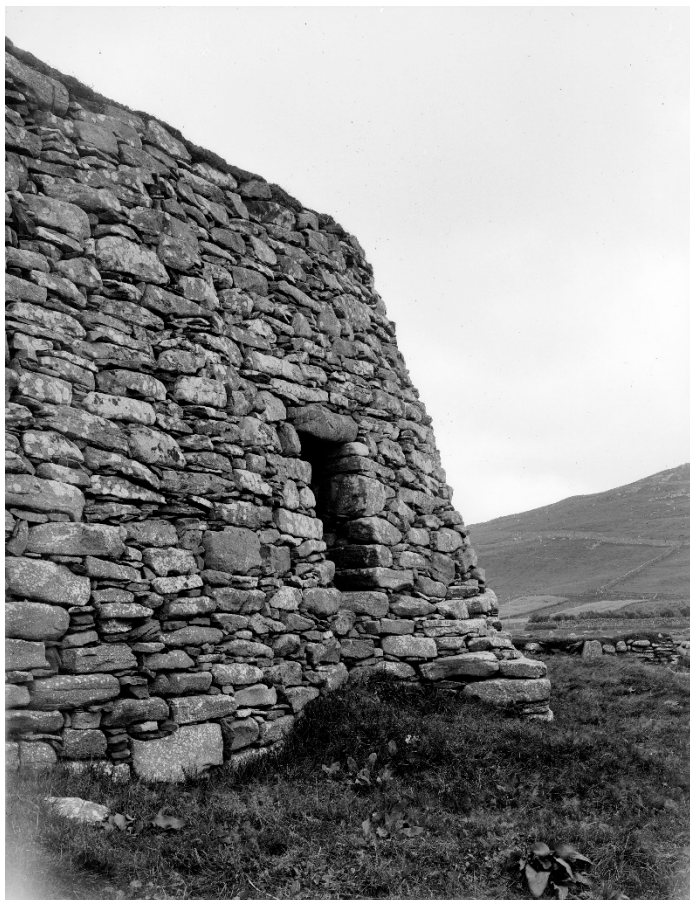
SC 1224136 © Courtesy of HES. The spur wall and second entrance in the broch wall.
