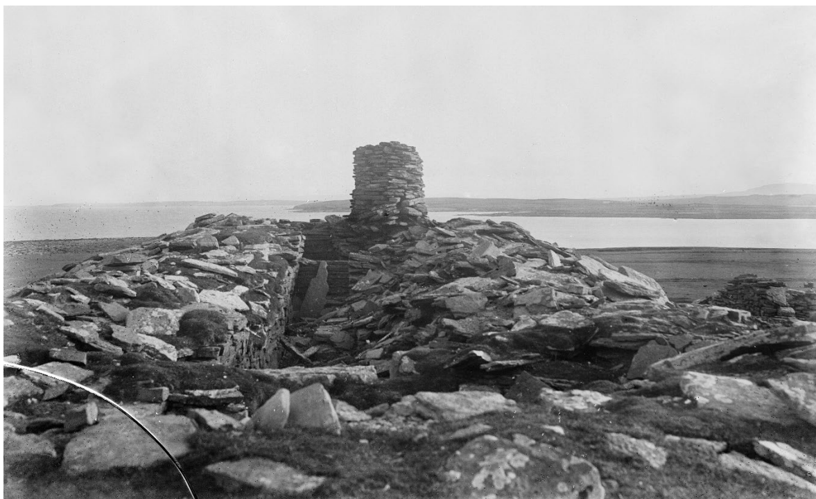
Figure 2: Early 20th century image (1929?), prior to limited consolidation and installation of concrete roof in the 1931. Following its excavation, the tomb was left open and suffered considerable deterioration prior to entering State care. Note presence of drystone stack as naval navigation marker cairn on the highest part of the island. © Crown Copyright: HES.
