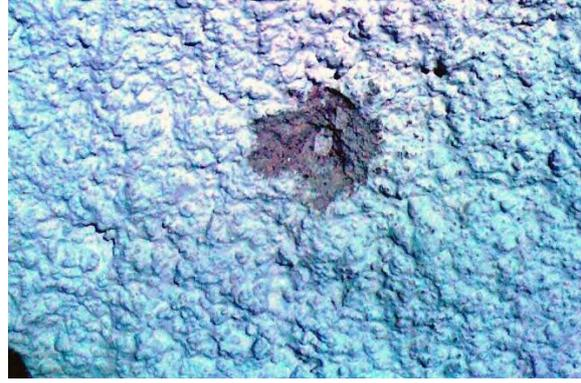
Figure 3: Pitted harl finish caused by the expansion of a particle of slow slaking quicklime after placing
