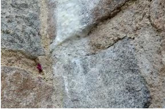
Figure 3: Leaching of mortar caused by poor building detailing and excessive wetting of masonry
