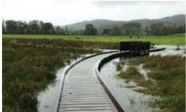
Flooding in Kilmartin Glen, with new raised walkway maintaining access.
