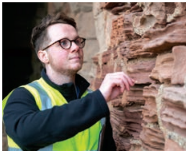
Inspecting decay of masonry at Tantallon.
