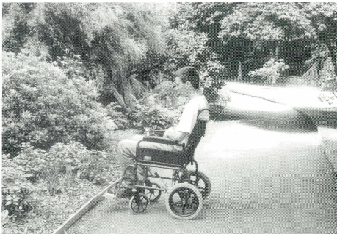
Plate 6. Fyvie Castle - Wooden kerbs to contain grass and earth and act as tapping rails
