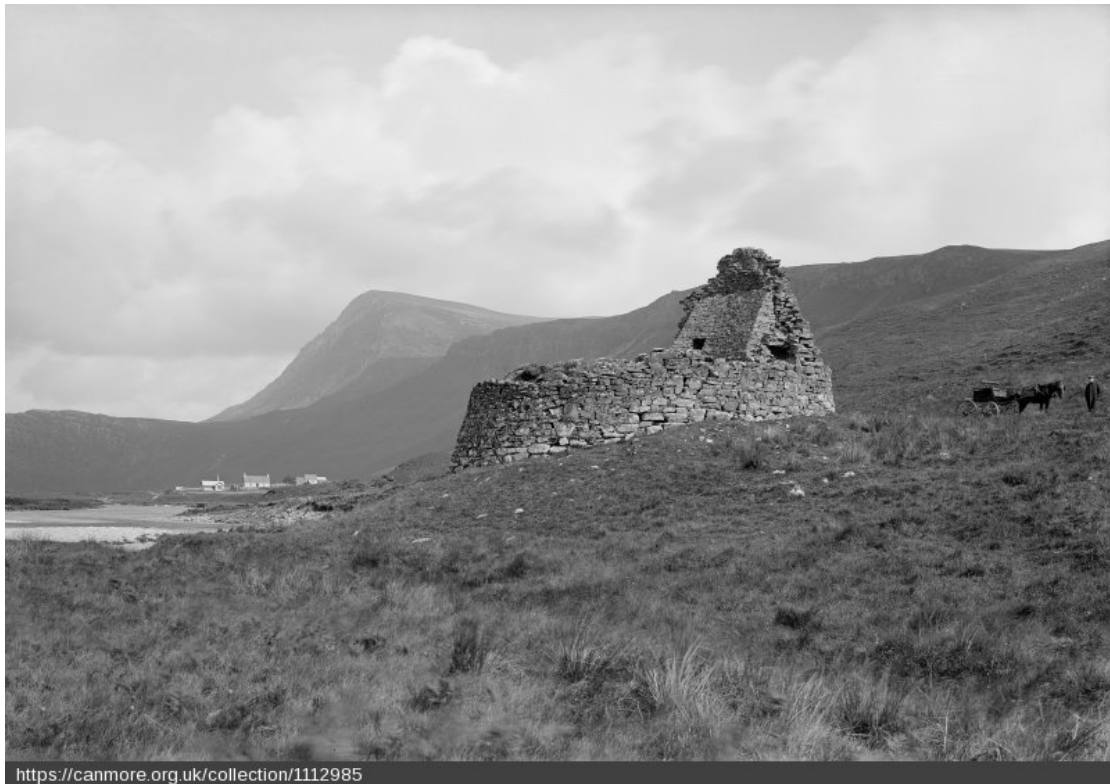
1899 photo by Erskine Beveridge showing buttress already in place (note gap in buttress to allow access to wall gallery – this was later closed up).
