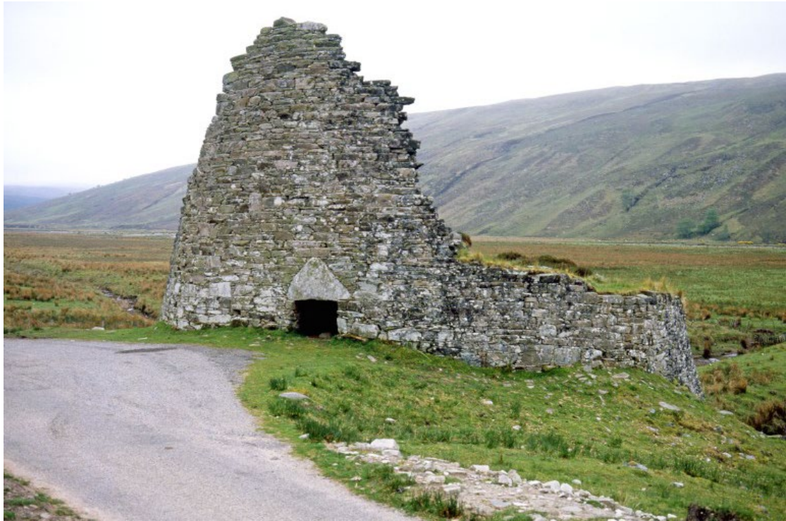
View from roadside.
