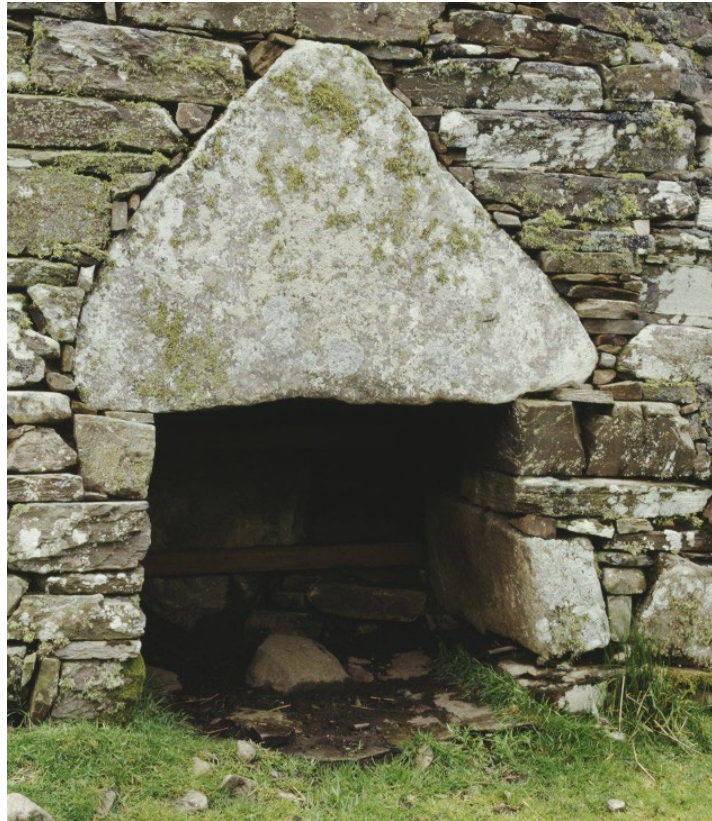
Detail of lintel and blocked entrance.
