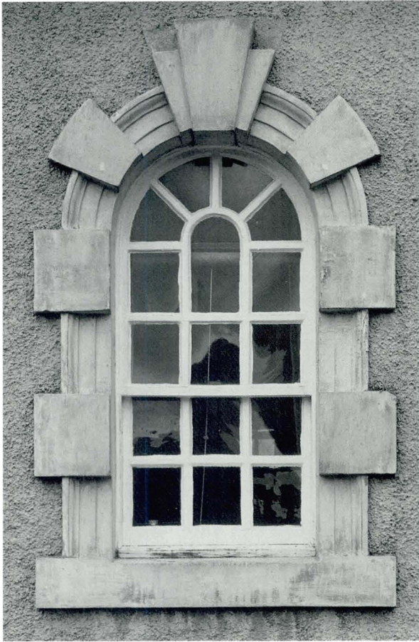
17 Ardmaddy Castle, Argyll, illustrates the character of the Palladian sash window framed by block-and-start dressed quoin stones.
