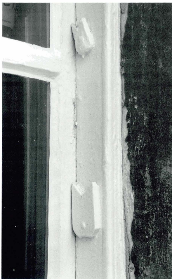
7 Example of early quadrant sash stays, Traquair House.
