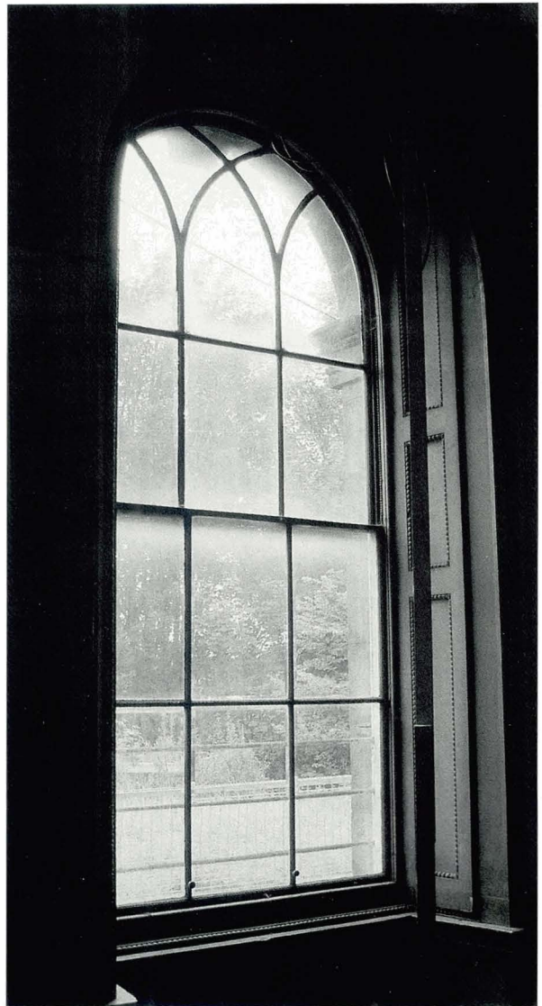
26 and 27 Two phases of work at Newhailes near Musselburgh illustrate the difference between early and late eighteenth century work. The heavy Palladian glazing of the 1720s library contrasts with the State Bedroom (fitted out in the late eighteenth century) which has very fine metal glazing bars and bevelled Vauxhall plate glass.
