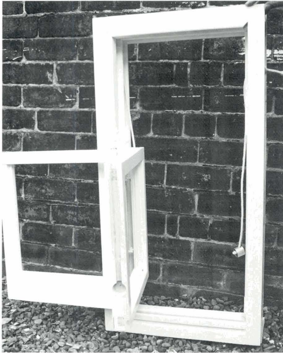
58 A demonstration of the provision of hinges that can allow an upper sash to open inwards for cleaning. The lower sash is rotated on a hinged baton rod. The upper sash is then located onto hinge pins folding out from the pulley stile. A section of the parting bead is made removable so that the sash can swing inwards.
