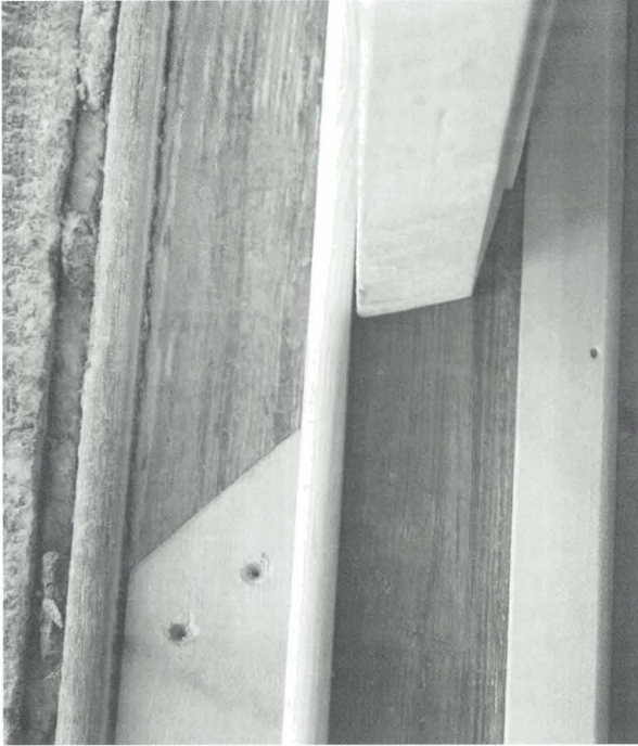
49 Renewing defective parting beads and baton rods.
