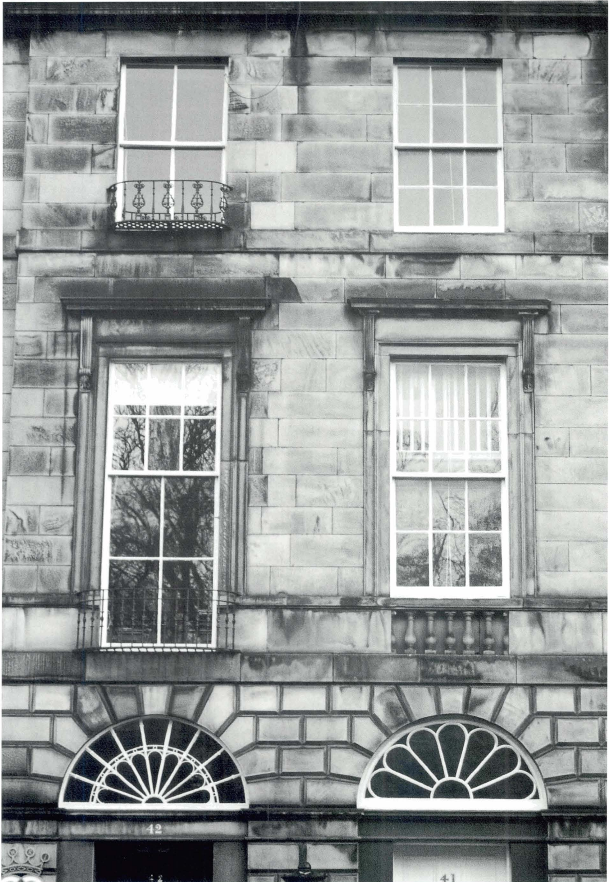
3 The variety in proportions of window openings and their effect on a classical facade. Heriot Row, Edinburgh.
