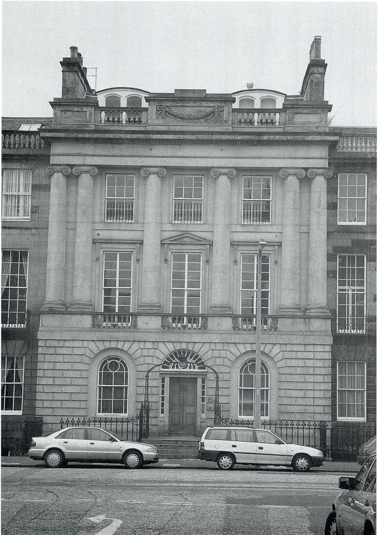
33 No. 23, Melville Street, Edinburgh (designed in 1814 by Robert Brown, but not built until the mid-1820s) is a showcase of all these fashionable variations of sash pattern.
