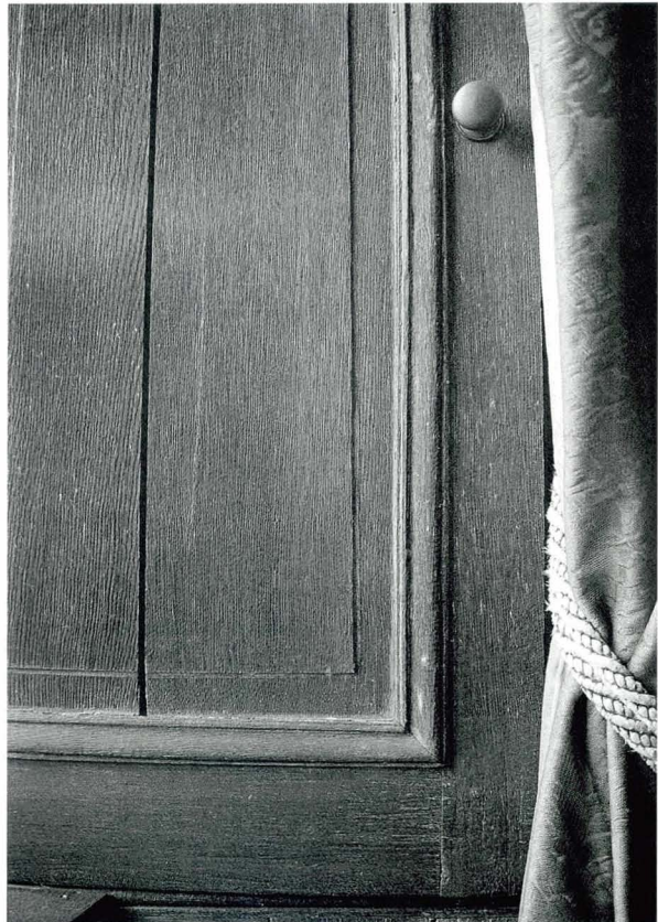
9 Shutter panel mouldings: bolection in conjunction with raised and fielded, on a shutter of the 1690s.
