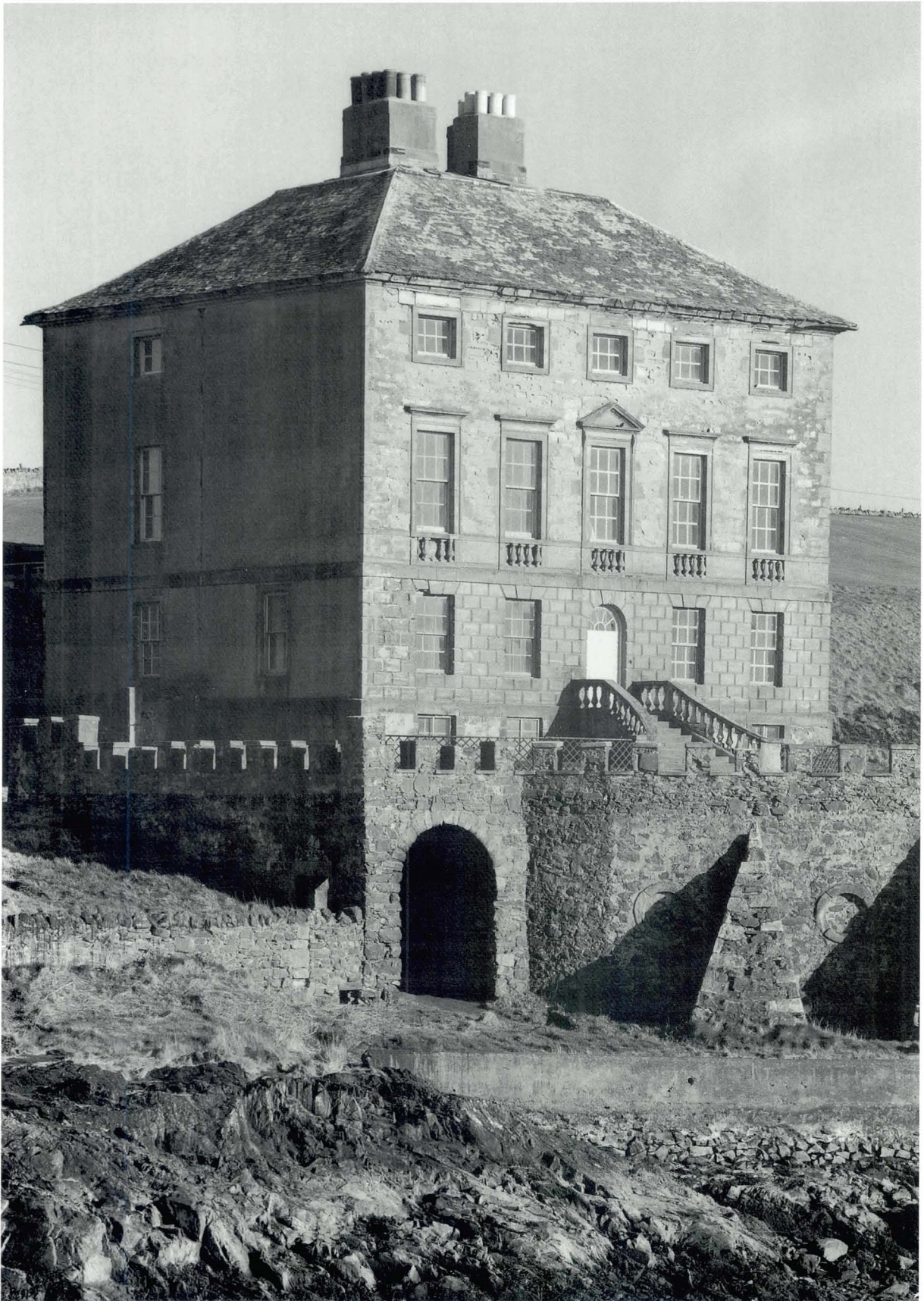
29 Small windows of just one sash (made to slide upwards into a cavity in the masonry above the opening) are found in the attic storey of Gunsreen, Eyemouth, c.1754, attributed to John Adam.
