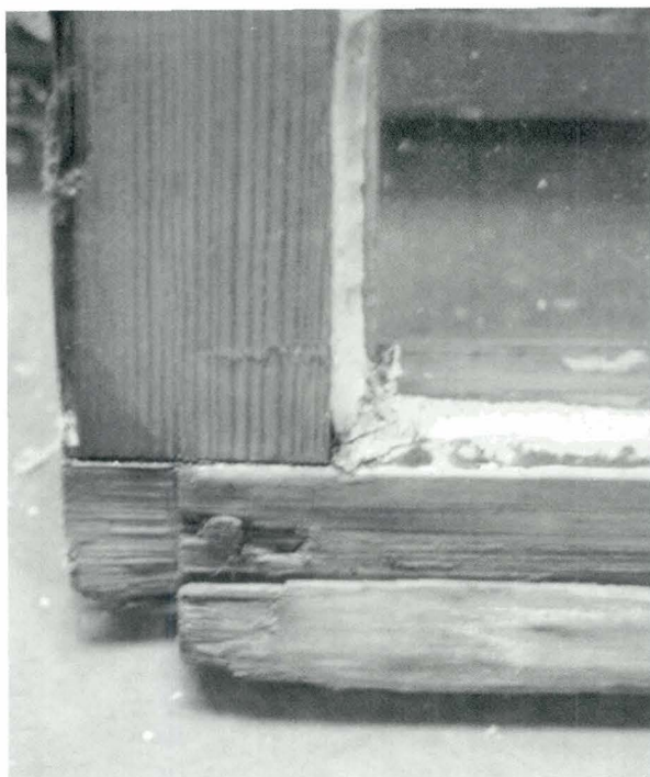
47 The careful repair of decayed timber (before)
