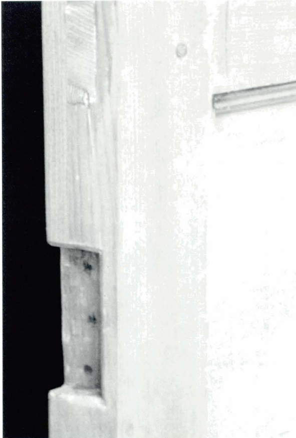
51 Shutter repair, replacing damaged timber at hinge fixing positions.
