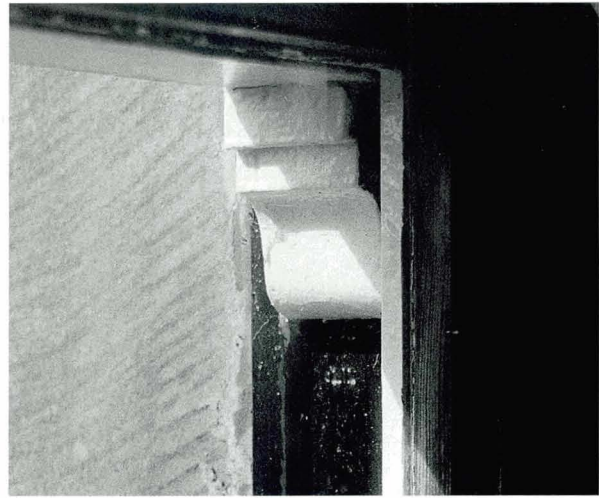
42 Moulded sash horns of the late C19.
