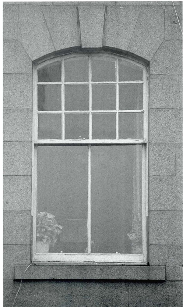
35 Mixed pane sizes in a building of 1899, Aberdeen.
