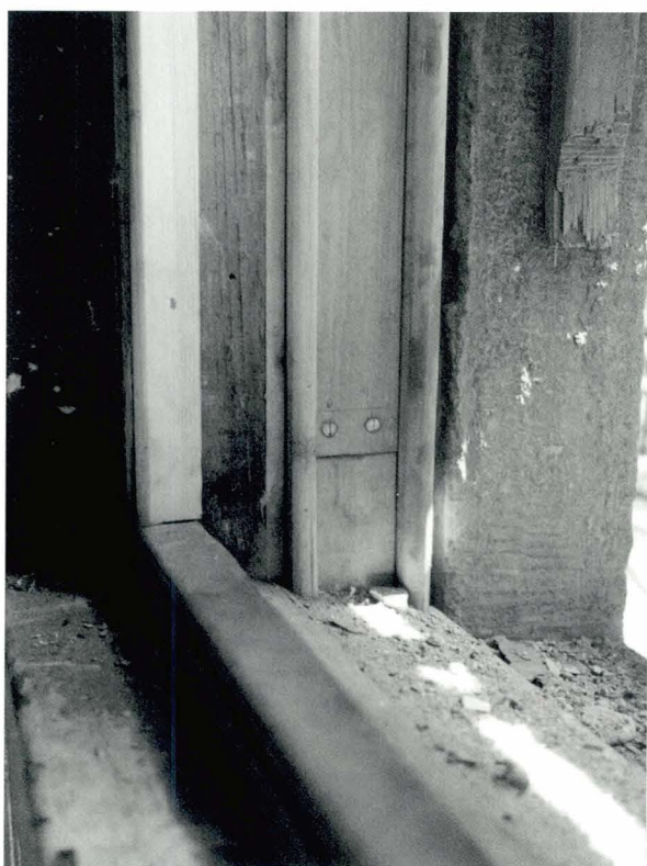
73 New weight cover fitted.
