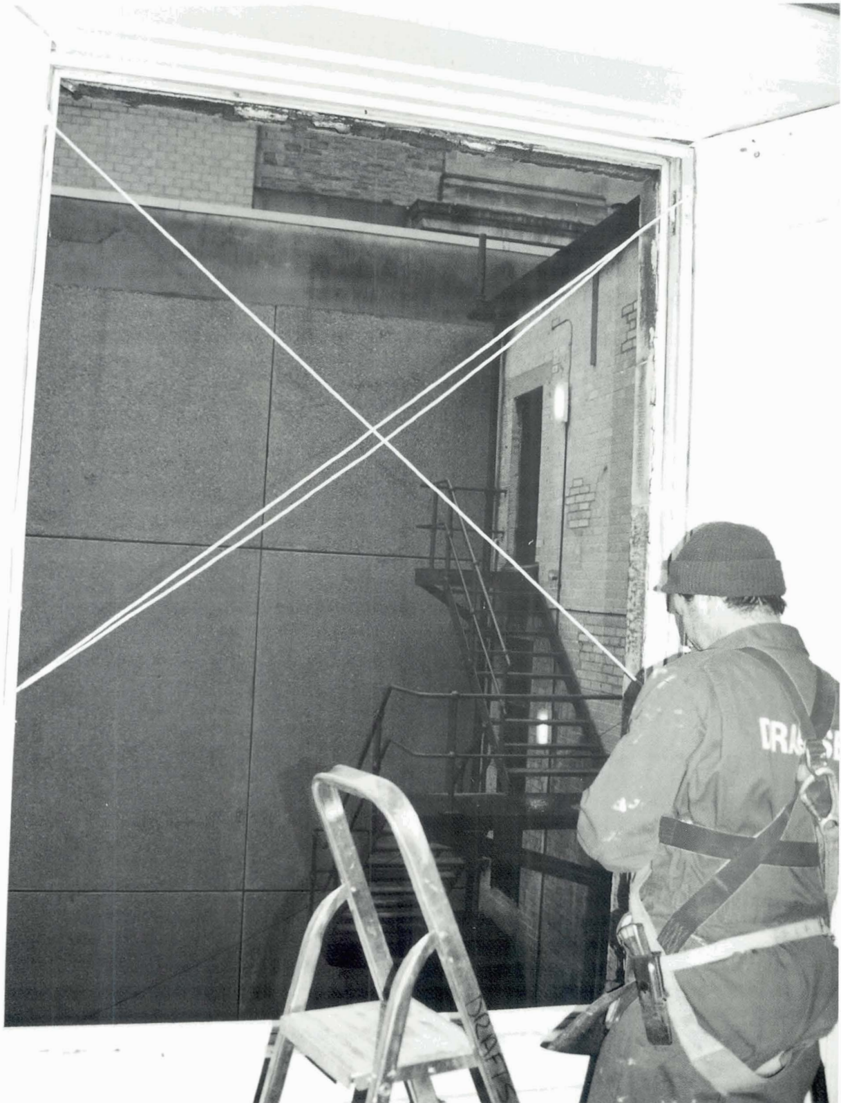
85 Re-cording a sash and case window.
