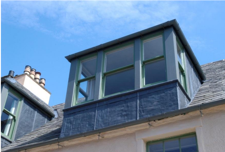
Fig. 17: Front dormer (street facing) with new lead cladding
