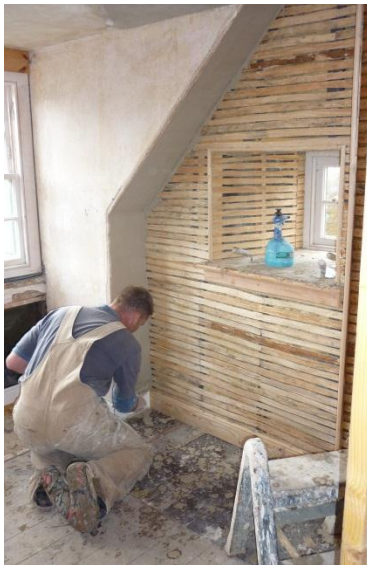
Fig. 30: Application of lime plaster to timber lath
