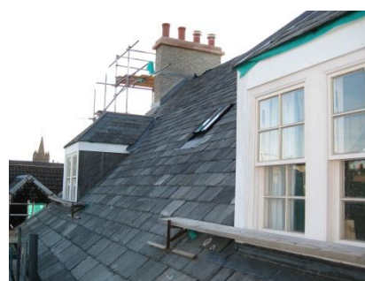
Fig. 8: Reslatted roof - rear view of property
