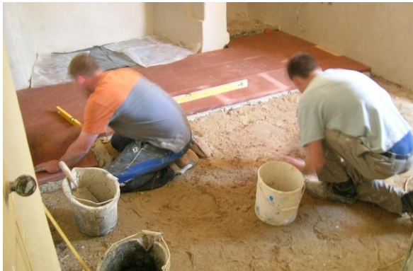
Fig. 26: Sandstone floor laid on aggregate and sand foundation
