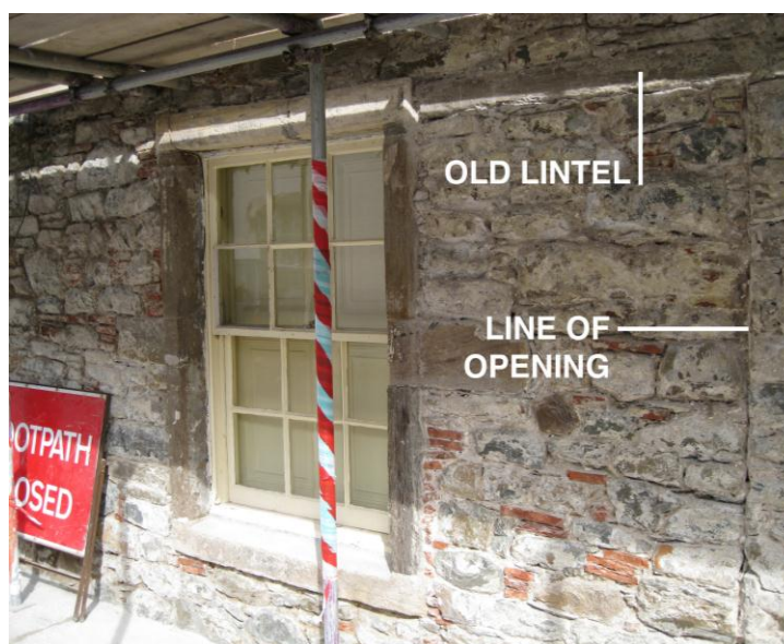
Fig. 54: Remnants of old shop door on front elevation
