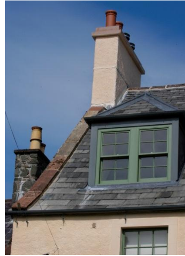
Fig. 18: Rear dormer with lead flashing and cladding
