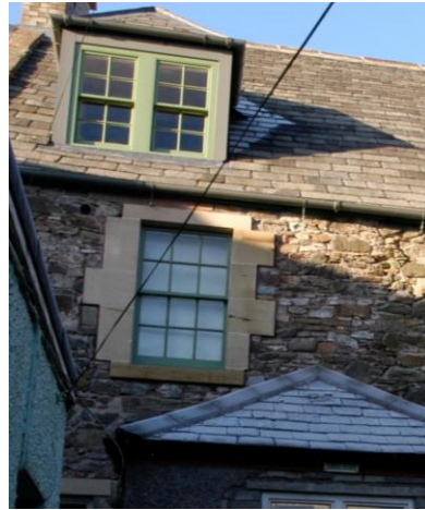
Fig 39: The new stone surround for the window
