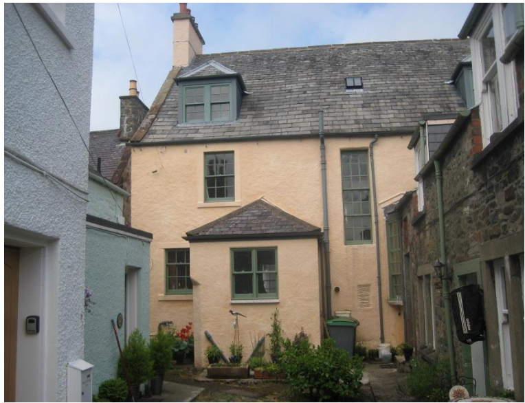
Fig. 20: The rear elevation after new windows had been installed
