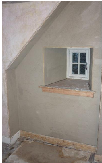
Fig. 31: Lime plaster with timber beading
