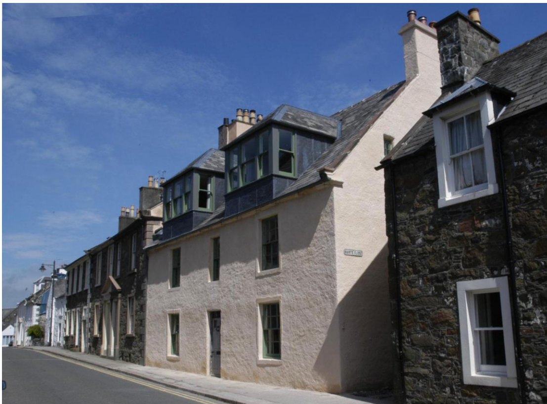
Fig. 41: The completed works - 2010
