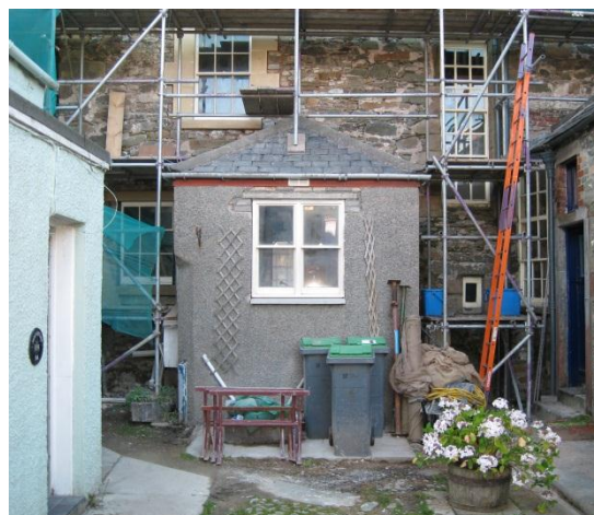
Fig. 56: Utility addition to rear of property. Built in circa. 1970.
