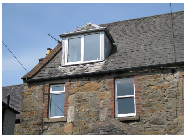
Fig. 55: Dormer on the rear of the property. There are two dormers to the rear of similar size. Both were added circa. 1937.
