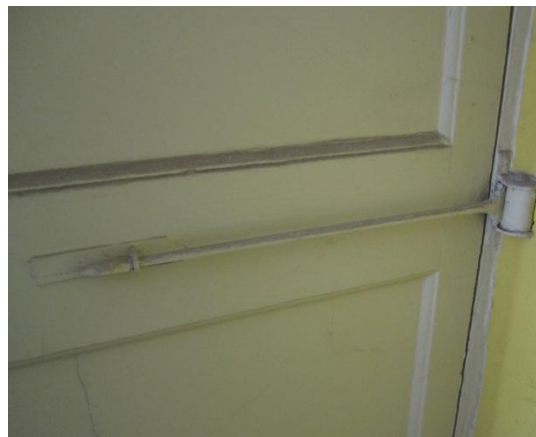
Fig. 34: Existing ironmongery - door closer
