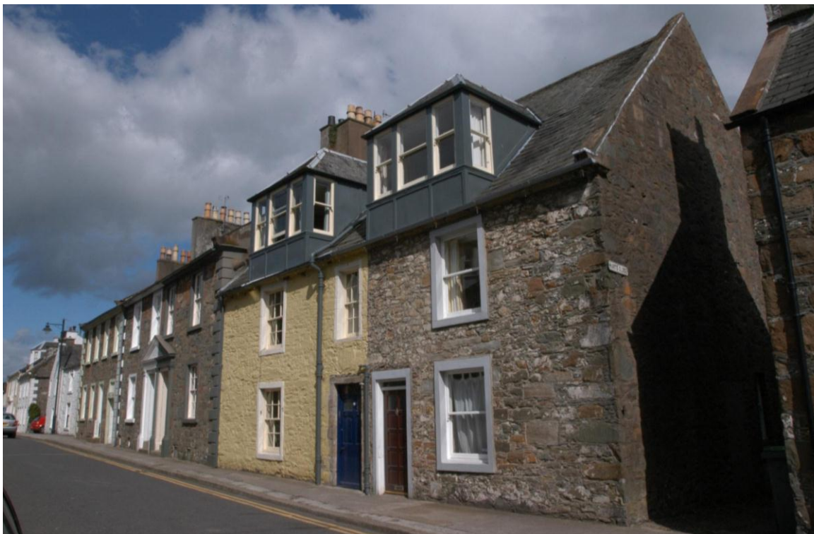
Fig. 1: No. 27 (left) and No. 29 (right) High Street, Kirkcudbright prior to works
