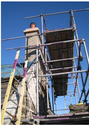
Fig. 12: Construction of south gable chimney stack
