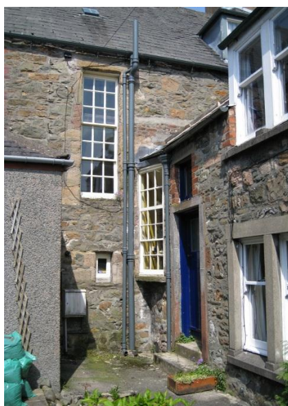
Fig. 53: Boot room addition to the rear of the house to the right. The later utility room extension is visible on the left.
