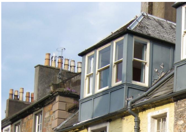
Fig. 15: Front dormer prior to upgrade and improvement works
