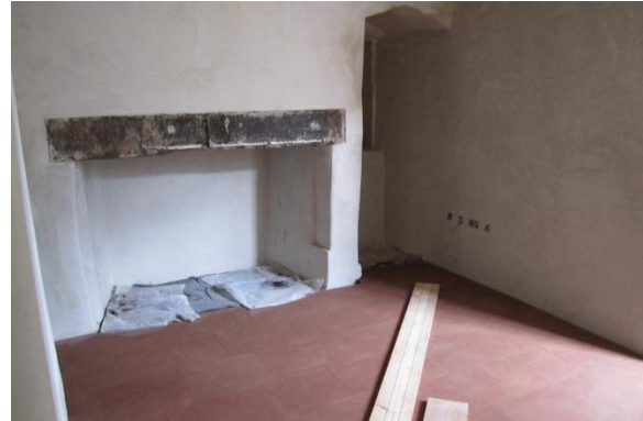
Fig. 27: Sandstone floor laid without mortar joints
