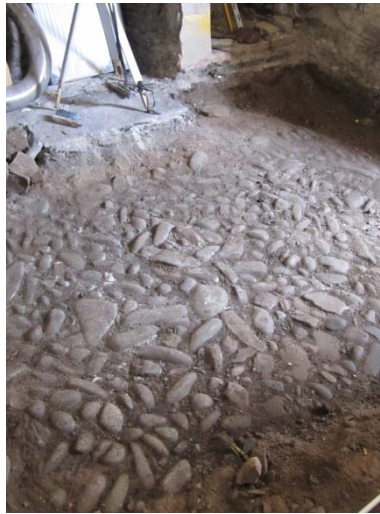
Fig. 3: Cobbled floor excavated in snug
