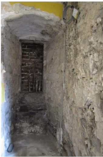
Fig. 2: Arched lintel and roll mouldings on window margin beyond.
