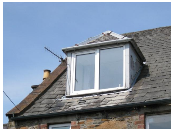
Fig. 16: Rear dormer prior to upgrade and improvement work
