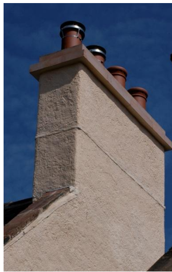
Fig. 13: Reinstated lime harled chimney stack
