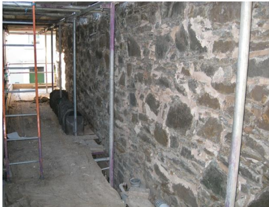
Fig. 9: Repointing work to the external walls
