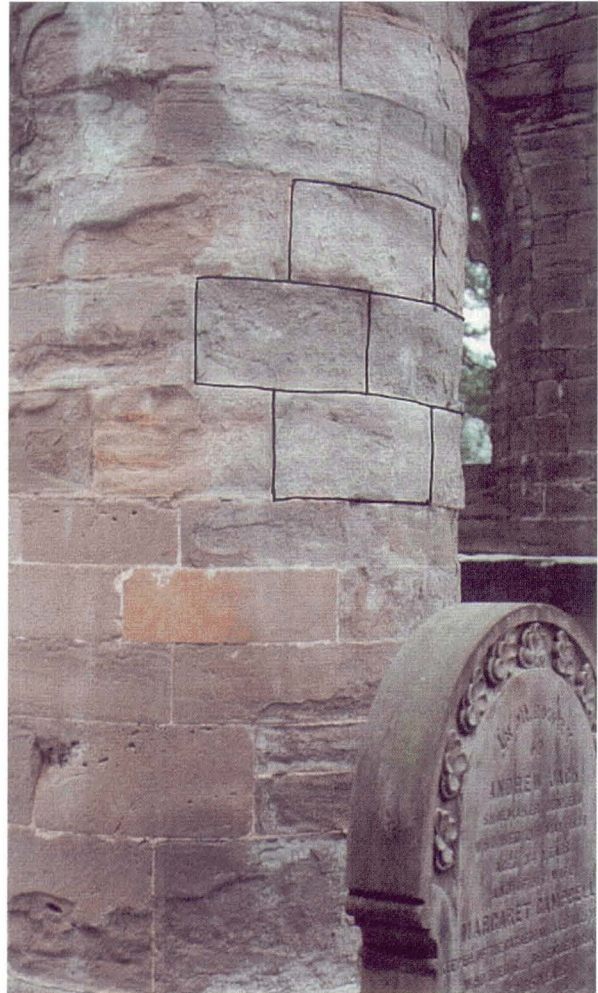
Figure 64 Treated area on column at Dunkeld Cathedral.
