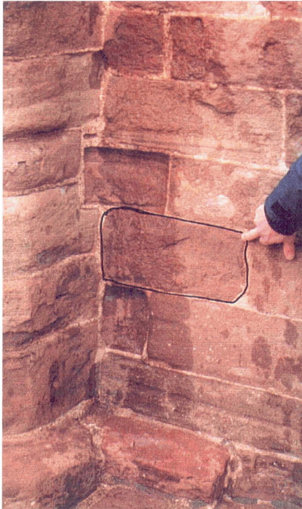
Figure 63 Sandstone block from Arbroath Abbey cored during this research project.
