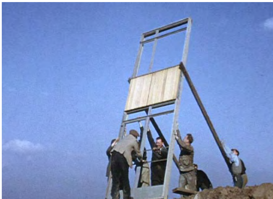
4 Unskilled workers from the Dunedin Self-Build Association in action erecting a window panel. Taken from the 16mm silent, colour film We Build Houses , 1953, directed by John L Paterson. Courtesy of Scottish Screen Archive at National Library of Scotland, ref 6378
