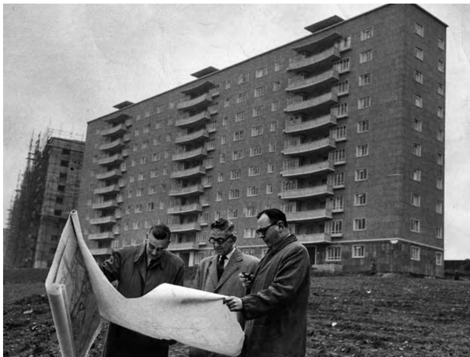
7 Councillor Duncan discussing details of the Glasgow apartment block 'Moss Heights' with T Barclay and G Campbell, 1953 © Getty Images
