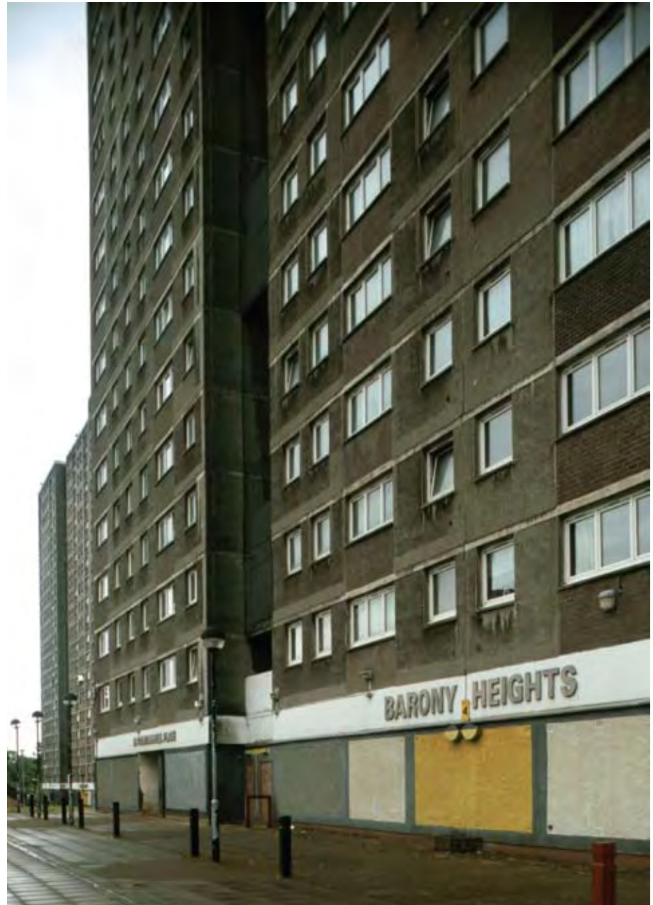
2 20-storey Crudens slab blocks at Sighthill, Glasgow, built 1963-8: the blocks in this view were blown up in 2009. © M Glendinning
