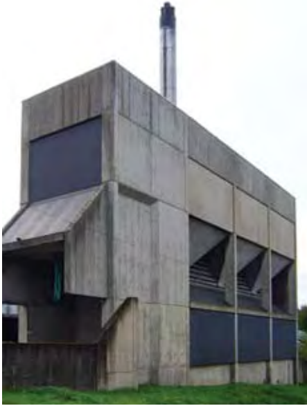
8 Dingleton Hospital former Boiler House, Melrose, by Peter Womersley, 1977.
