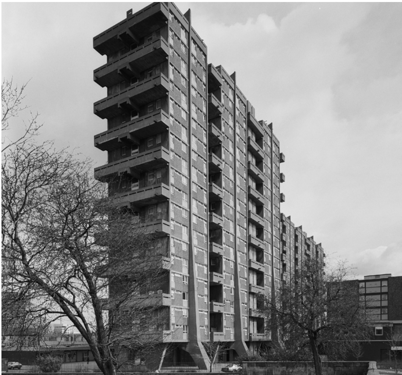
10 View from west of Area 'C' of Hutchesontown-Gorbals Comprehensive Development Area (CDA), Glasgow (built 1962, photo 1987)
