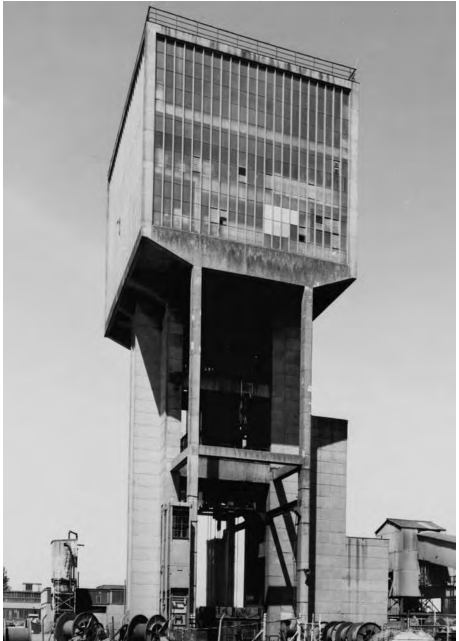
2 Monktonhall Colliery, Fife (No 1 shaft winding tower), prior to demolition in 1989.
