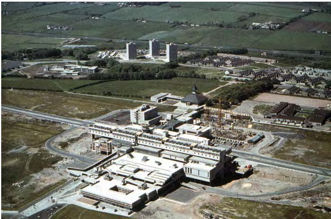
3 1967 view of Cumbernauld New Town under construction: Town Centre Phases 1 and 2 at centre and Ravenswood and Seafar housing areas in background. © Cumbernauld Development Corporation
