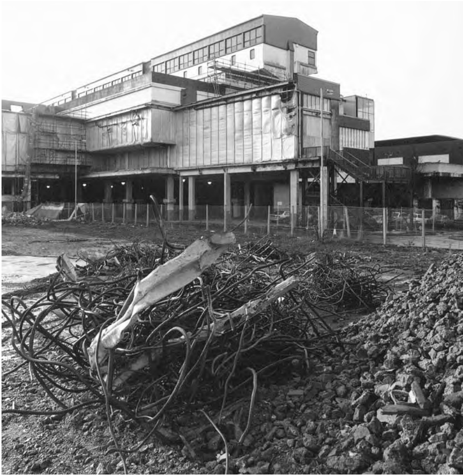
4 Cumbernauld Town Centre, during part demolition in 2000.
