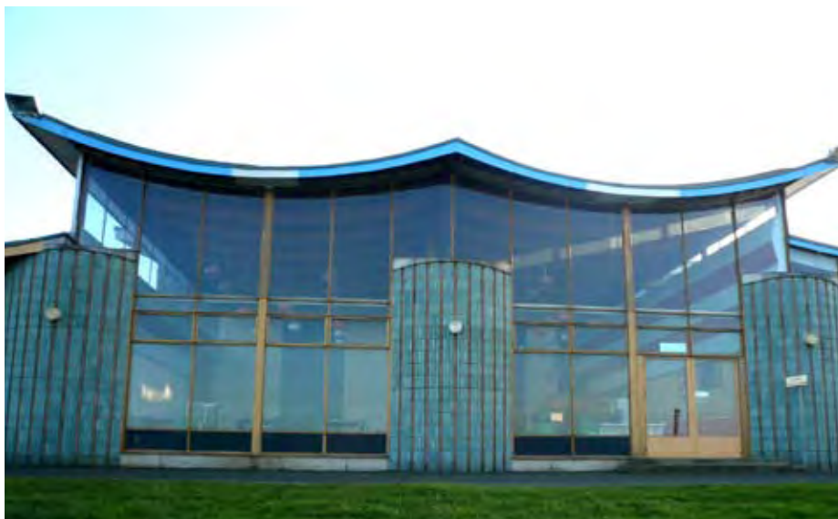
3 Madras College, Kilrymont Building, St Andrews, Ian Stewart with R S Lawrie and Fife County Council Architects, opened 1967.
