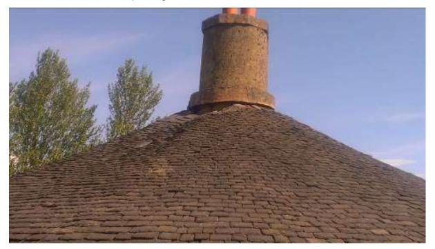
Figure 2. Water ingress through the chimney and the skew junction had resulted in the rotting and settlement of rafters, seen here middle left.
