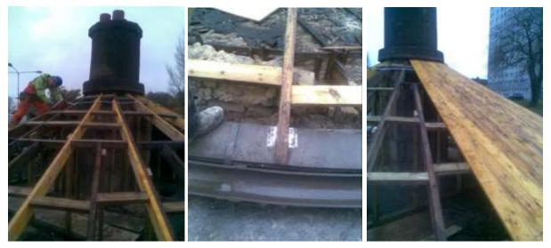
Figure 8. Repairing roof timbers; original rafters were retained where in good condition with a number of complete and partial replacements used. Additional lateral bracing was also introduced.
