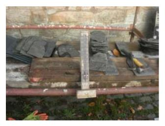
Figure 5. A simple gauge was used to sort slates which had been removed from the roof into sizes for use in re-slating.
