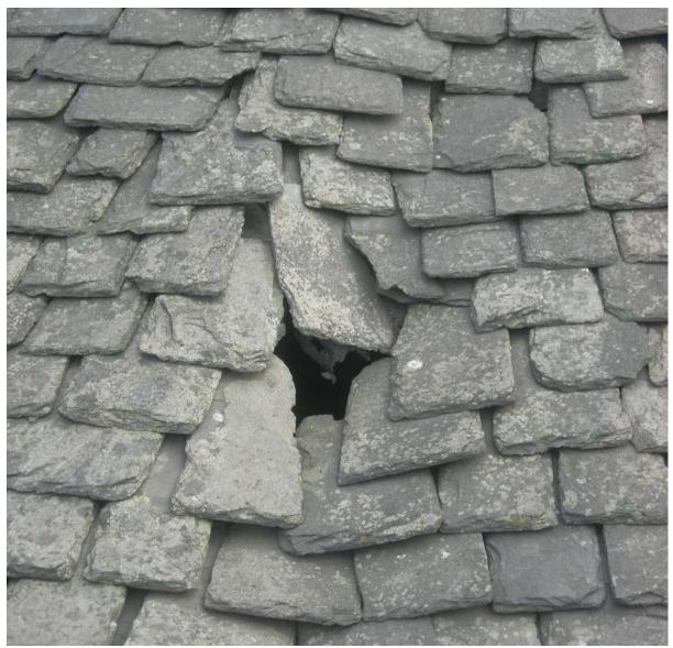
Figure 3. Missing slates and damaged sarking were some of the defects identified.
