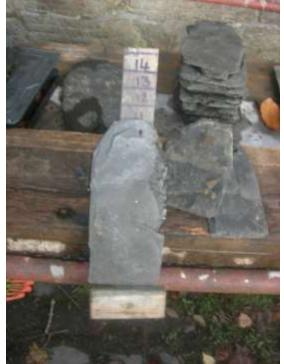
Figure 6. Using the slate gauge to grade slates for size prior to re-use.
