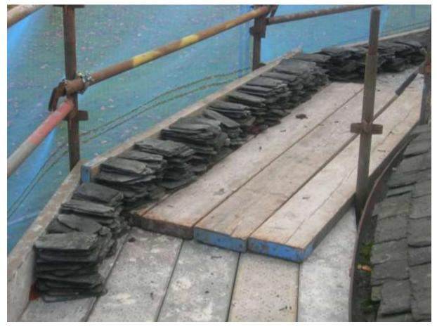
Figure 7. The sized slates laid out on the scaffold ready for re-laying.
