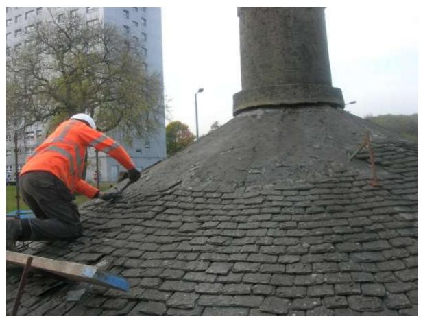
Figure 4. The removal of slates at the Round Toll was undertaken with care in order to maximise the amount of slate which could be re-used.
