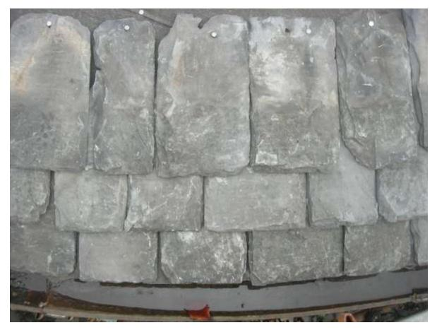
Figure 11. The first three courses of slate re-laid at the Round Toll using the largest slates at the eaves course, using a single nail at the head, as is traditional practice.
