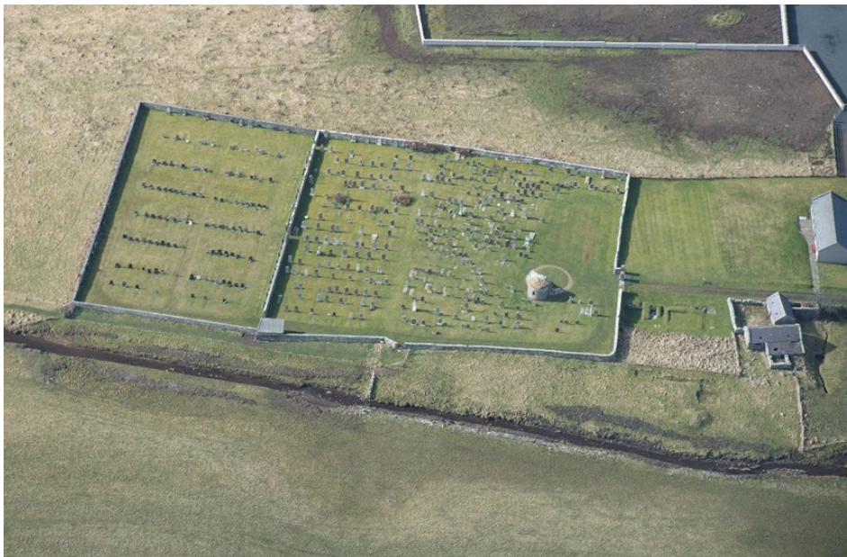
Figure 6: Aerial photograph of site. © HES.
