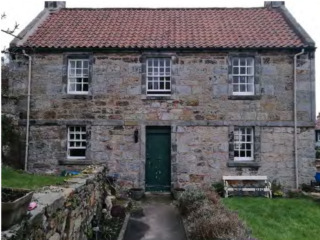
Figure 1: Domestic buildings such as Wee Causeway, described in Refurbishment Case Study 3, were included in the project review.
