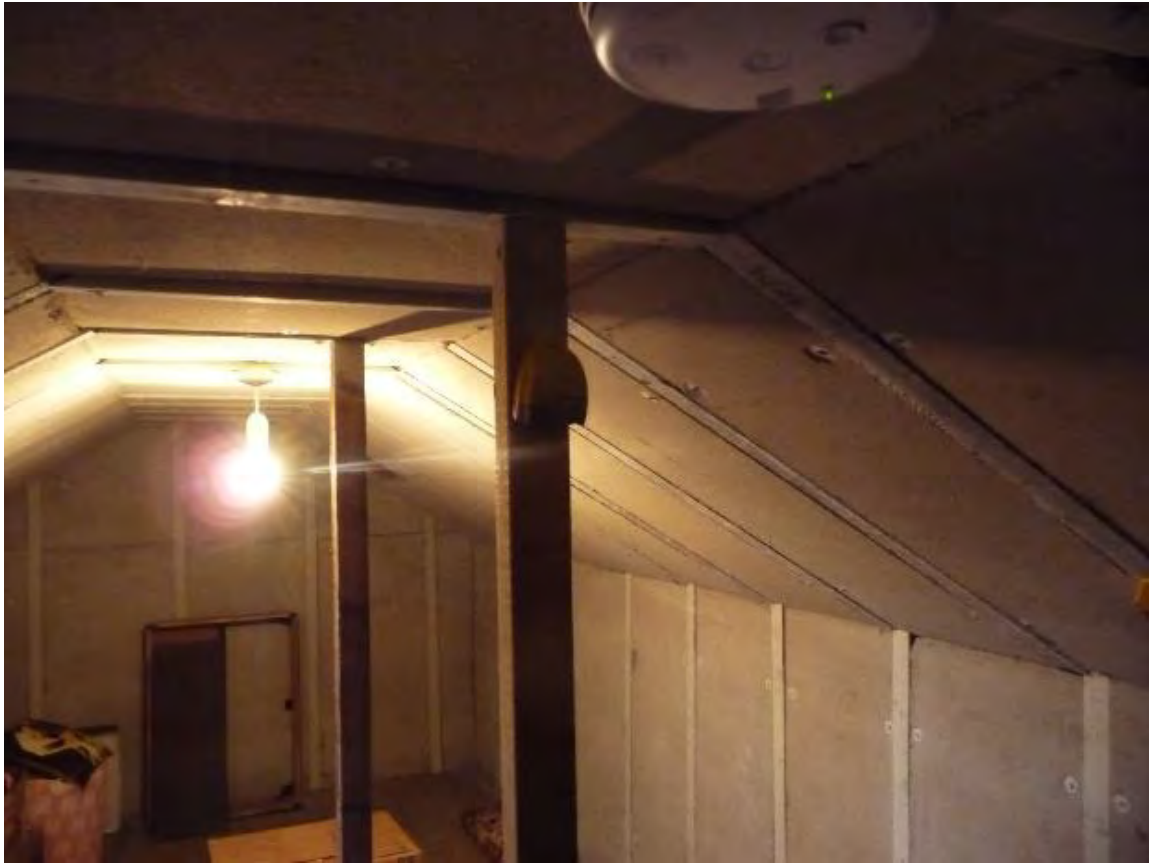
Figure 11: Wood fibre board insulation creating a warm roof at Annat Road.
