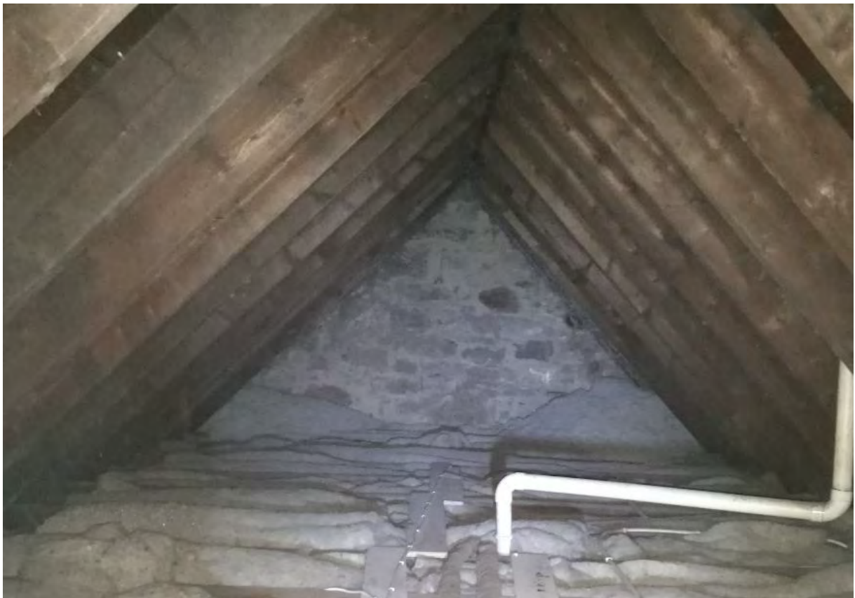
Figure 7: Blown cellulose insulation deposited in the attic space at Wells o' Wearie.
