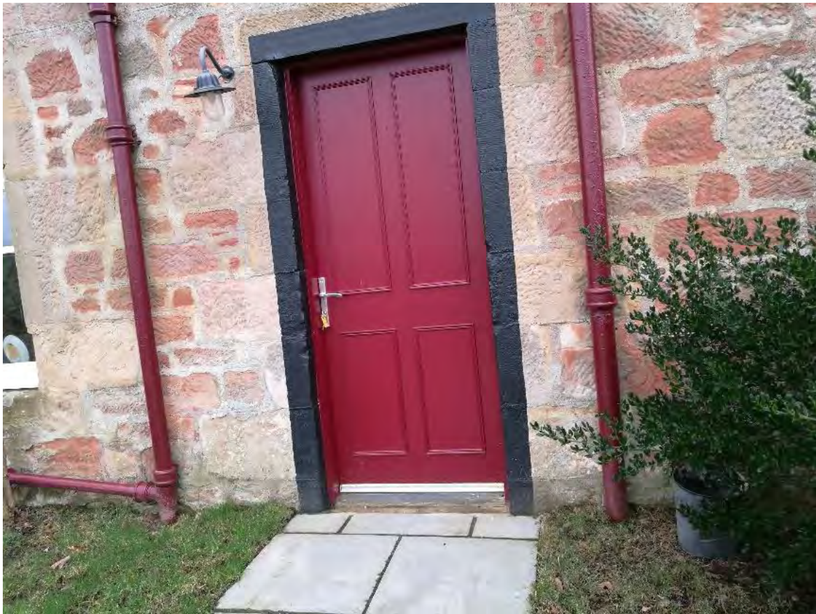
Figure 25: The new front door for the Garden Bothy, insulated with aerogel.
