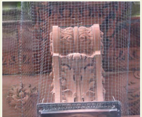
Fig. 4: In this case, the netting completely surrounds the carvings making it quite difficult to see the detail.
