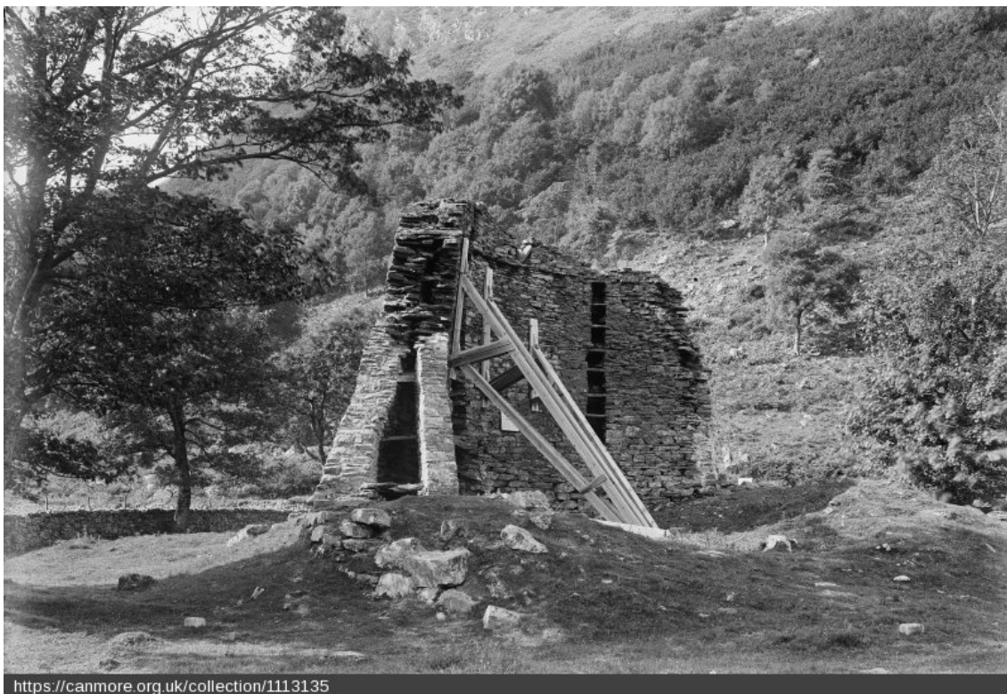
Photo taken by Erskine Beveridge c. 1897, showing timber props and cement patching of wall-ends
