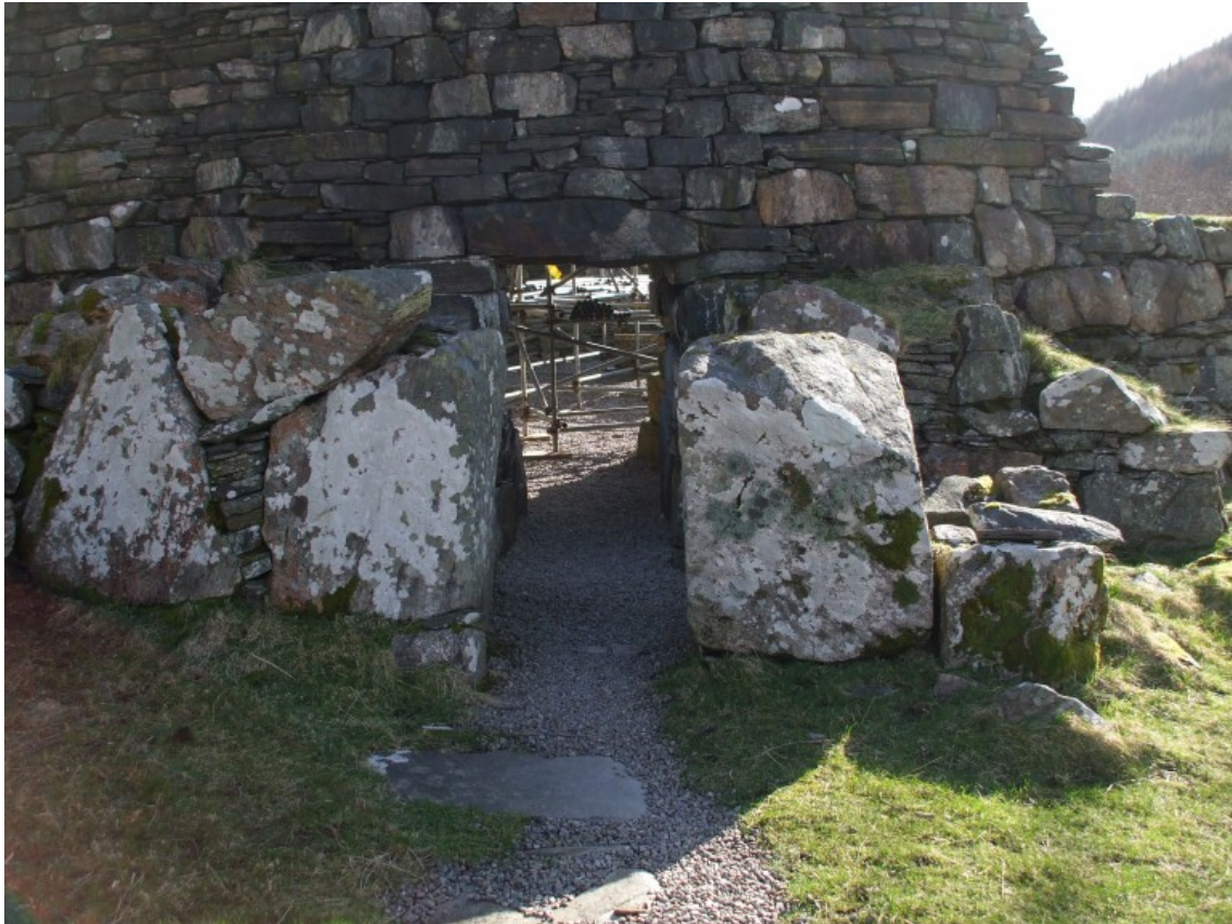
Entrance from outside, showing lintel and massive stones of added outer structure
