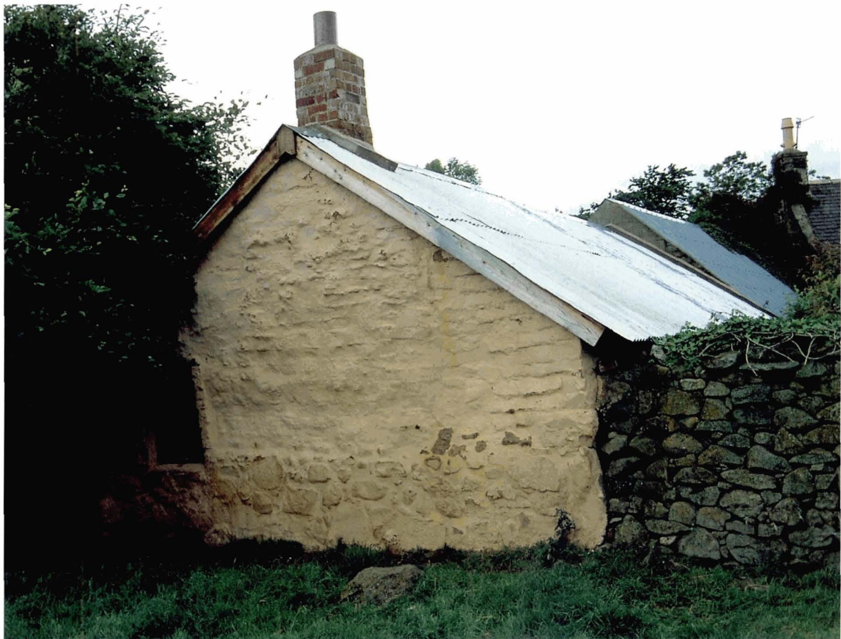
fig 58. Completed gable, Corse Croft. © Bruce Walker.
