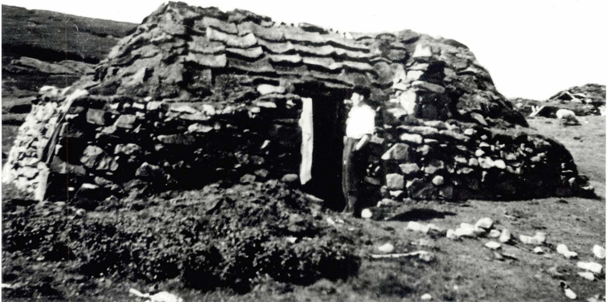
fig 24b. Divet roof to sheiling hut. © NMS.
