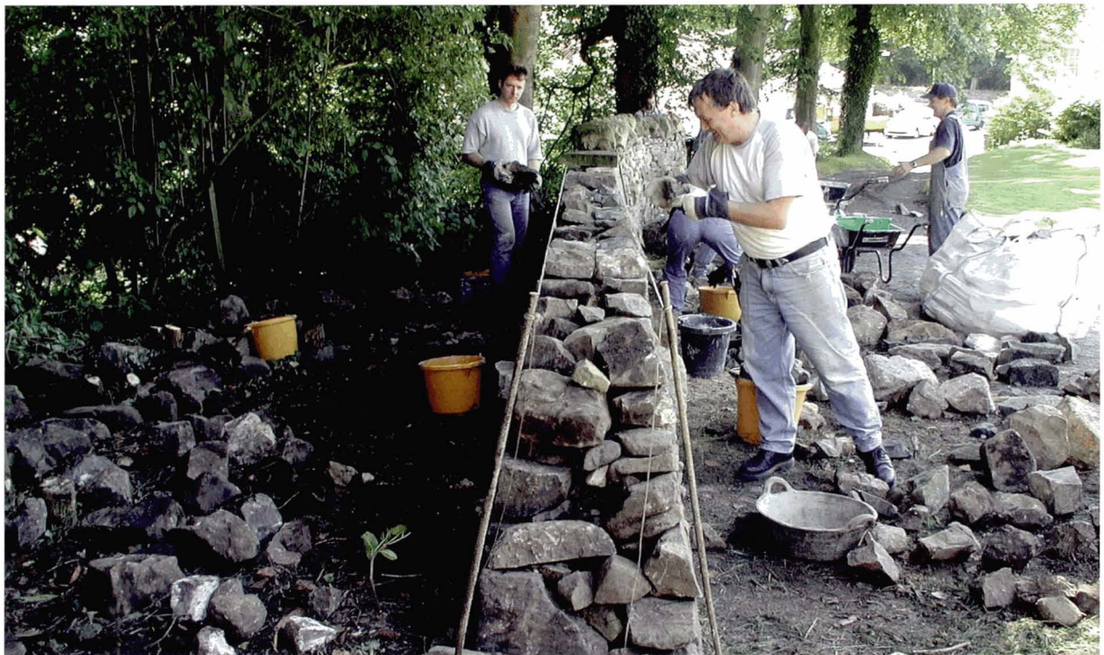
fig 52. Rough profile frame used here in dry-stone walling © Scottish Lime Centre.
