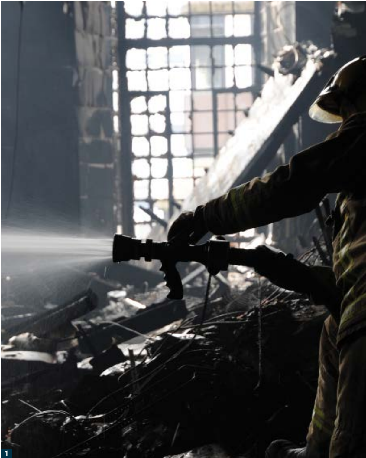
Figure 1. Fire is one of the most devastating incidents which could affect a historic building. This image shows a firefighter during the aftermath of the 2014 fire at Glasgow School of Art.
