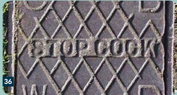
Figure 36. Close up of a stop cock cover.
