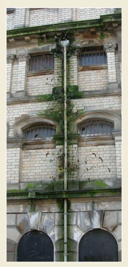
Fig. 2: Water ingress from sources such as blocked gutters or downpipes is a major cause of deterioration of brickwork.
