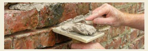
Fig. 10: Joints should be well raked out and dampened before repointing work takes place.
