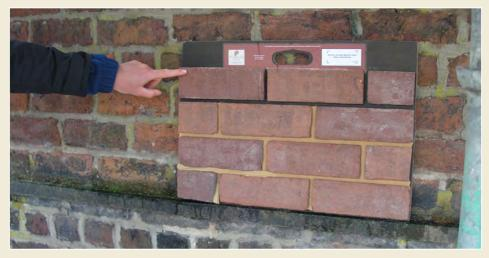
Fig. 7: Replacement bricks should match those in-situ as closely as possible; samples of bricks should be checked to gauge their suitability prior to a repair project.
