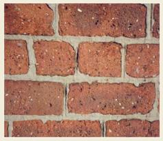
Fig. 9: Brick after cleaning showing the potential damaging effects of abrasive cleaning methods. Note the loss of the protective external surface making the bricks more prone to decay.
