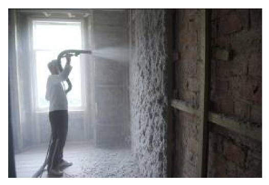
Fig. 4. Blown cellulose material sprayed damp directly onto masonry
