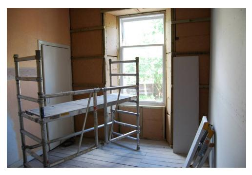
Fig. 6. Hemp board insulation applied between timber framing
