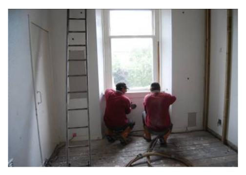
Fig. 3. Blowing bonded polystyrene bead behind existing wall lining
