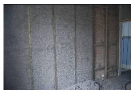
Fig. 5. Cellulose fibre trimmed finished flush prior to sheeting with plasterboard
