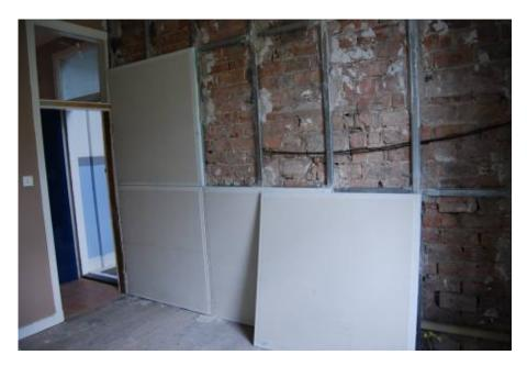
Fig. 7. Aerogel insulated board being applied to mass masonry on metal straps
