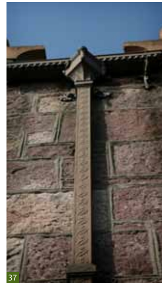
Fig 37 Cast iron rainwater goods were often highly decorated.
