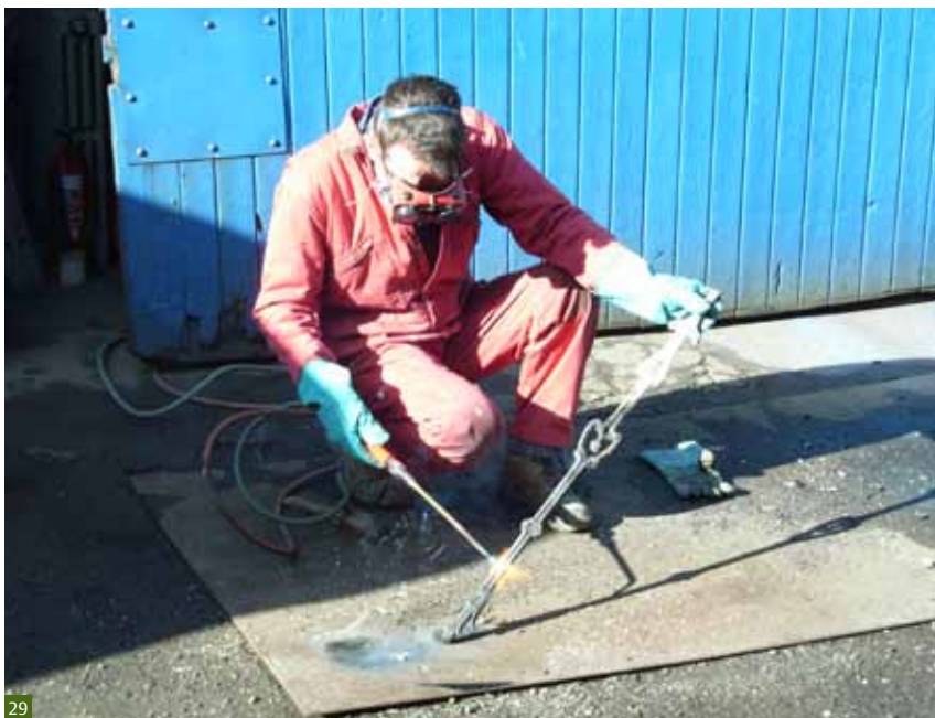
Fig 29 Flame cleaning ironwork using an oxyacetylene torch.
