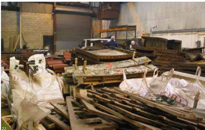
Fig 22 This workshop is not large enough to store a dismantled iron structure of this size without serious risk of damage. The iron components have also not been stacked securely. If ironwork is to be removed to a workshop, ensure that the contractor has suitable premises to store the ironwork and carry out works.
