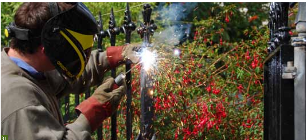
Fig 31 Welding ironwork in-situ.
