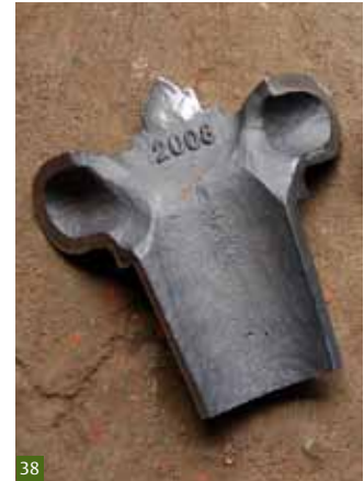
Fig 38 New castings should be marked with the year of manufacture to distinguish them from original castings.
