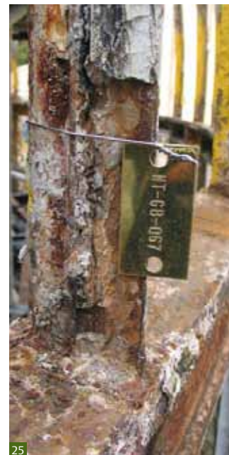
Fig 24 Metal tags can be numbered according to a record drawing and attached to the ironwork as it is dismantled.
