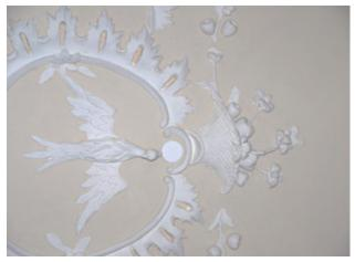
Fig. 7 Circular concealed sprinkler head beside the bird's beak on a decorative plaster ceiling.
