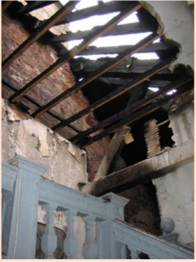
Fig. 4 Faulty wiring was the possible cause of fire in this sub-divided townhouse.
