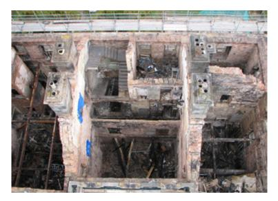
Fig. 2 Fire damage to a property during conversion works.
