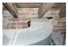
Fig. 5 Breaches such as this hole in a brick masonry wall can facilitate fire and smoke spread.
