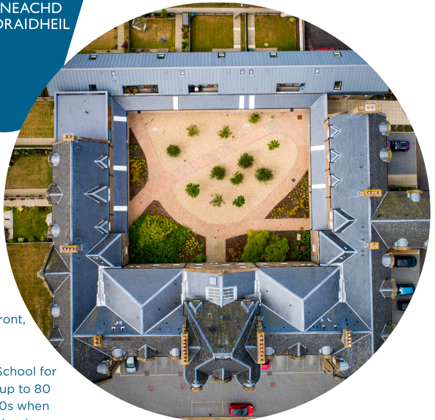
Top view of Parkview school with redeveloped courtyard and mews properties. © Whiteburn
