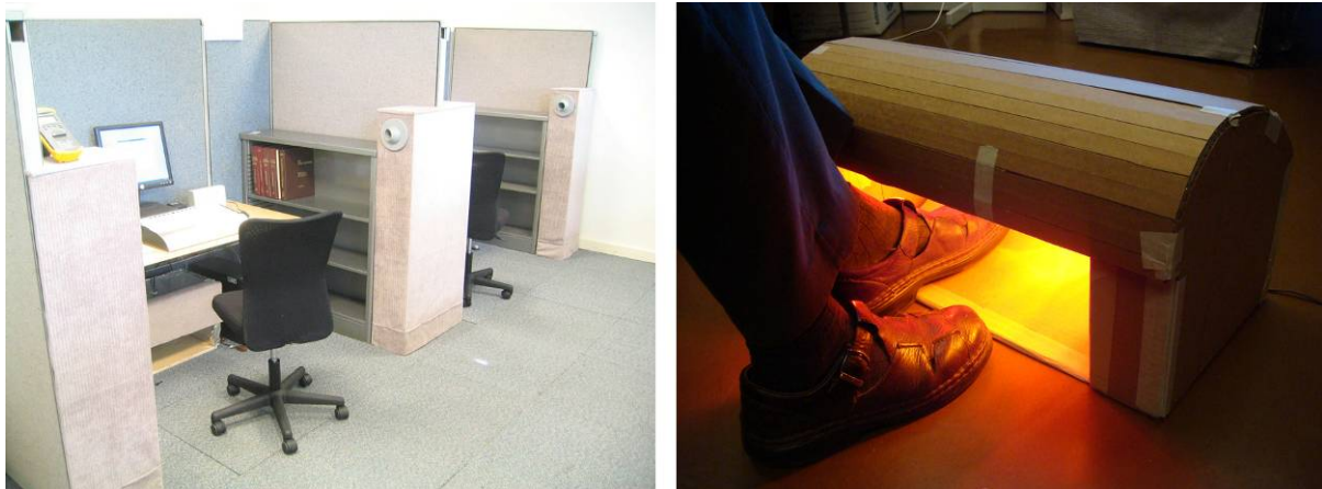
Figure 7 Radiant foot warmers, now being experimented with in the USA, could avoid the need to heat the room for certain periods of the year. (Photo © E. Arens)
