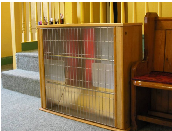
Figure 5 The prototype Heatbox Radiant Stove (dual control with 2×1 kW) installed in the community room of a church (Photo © M. Humphreys)
