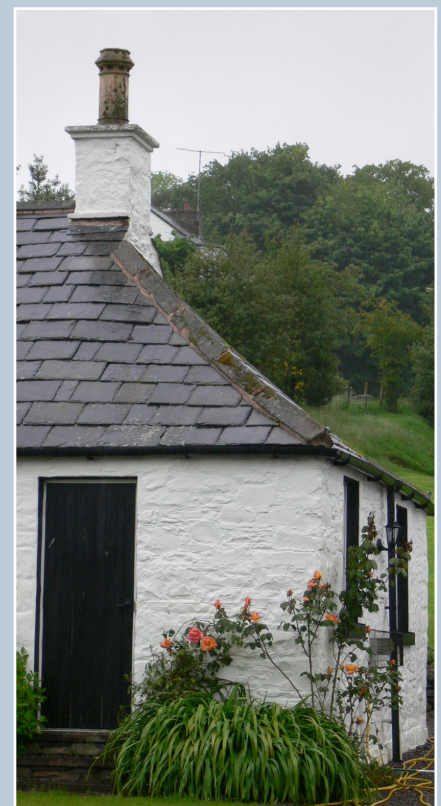
Regular courses, but random widths of local slate fixed using a double-lap method under stone ridge pieces. Dumfries & Galloway.
