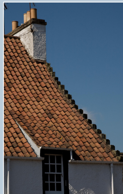
Clay pantiles and a 'catslide' dormer on a 17th-century house, Falkland, Fife. The roof sweeps up a little towards the eaves. © N. Haynes.
