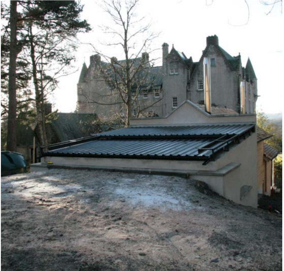
Fuel store for a biomass boiler serving category B listed Kincardine Castle, Aberdeenshire. This small storage facility is refilled from a larger shed located further away. This storage shed has been built discreetly behind a timber dog kennel.
