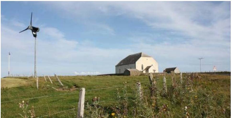
Category C listed Westray Parish Church in Orkney became self-sufficient in energy with a 6kW wind turbine, ground-source heat pump and back-up diesel generator. The turbine is far enough (80m) from the building to avoid turbulence. © Ease Archaeology
